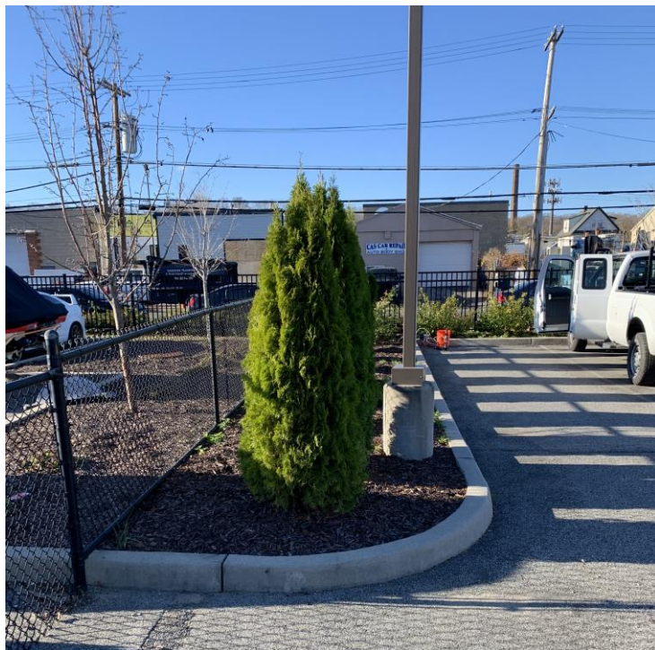
Photograph 2: Curbed lighting areas at 442 Waverly Avenue are in good condition with no evidence of erosion or cracks, looking northwest.
