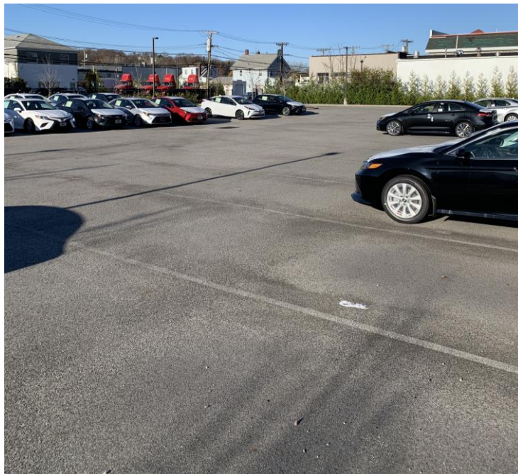
Photograph 4: Onsite asphalt at 442 Waverly Avenue is in good condition with no evidence of penetrations or large cracks, looking north-northwest.
