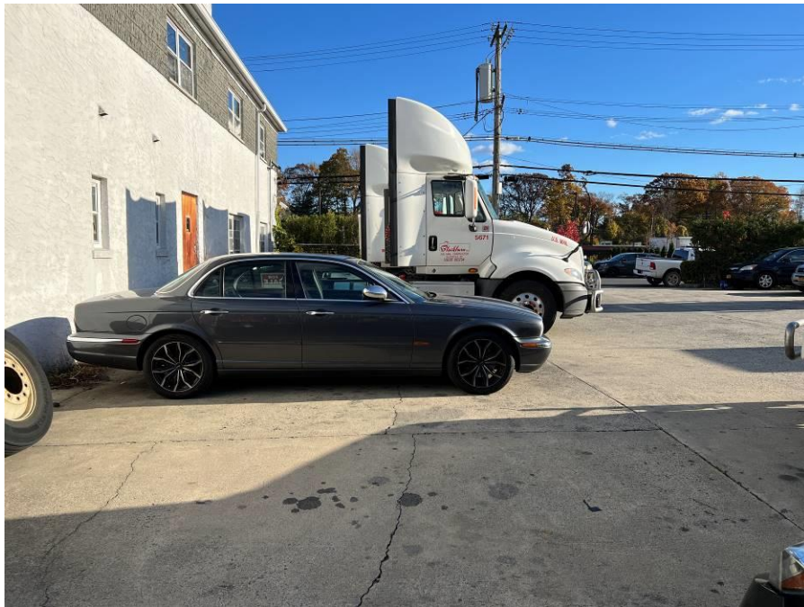
Photograph 1: View of concrete cover system at 441 Waverly Avenue in good condition with some cracks wider than 1/4-inch that should be monitored, looking southeast.
