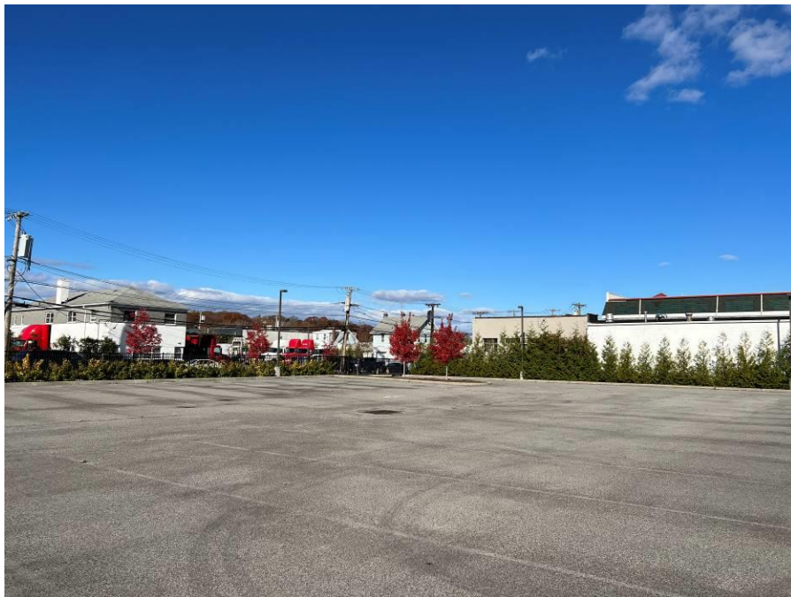
Photograph 4: Onsite asphalt at 442 Waverly Avenue is in good condition with no evidence of penetrations or large cracks, looking north-northwest.
