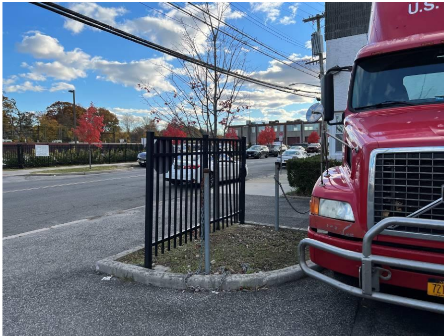
Photograph 3: Curbed areas and asphalt cover system at 441 Waverly Avenue in good condition with no evidence of damage or large cracks, looking south.
