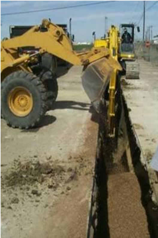
Installation of EHC PRB
