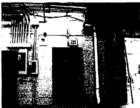
Photo 3 is a view showing a typical valved interior suction point (#4A-B) in Building #4.
