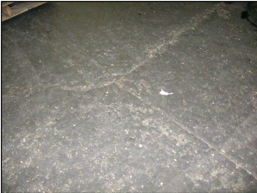
Photo No. 6: Cracks in concrete noted in small press room.
