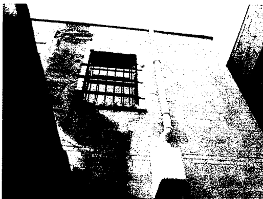
Photo 1 is a typical view of an outside mounted exhaust fan and discharge pipe for system 4B on Building #4.
