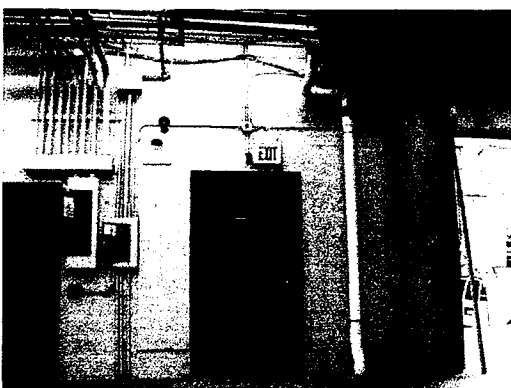
Photo 3 is a view showing a typical valved interior suction point (#4A-B) in Building #4.
