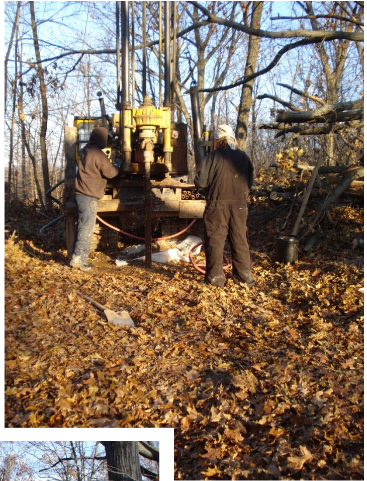
Site Photograph Number 11: Drill cuttings were placed on polyethylene sheeting next to the borehole. Cuttings were placed in the borehole as backfill once boring was completed.
