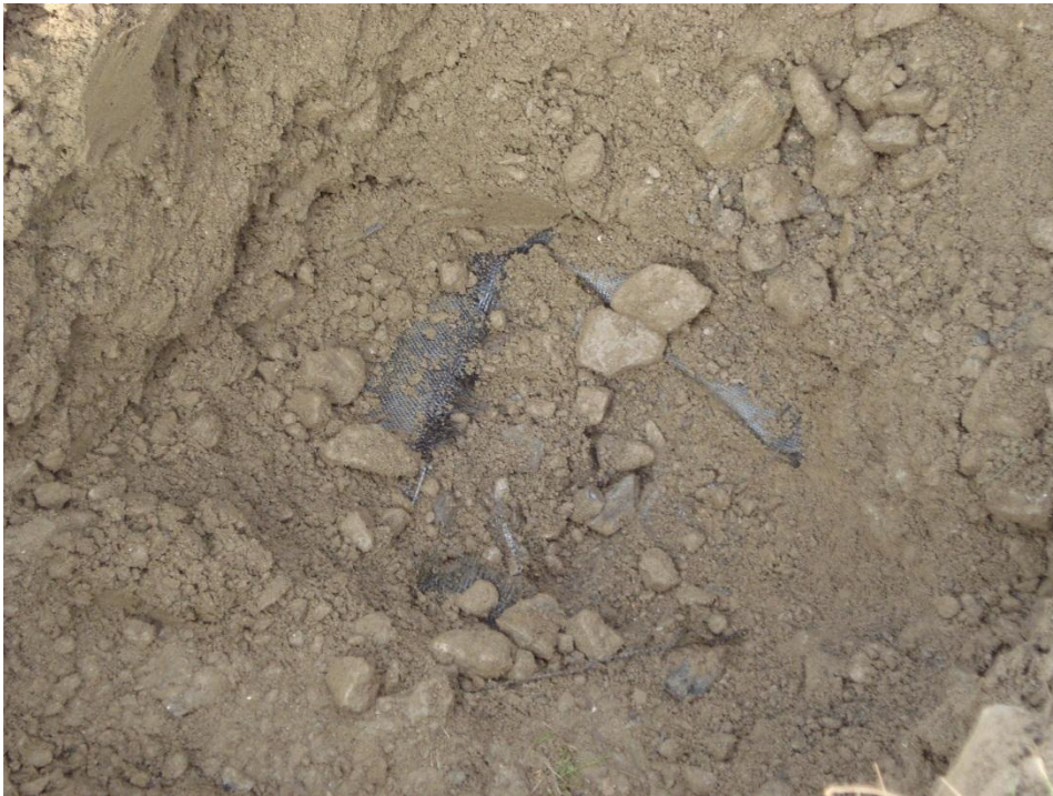
Site Photograph Number 4: Cut demarcation layer at GTB-15.
