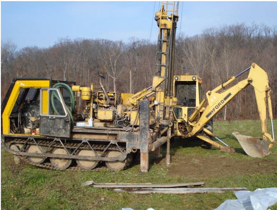
Site Photograph Number 6: Excavation backfilled around auger at GTB-15.
