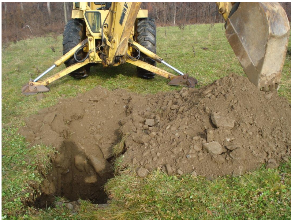
Site Photograph Number 2: Excavating down to demarcation layer at GTB-15.
