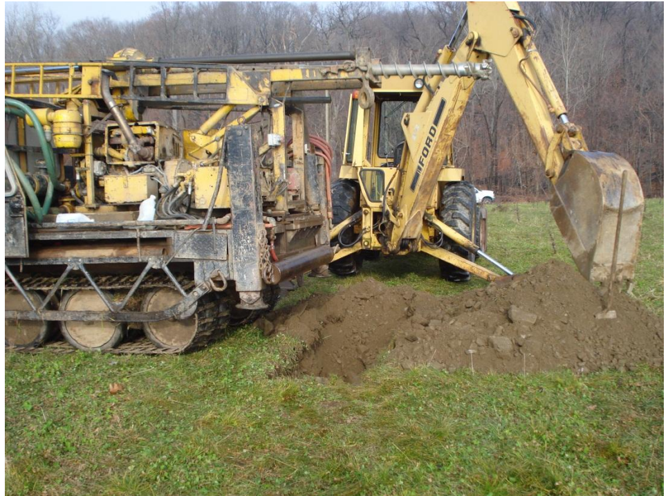
Site Photograph Number 5: Rig in place over excavation at GTB-15.
