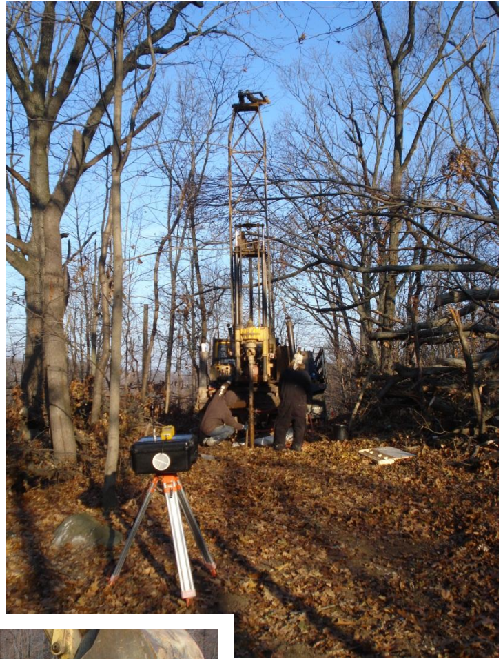
Site Photograph Number 1: Community air monitoring setup while drilling GTB-3.
