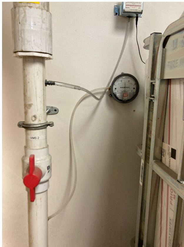
Photograph 16: Vacuum Reading at extraction point EP-2 inside post office
