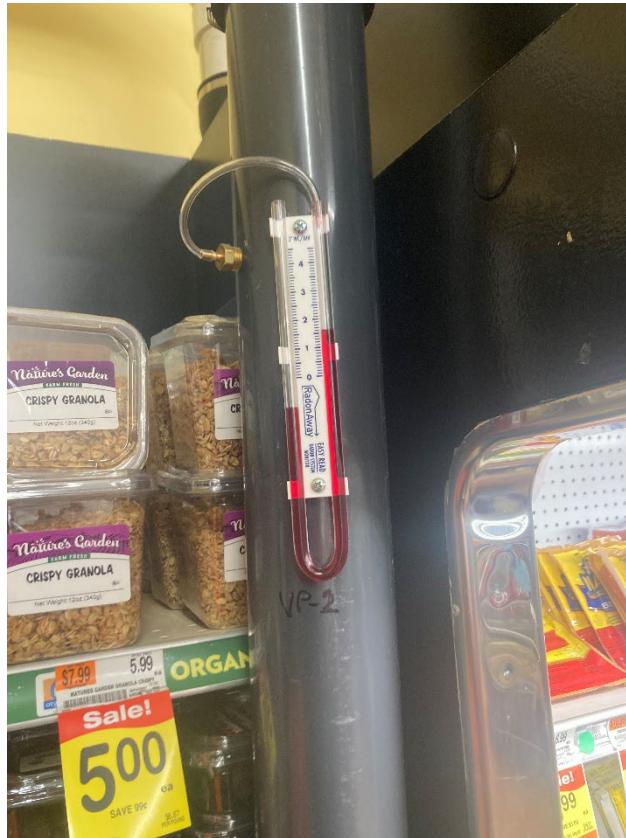
Photograph 4: Vacuum Reading at extraction point VMP-2 inside ACME Grocery Store
