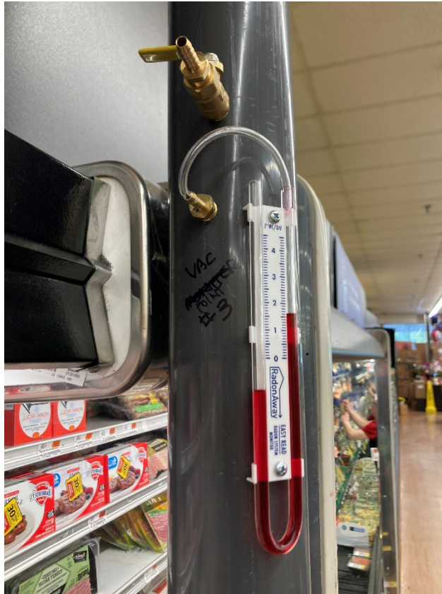
Photograph 5: Vacuum Reading at extraction point VMP-3 inside ACME Grocery Store
