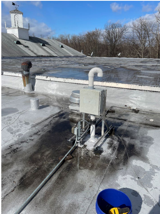
Photograph 22: [2/24/23] Obar Systems fan reinstalled at EP-1
