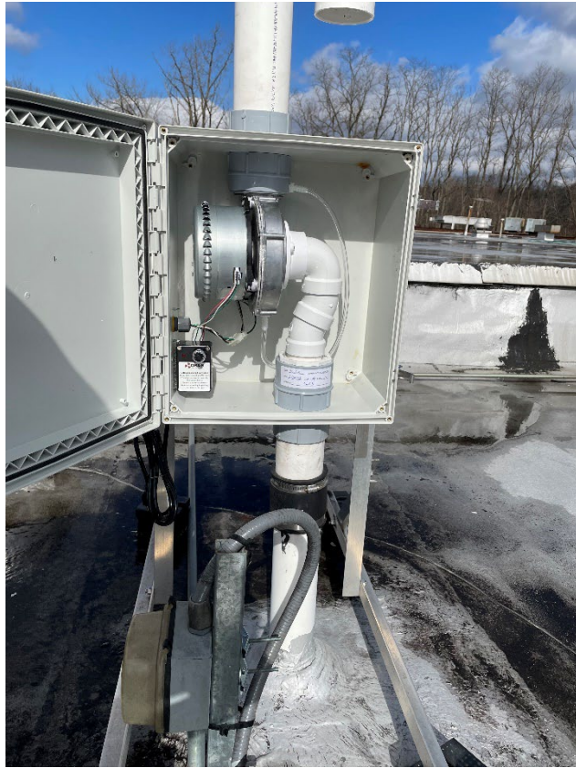
Photograph 21: [2/24/23] Obar Systems fan reinstalled at EP-1
