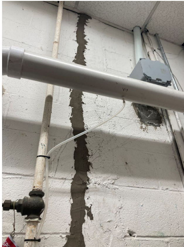
Photograph 12: [5/13/22] Sampling port located on combined header inside ACME Grocery Store (V-3)
