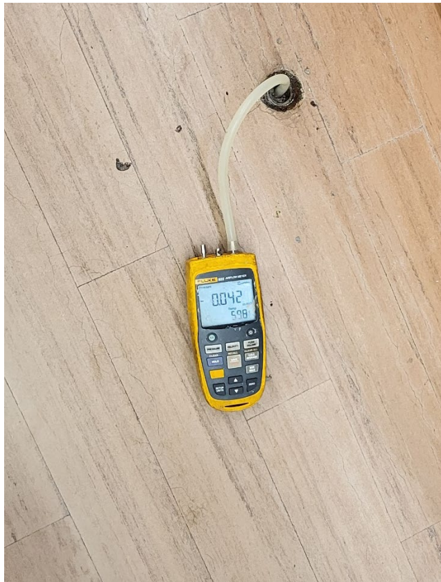
Photograph 3: [5/13/22] Vacuum Reading at monitoring point MP-3 inside ACME Grocery Store
