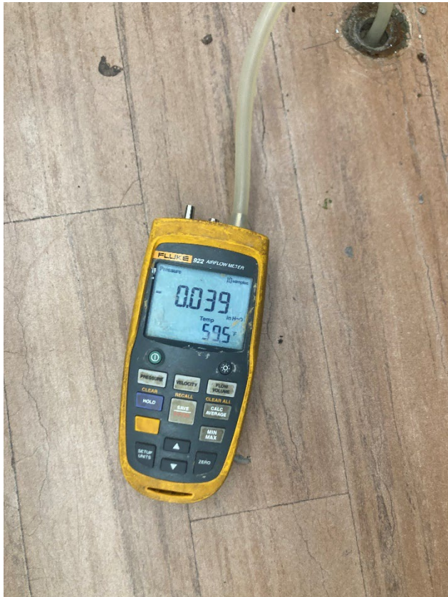
Photograph 2: [5/13/22] Vacuum Reading at monitoring point MP-2 inside ACME Grocery Store
