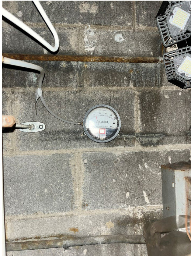
Photograph 23: [2/24/23] Vacuum Reading at extraction point EP-1 inside dry cleaner
