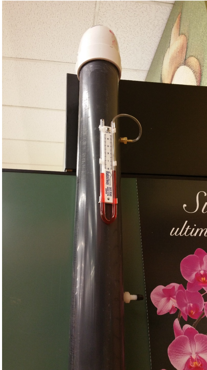
Photo 3 – View of manometer and sampling port on extraction pipe at sample location 2830-SS-3.
