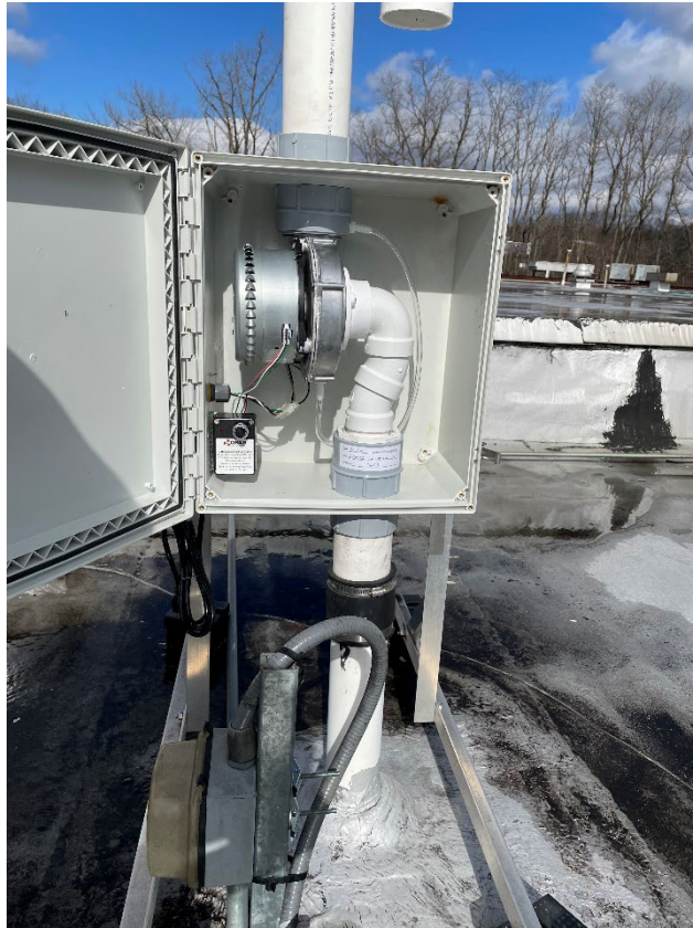
Photograph 21: [2/24/23] Obar Systems fan reinstalled at EP-1
