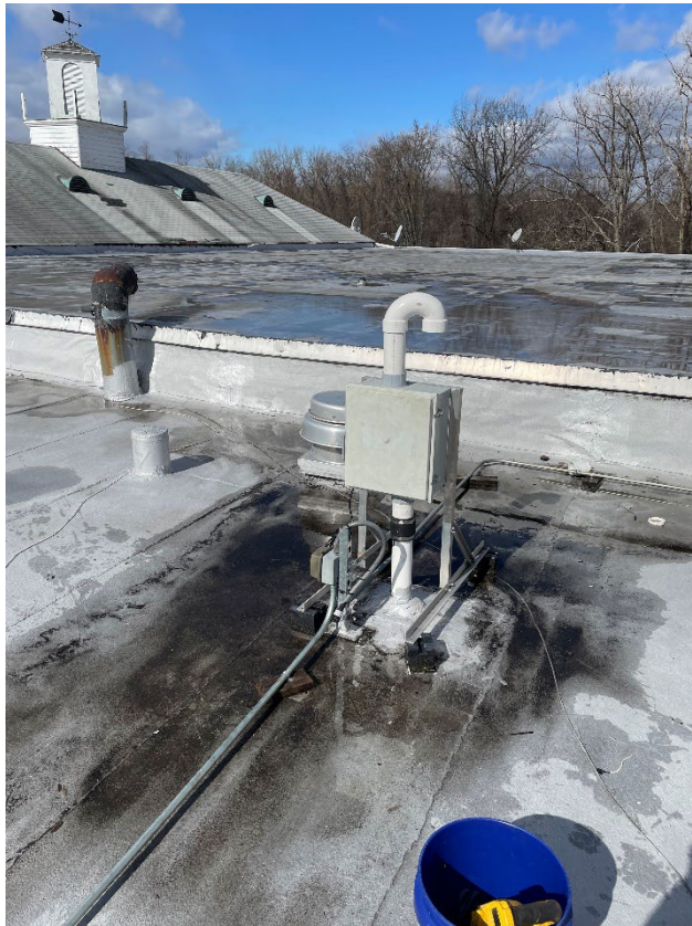
Photograph 22: [2/24/23] Obar Systems fan reinstalled at EP-1
