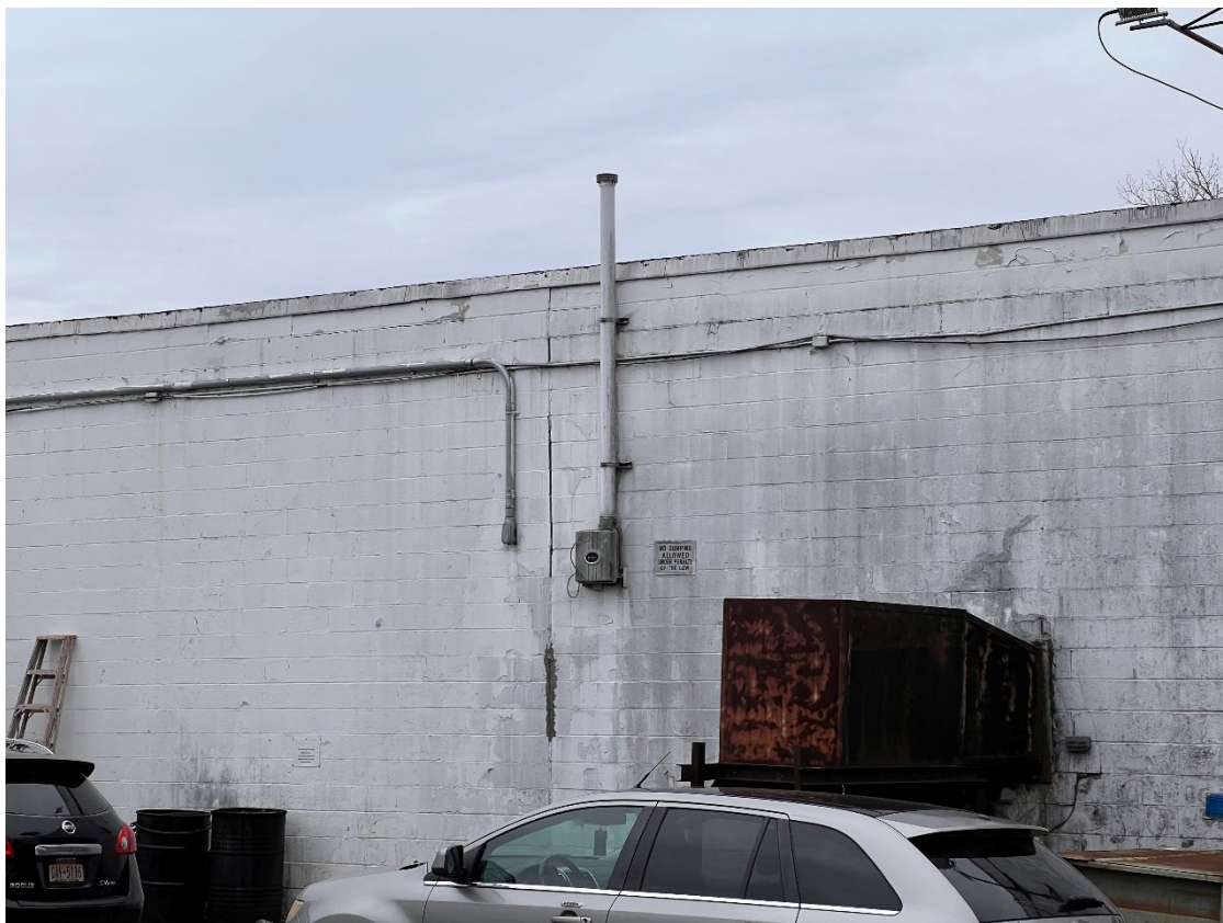
Photograph 11: [5/13/22] View of fan connected to VMP-1 through VMP-3 located outside ACME Grocery Store
