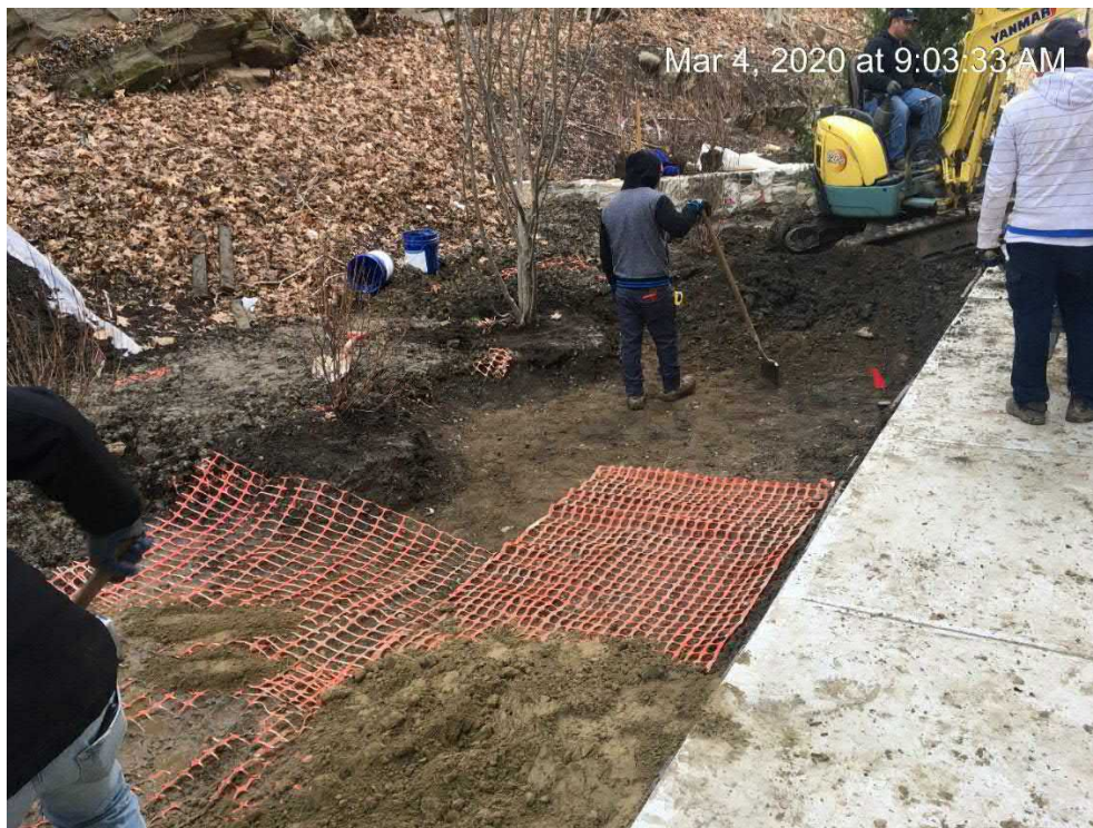
Clay and demarcation layer installation behind the hotel
