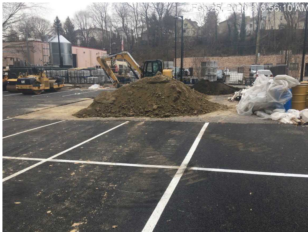
Clay (foreground) and topsoil (background) stockpiles
