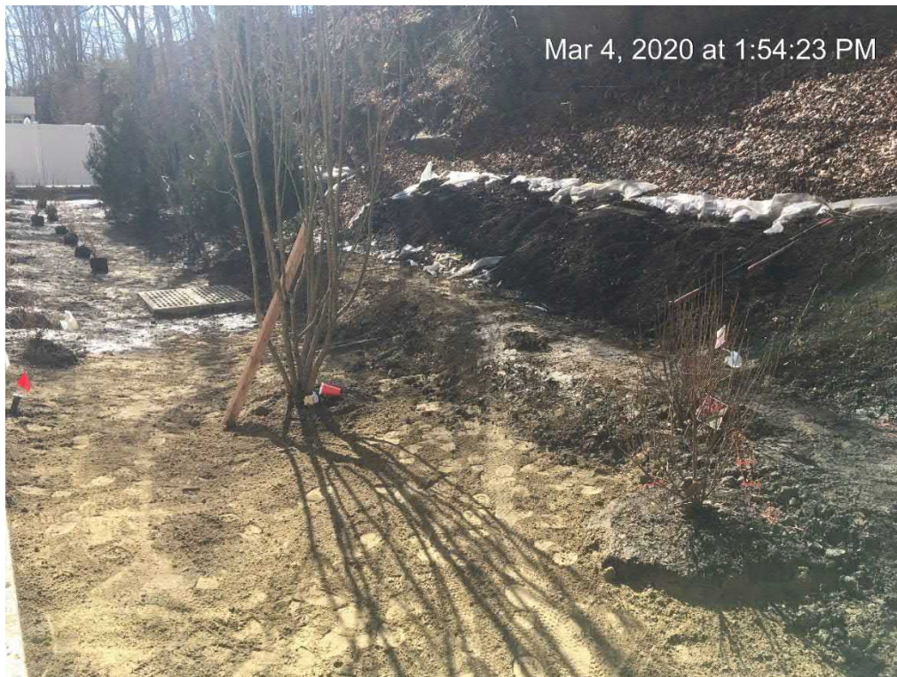
Area behind the hotel following clay installation
