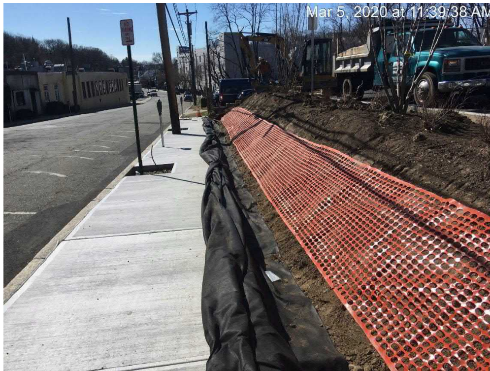
Slope on eastern property boundary following demarcation layer installation
