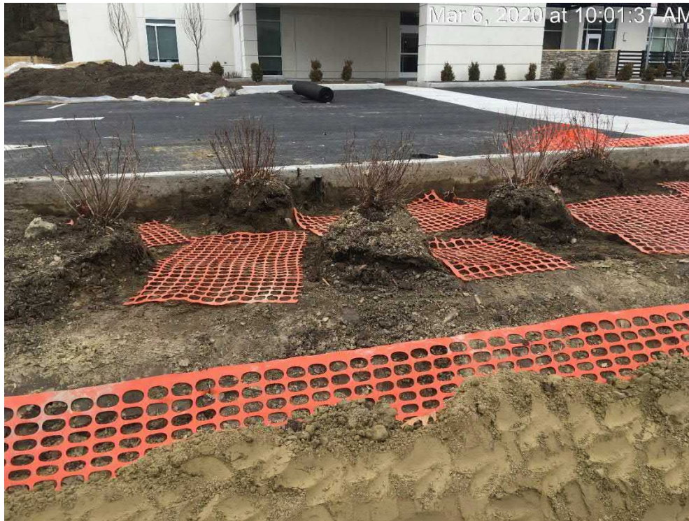
Demarcation layer installed at top of slope
