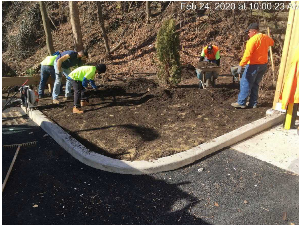
Mulch being removed prior to cap restoration
