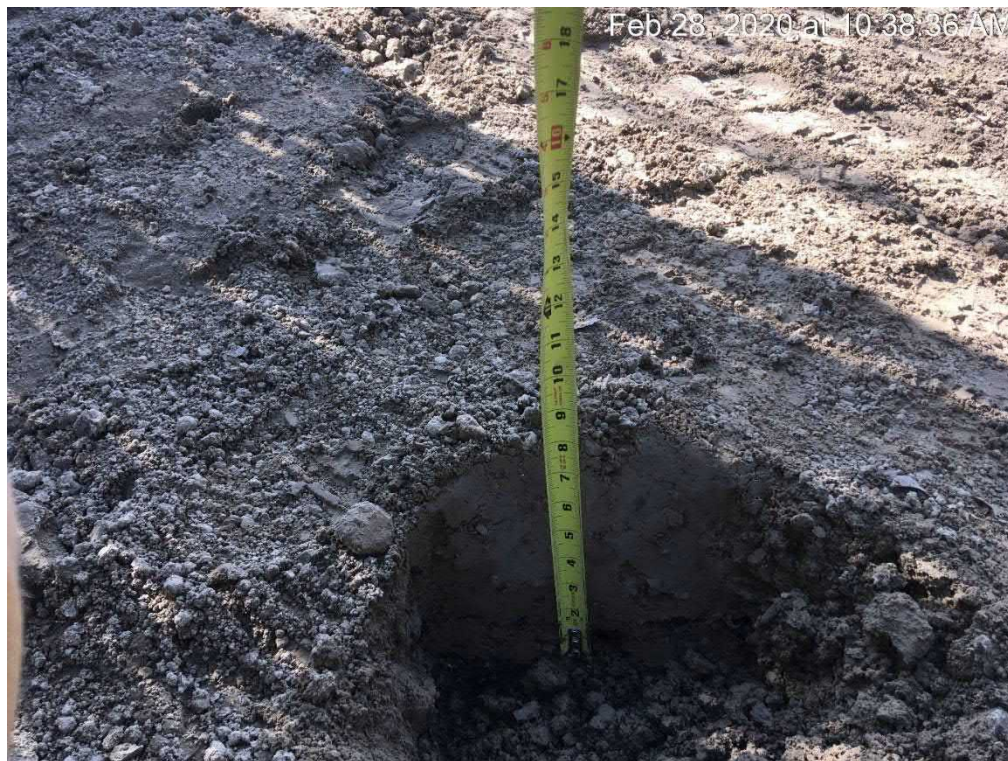
Inspection of clay layer thickness
