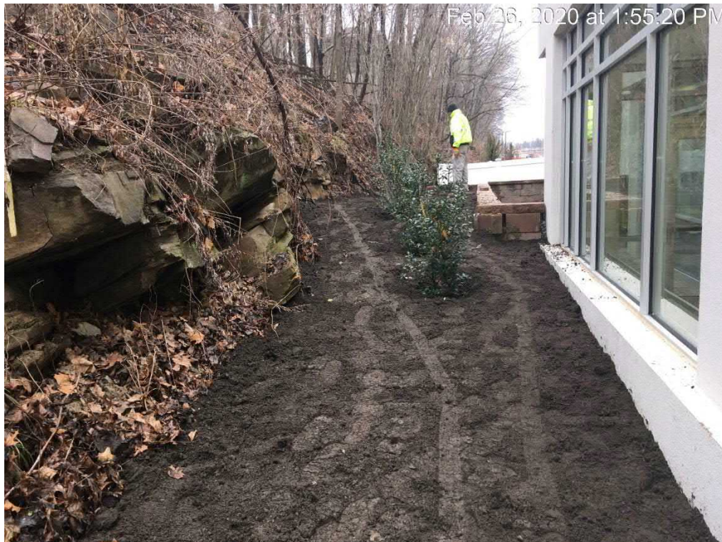
Topsoil installed in area behind pool
