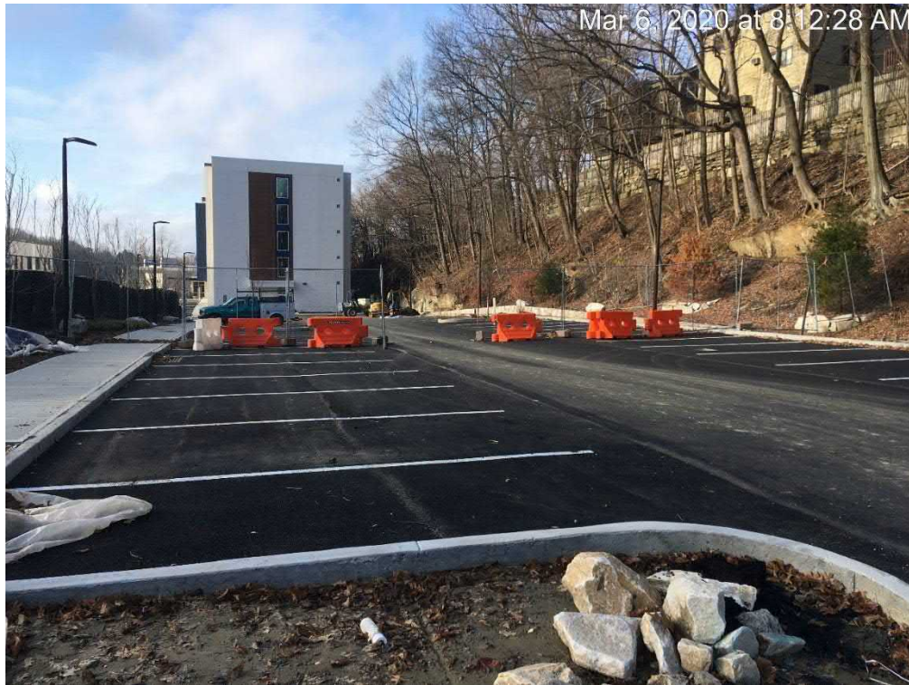
Location of temporary fence
