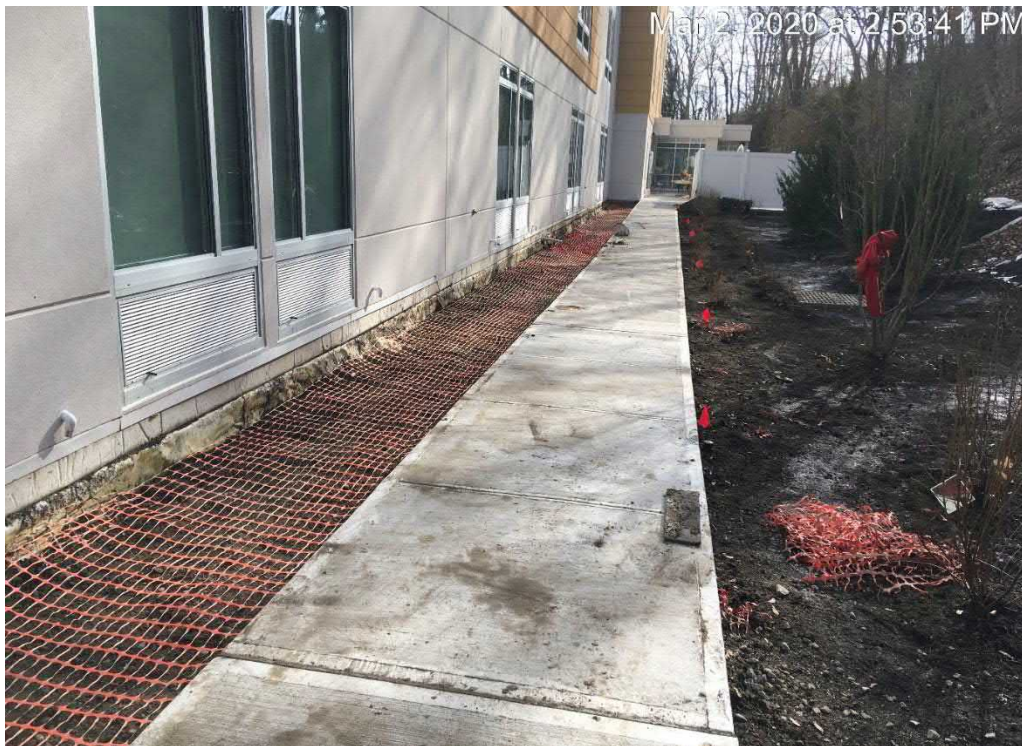
Demarcation layer installation in area behind hotel
