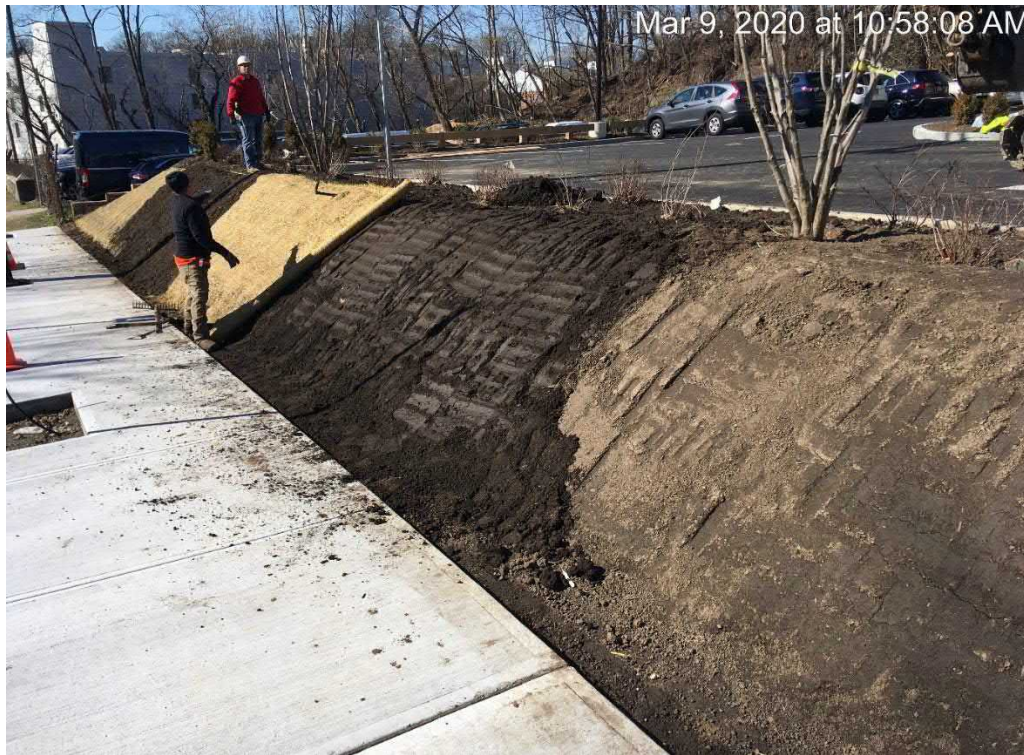
Erosion control matting installation over topsoil on slope
