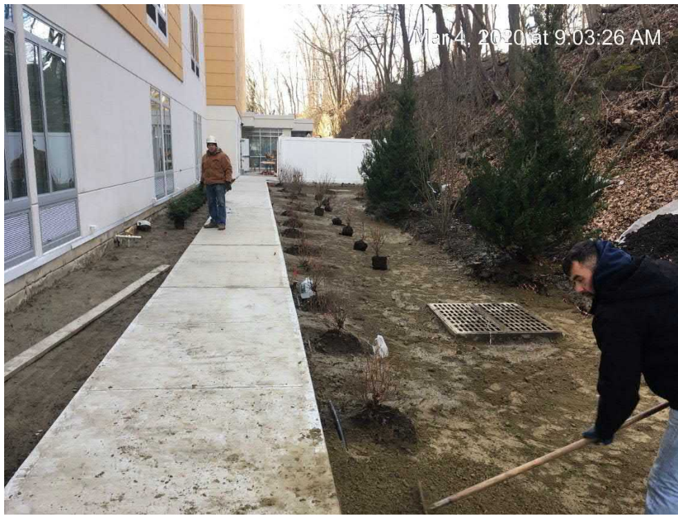
Clay installation behind hotel
