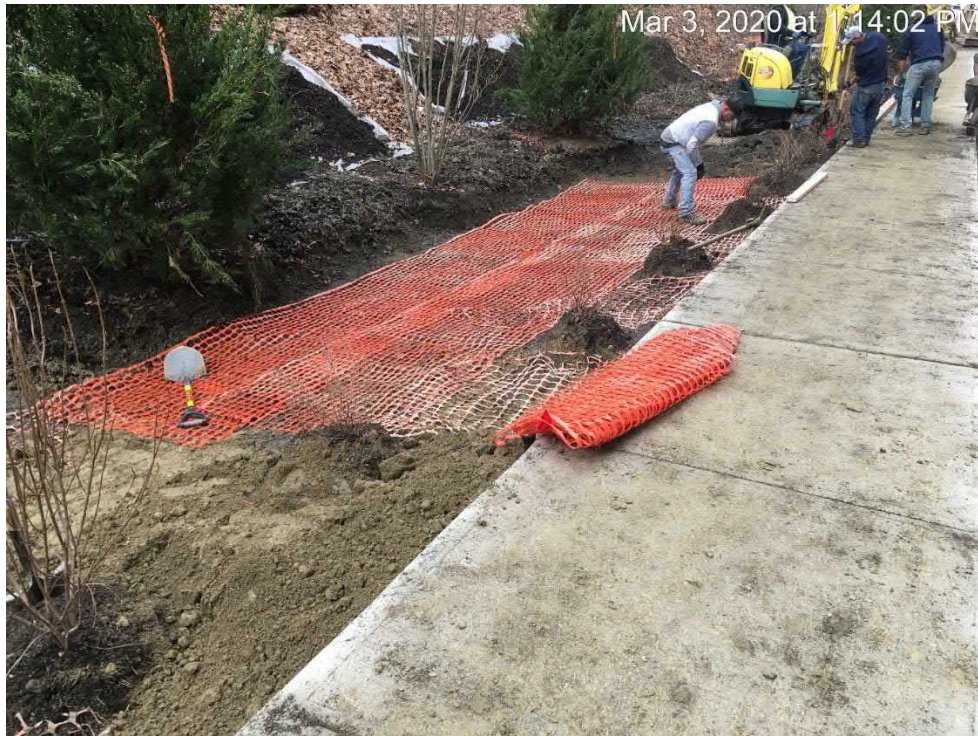
Demarcation layer installation in area behind hotel
