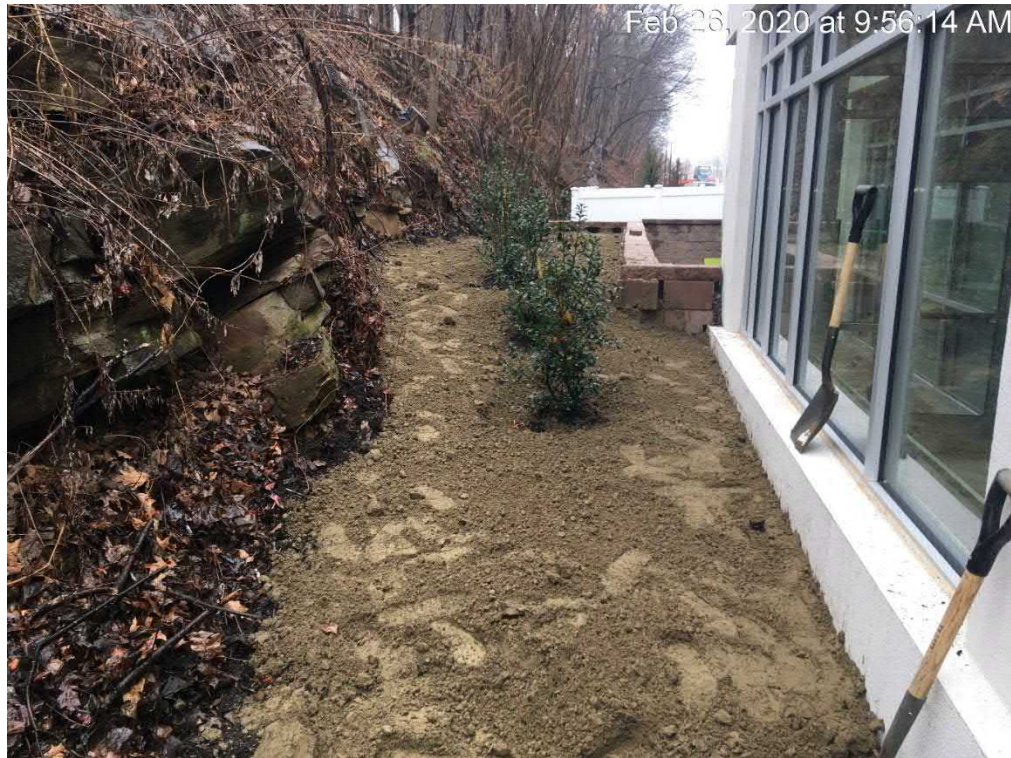
Clay installed in area behind pool
