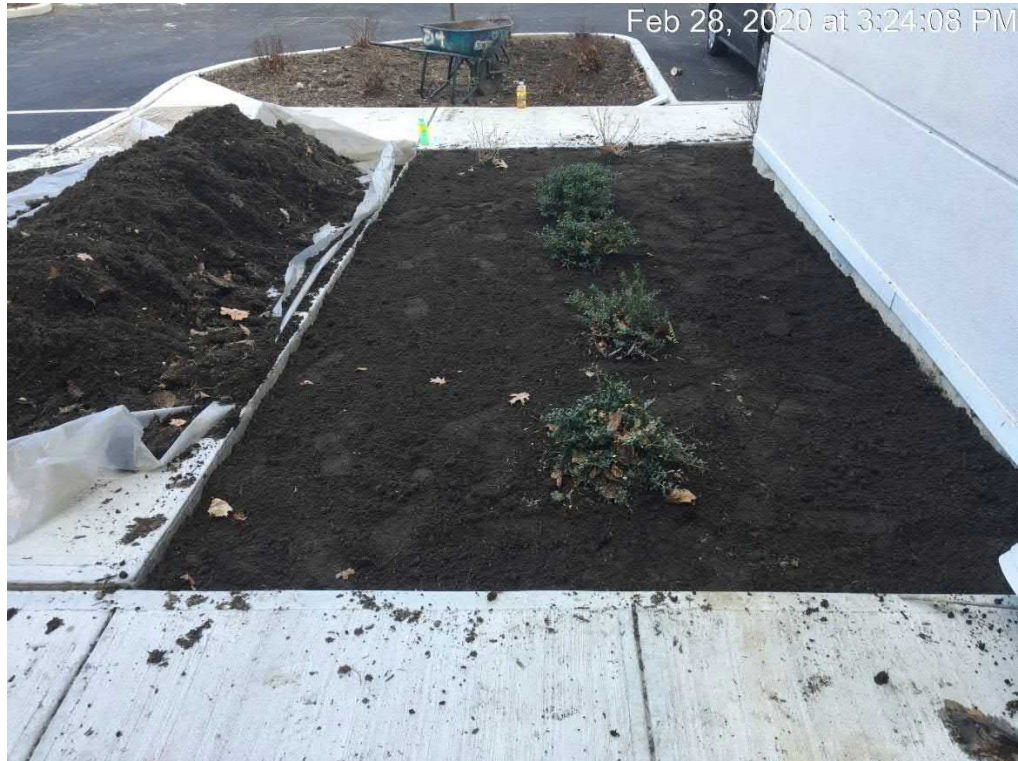
Northeast corner of hotel following topsoil install
