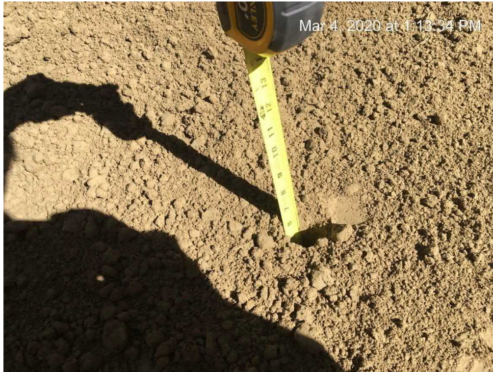
Clay layer thickness inspection
