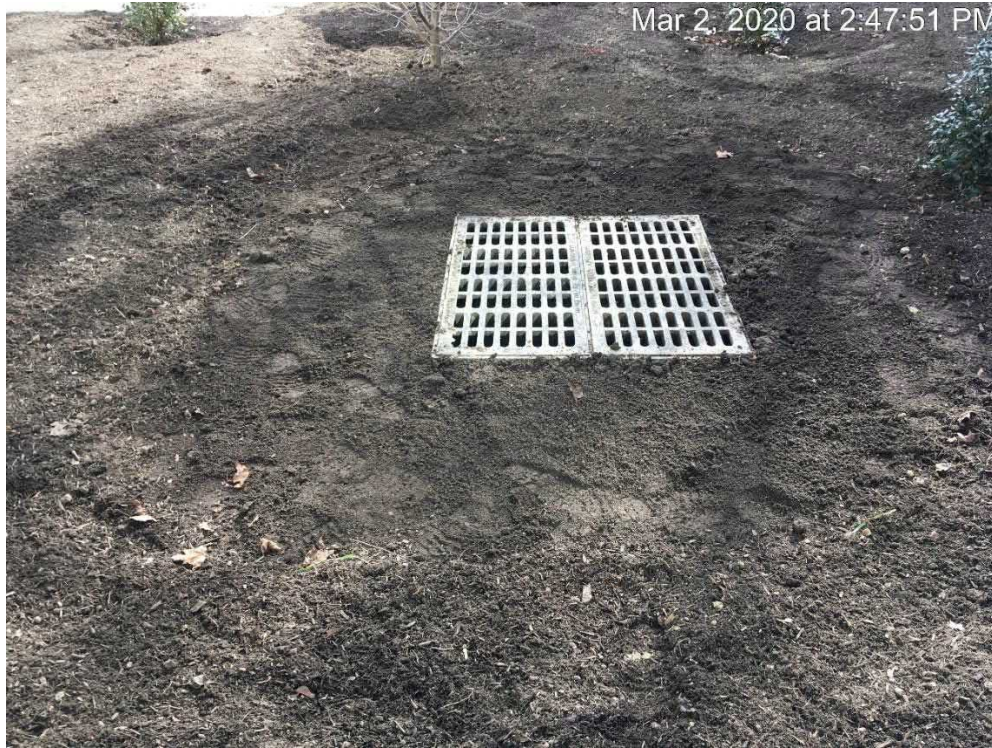
Storm drain behind the hotel following installation of clay and topsoil
