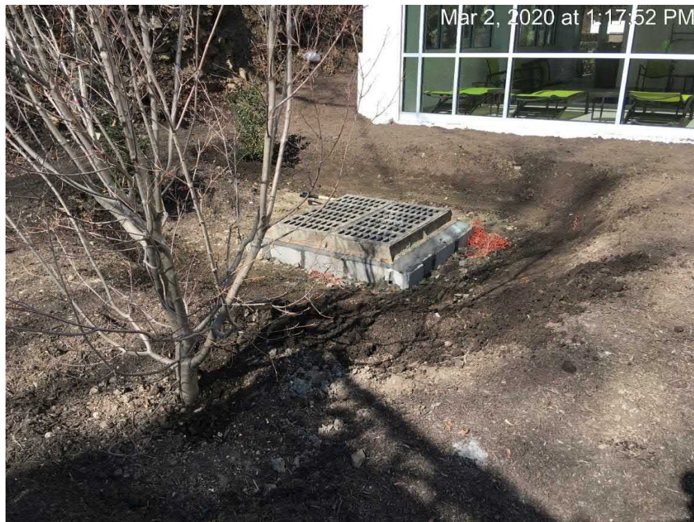
Storm drain behind the hotel following re-installation
