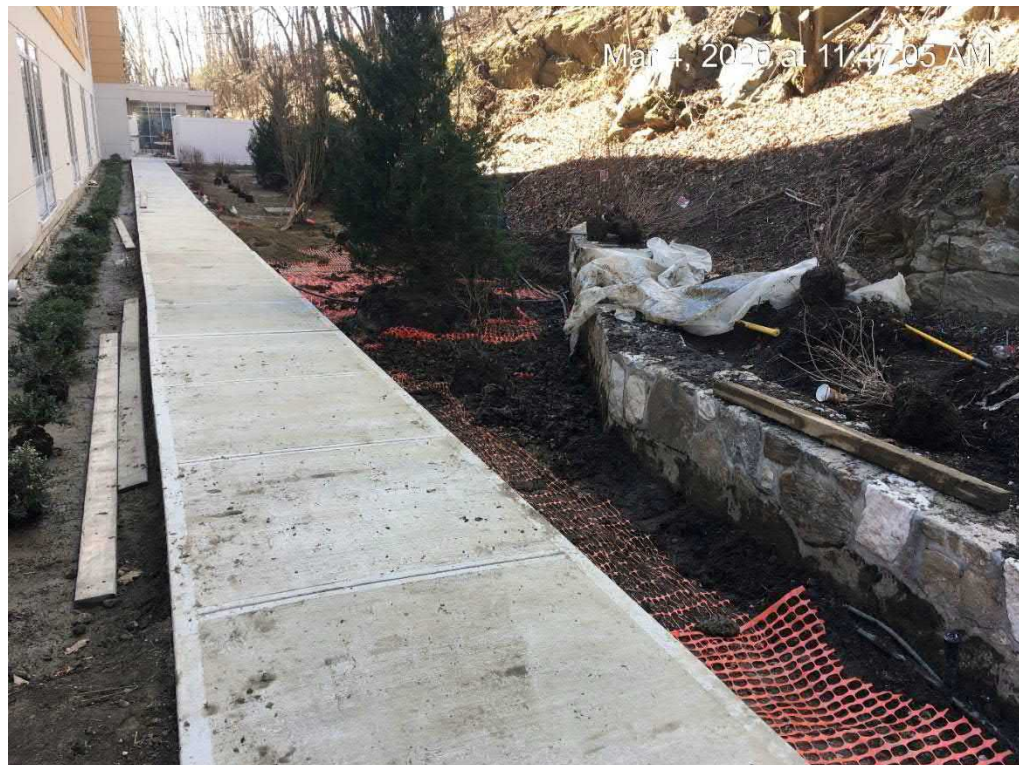
Demarcation layer installation behind the hotel
