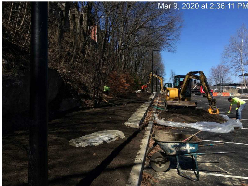
Cap installation at site's western boundary
