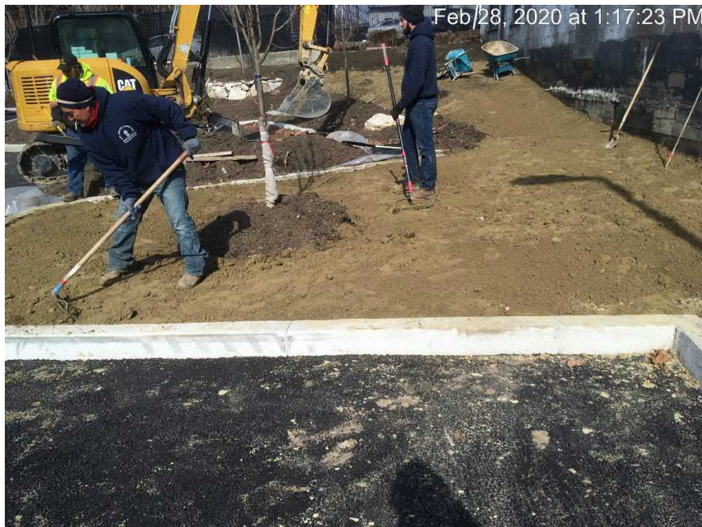
Clay installation at the site's eastern property boundary
