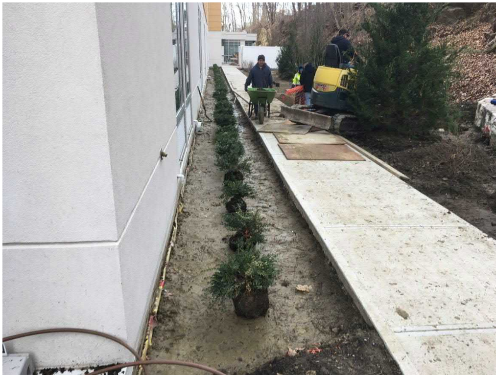
Clay installation behind hotel
