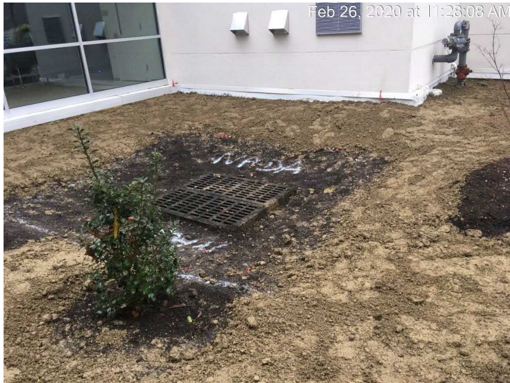
Clay installed in area behind hotel, prior to removal and re-installation of storm drain
