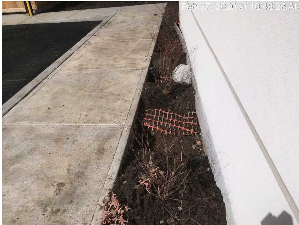
Soil removed around plants before clay install
