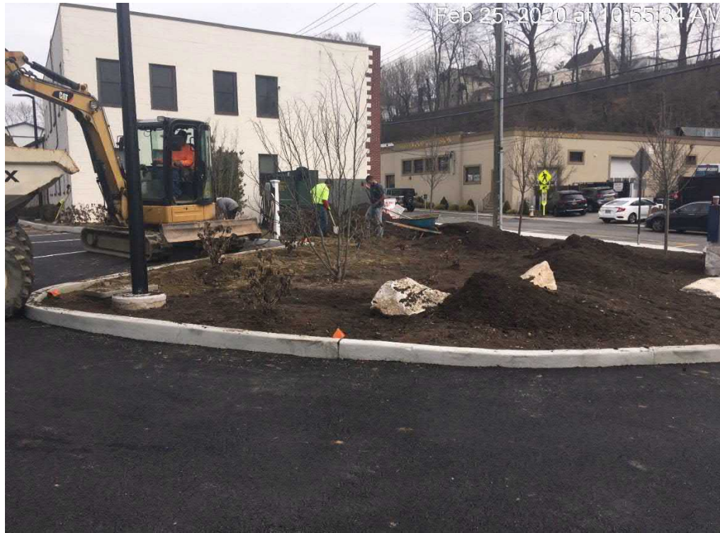
Mulch and soil being removed from area prior to cap installation
