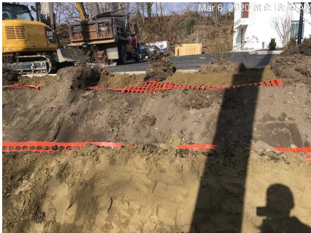
Clay installation on eastern property boundary slope
