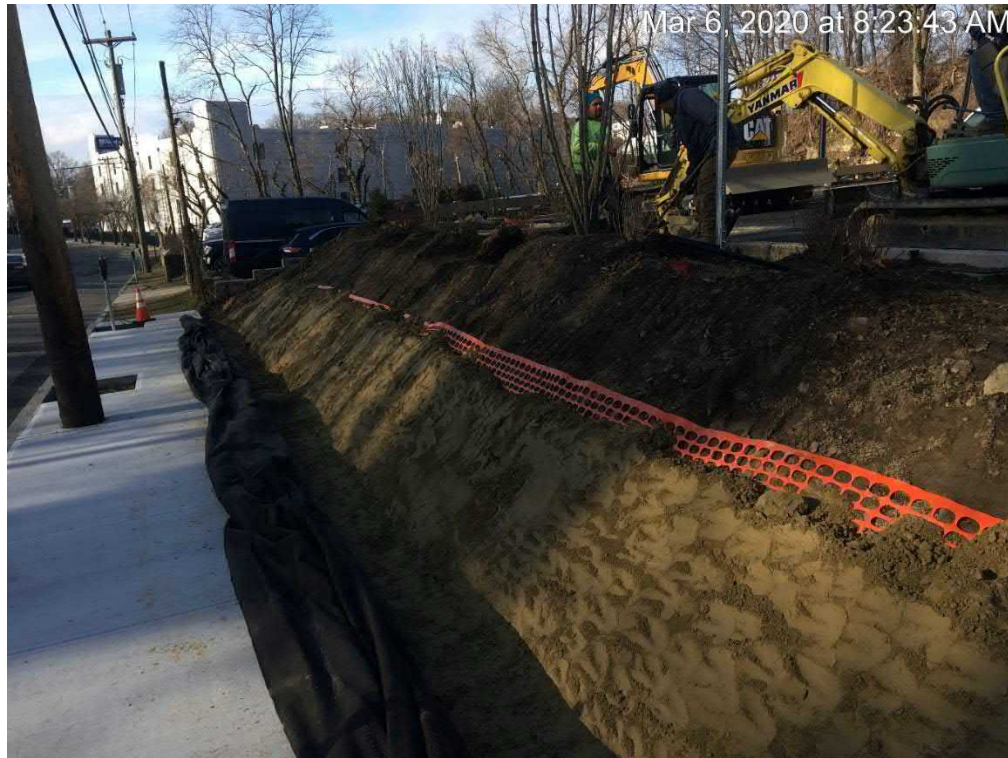
Clay installation on eastern property boundary slope
