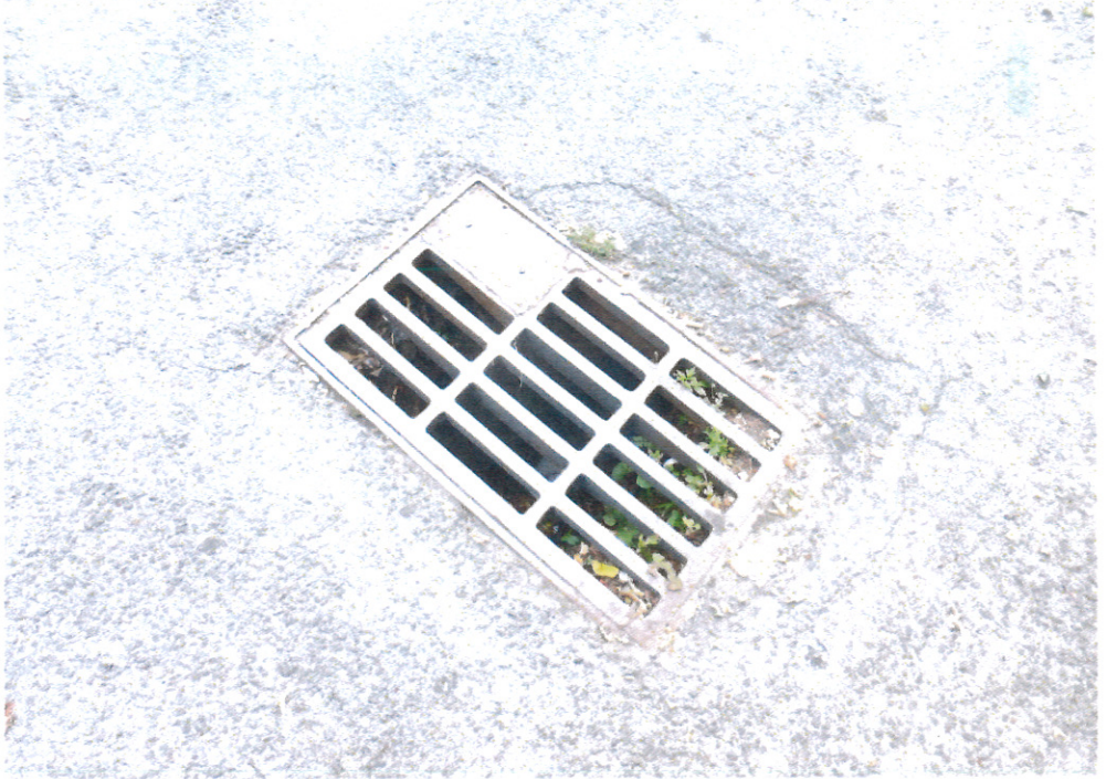
CATCH BASIN IN CENTRAL PORTIONS OF THE SITE
