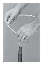
Figure 3. Engaging threads by rotating tubing.
