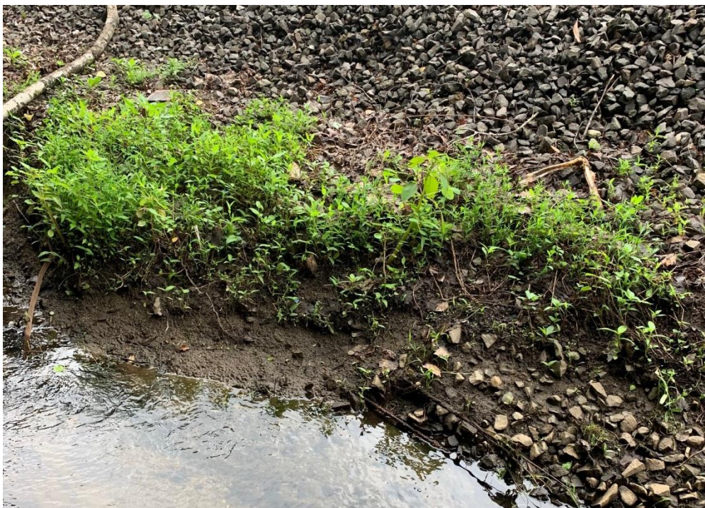
Photo 2: Exposed fill from railway embankment eroding to Branch Brook (facing east)
