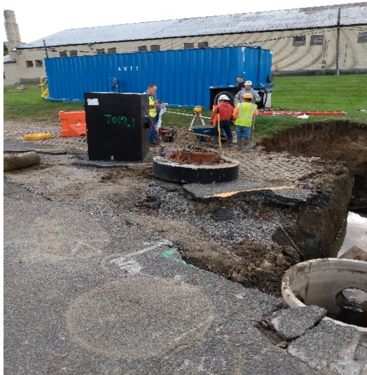
Photo 12 – Placing MH 7017.1
