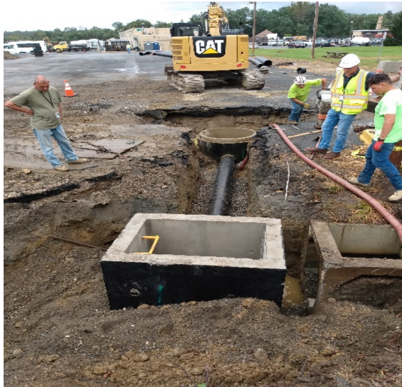
Photo 10 – Pipe in place MH 7016 to 7016.1
