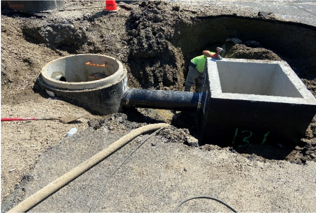
Photo 1 – Connection at MH 7013 and 7013.1
