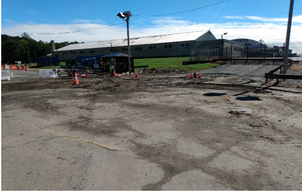
Photo 11 – Backfill completed MH 7016 area
