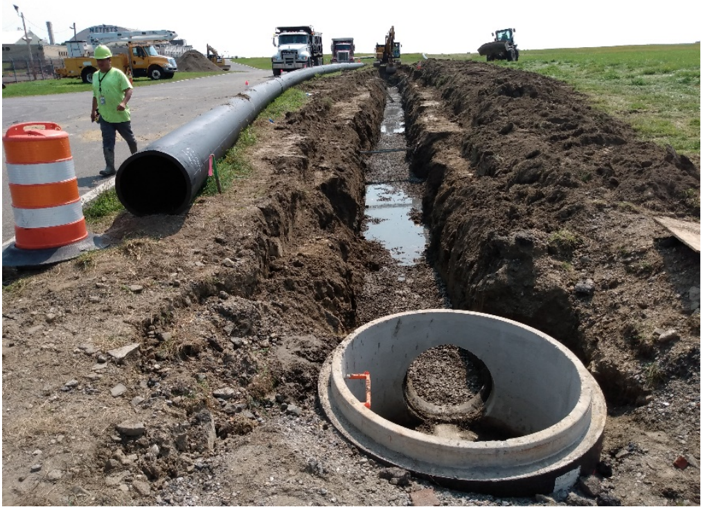
Photo 5 – Trenching MH 7023 to 7024
