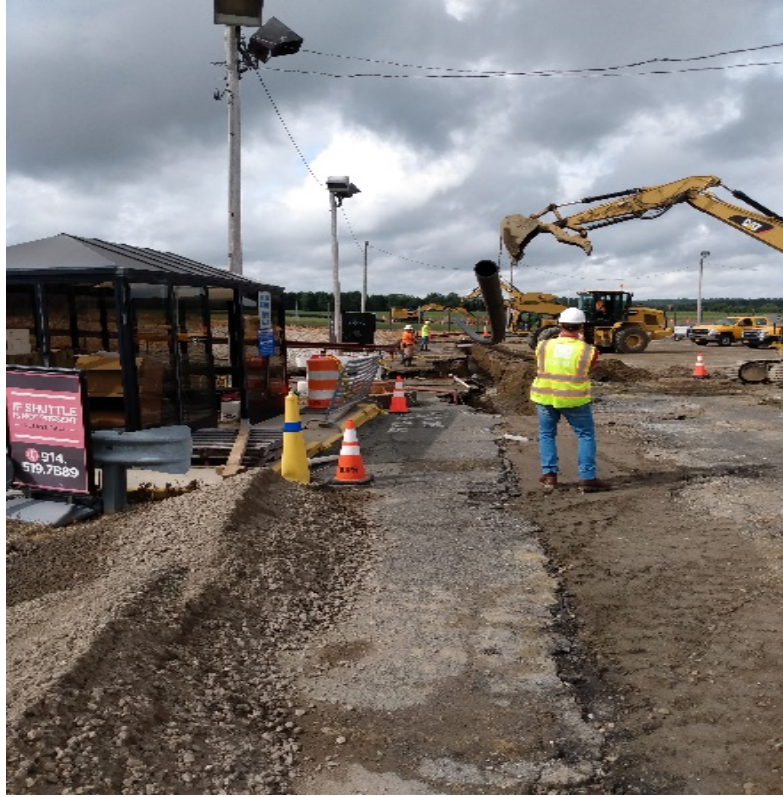
Photo 9 – Placing pipe from MH 7015 to MH 7016 over altered water main
