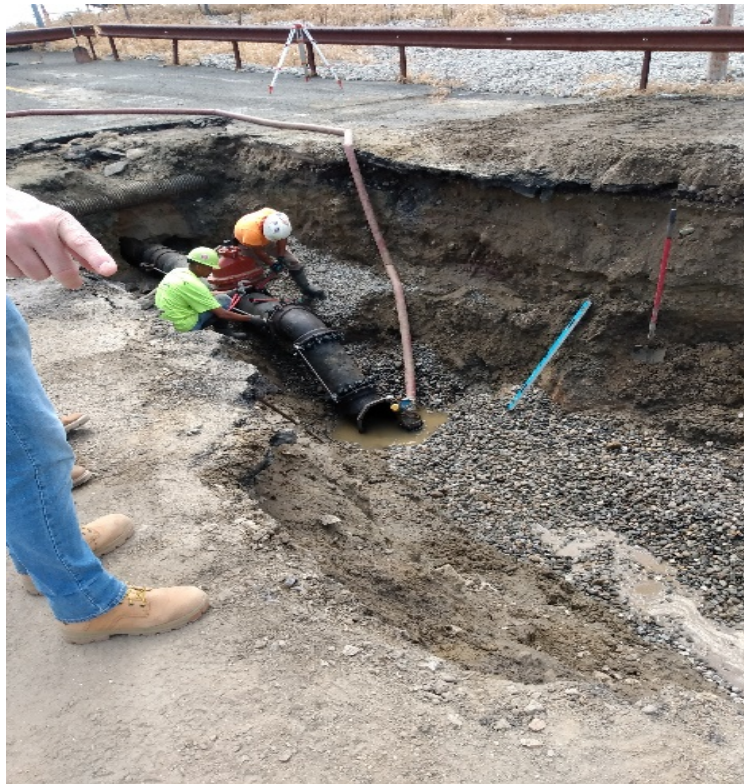
Photo 8 – Water main undergoing alteration
