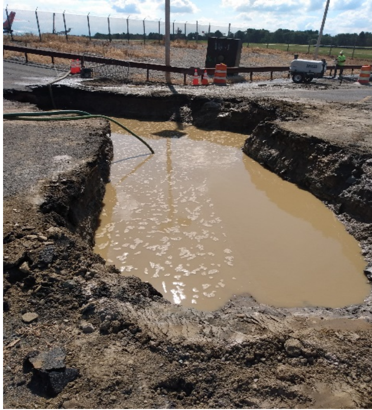
Photo 7 – Excavation after water main leak
