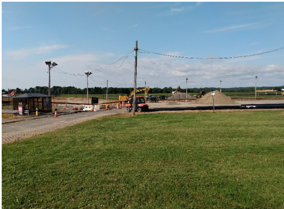
Photo 4 – Work area September 13, 2021
