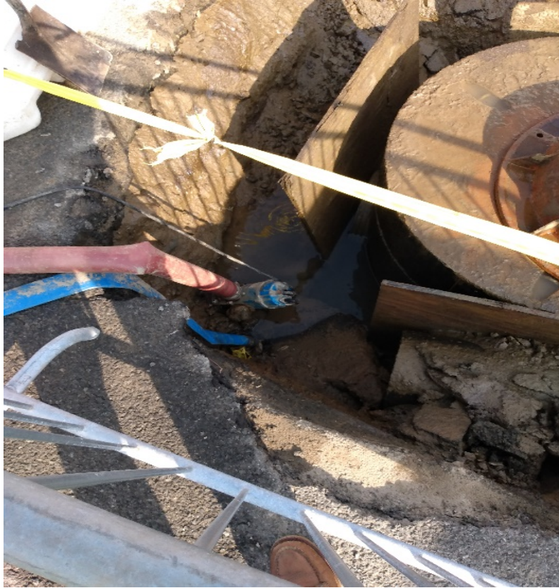
Photo 3 – Typical pump placement for dewatering
