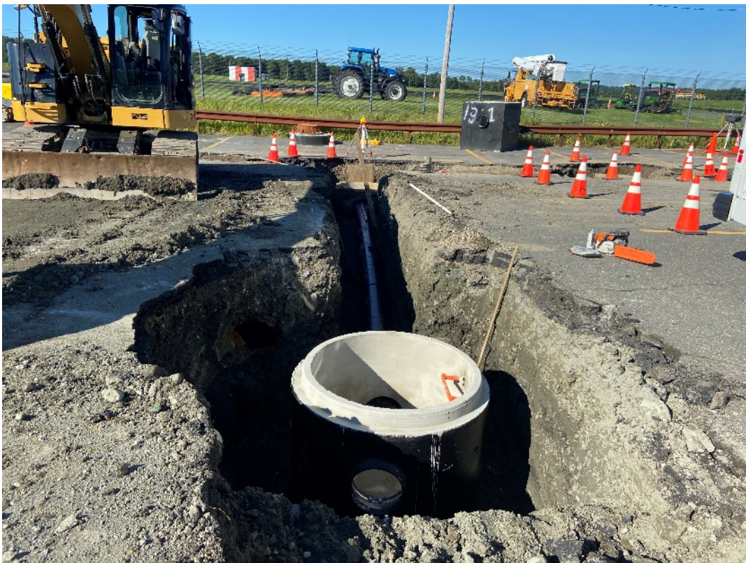
Photo 2 – Trenching from MH 7013.2 to 7013
