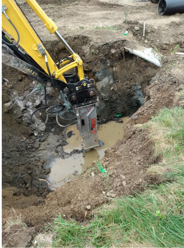
Photo 3 – Breaking up bedrock prior to placing bedding
