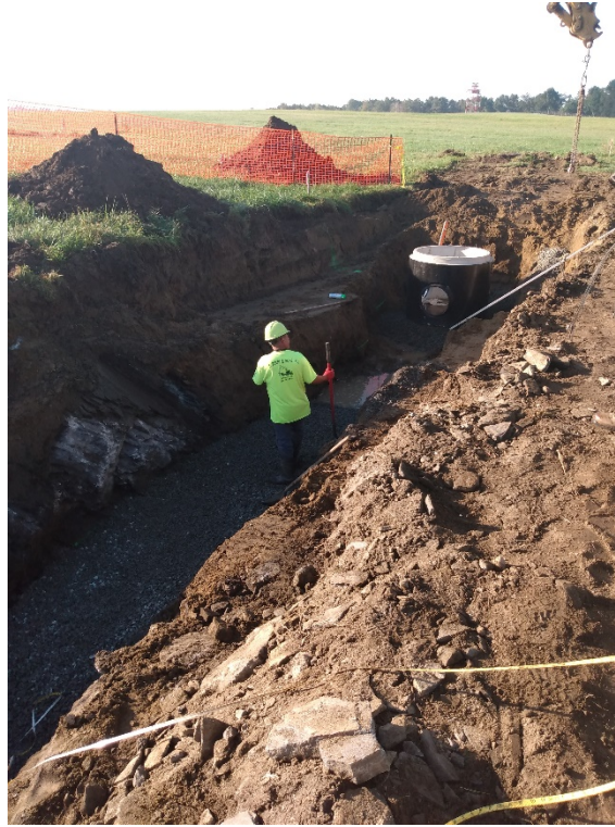
Photo 5 – Trenching MH 7024.2 to 7025
