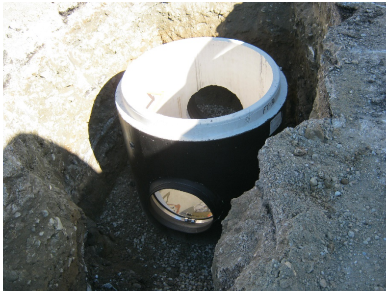
Photo 10 – MH-7027 in place
