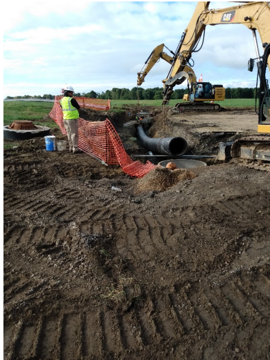
Photo 4 – Placement of pipe, MH-7024 to MH-7024.2
