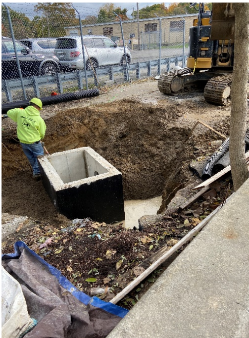
Photo 14 – CB-7029.5 in place
