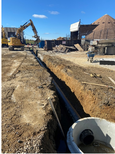
Photo 15 – Pipe laid from MH-7029.4 to 7029.1
