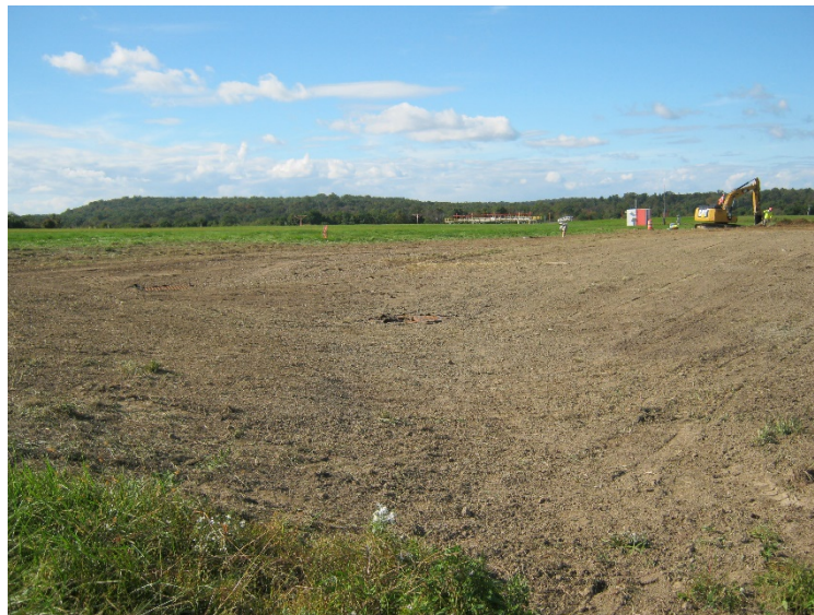
Photo 6 – Finished grade, vicinity of MH-7026
