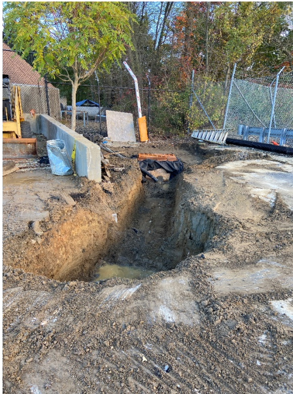
Photo 16 – Trenching between catch basin 7029.5 and MH-7029.4
