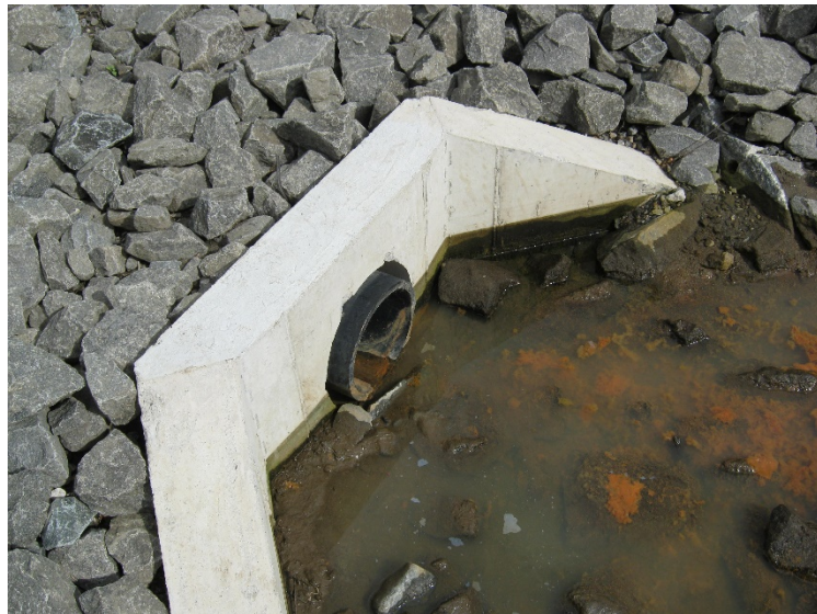
Photo 8 – Corrective action for Headwall 7015.1
