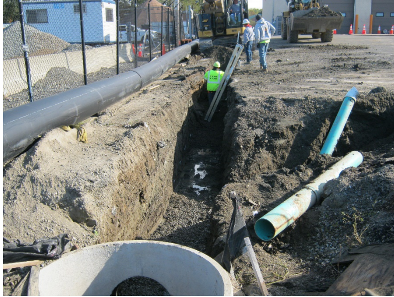
Photo 9 – Trenching from MH-7008 to MH-7027
