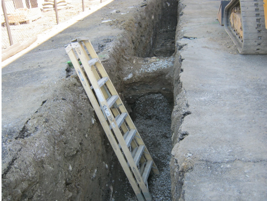
Photo 11 – Trenching MH-7027 to MH-7028 showing concrete cable run
