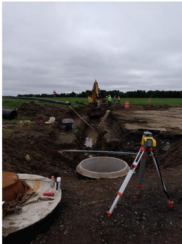
Photo 2 – Trenching from MH 7024 to 7024.2
