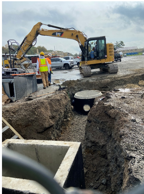
Photo 12 – Trenching between catch basin 7029.2 and MH-7029.1
