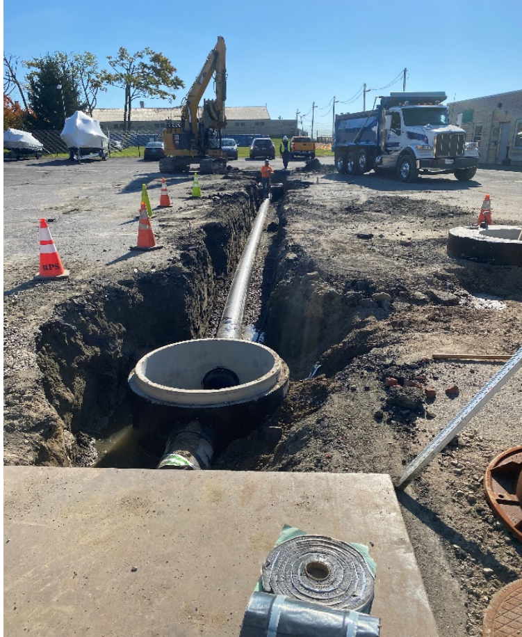
Photo 5 – Trenching MH 7032 to 7033
