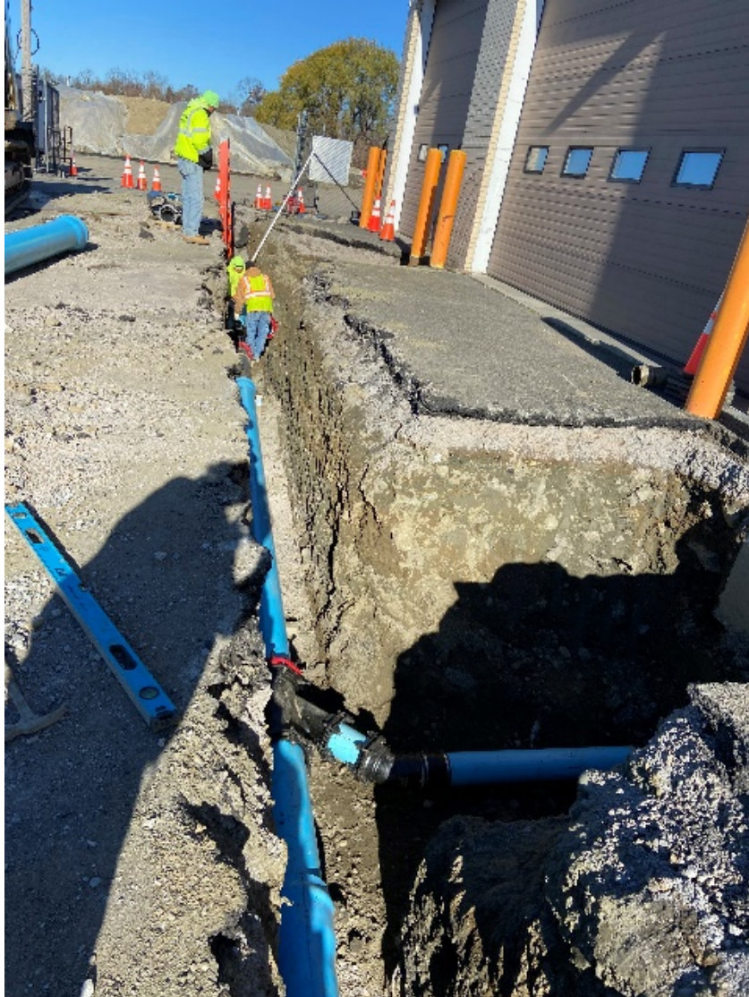
Photo 8 – Additional Roof Drain connections
