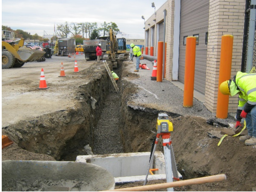
Photo 1 – Excavation between MH-7029 and MH-7030
