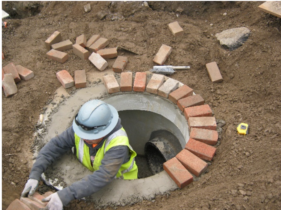
Photo 2 – Raising manhole chimney with brick and mortar, MH-7030
