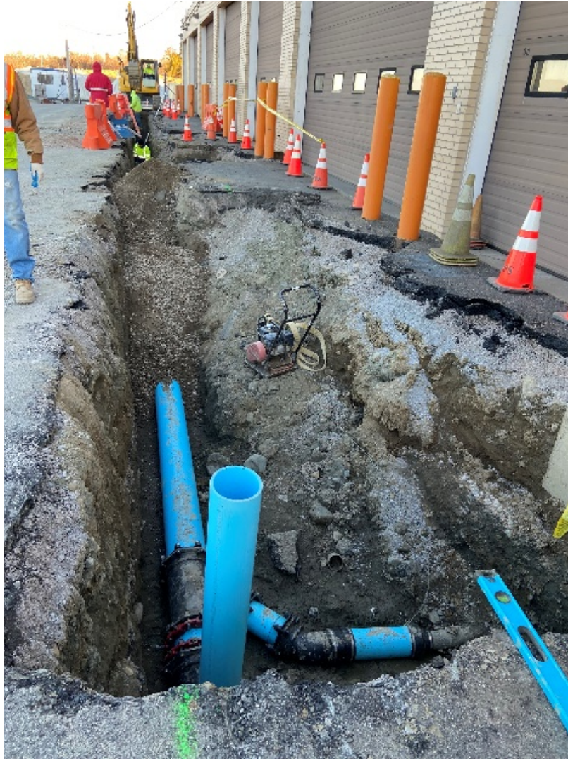
Photo 7 – New Roof Drain connections
