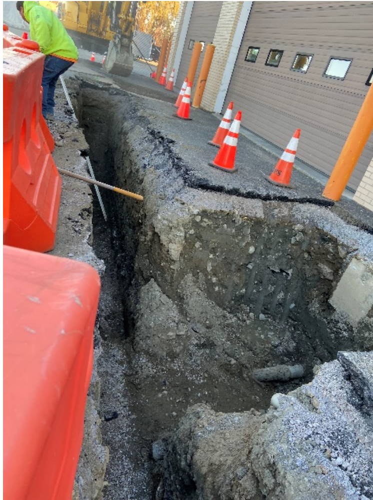
Photo 6 – Trenching for new piping, roof drains, behind Building 10
