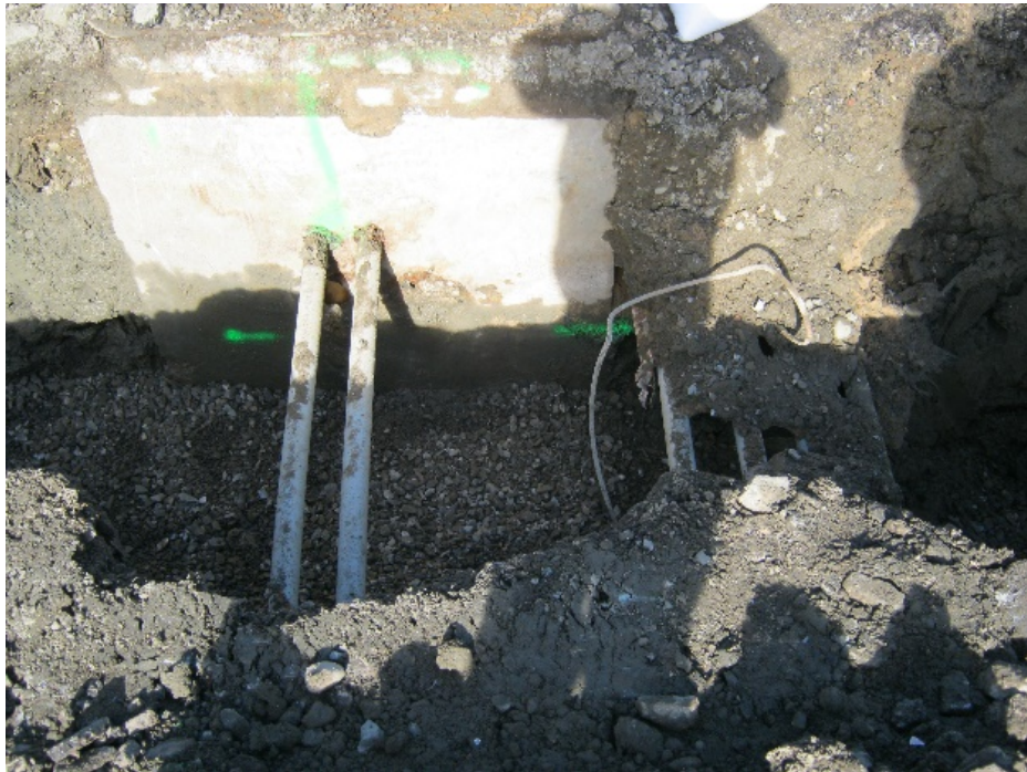
Photo 4 – Trenching, avoiding electrical utilities, between MH-7030 and MH-7030.1
