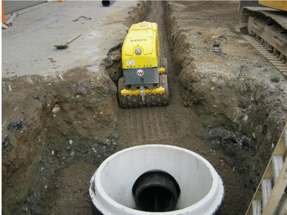
Photo 3 – Backfill and compaction between MH-7029 and MH-7030
