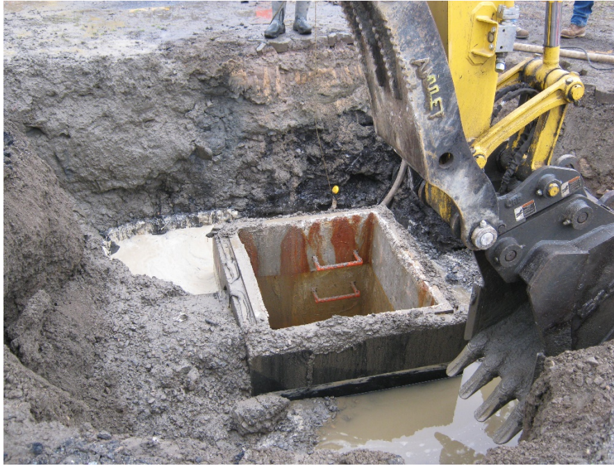
Photo 1 – MH-7013.3 during removal
