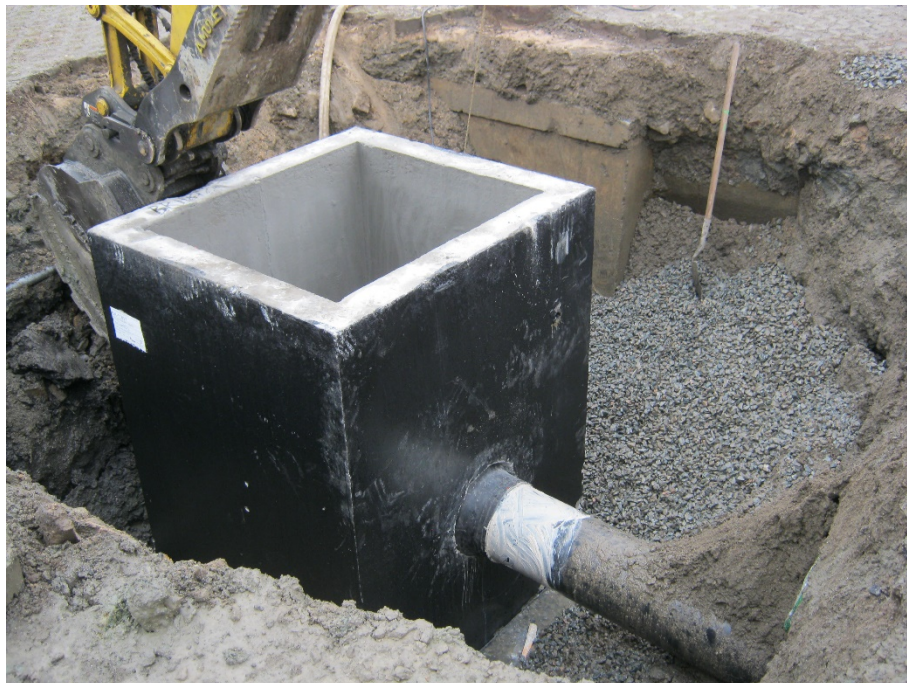
Photo 2 – MH-7013.3 after replacement with new single piece structure.
