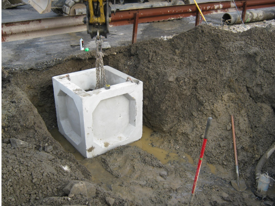
Photo 4 – Placing new inlet at MH-7015.1
