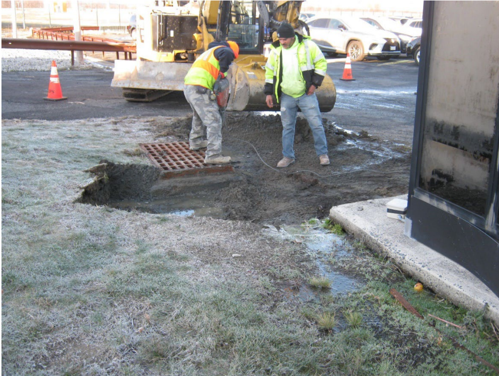
Photo 1 – Area of installation prior to excavation.
