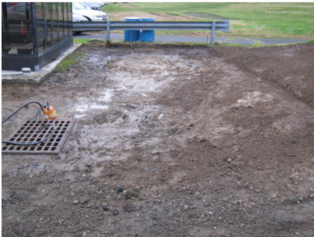
Photo 2 – Post excavation and contouring
