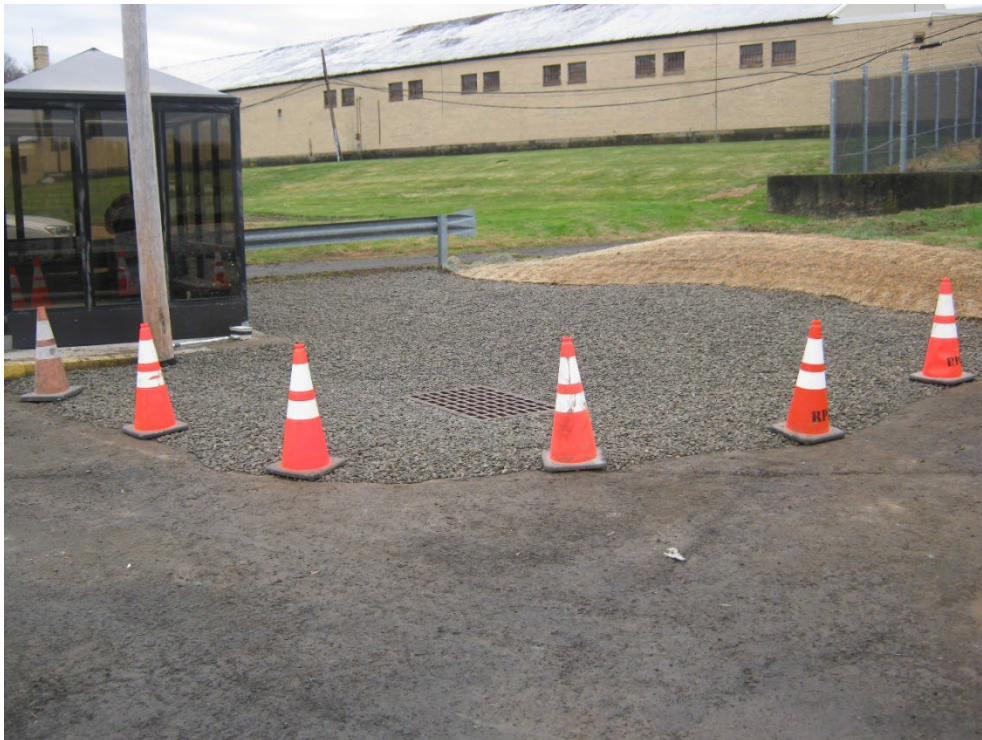
Photo 4 – Post installation with gravel cover, erosion control and traffic control.
