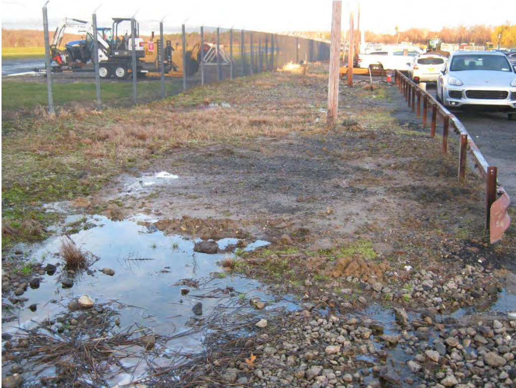
Photo 5 – 7014.2 Area of installation prior to excavation.
