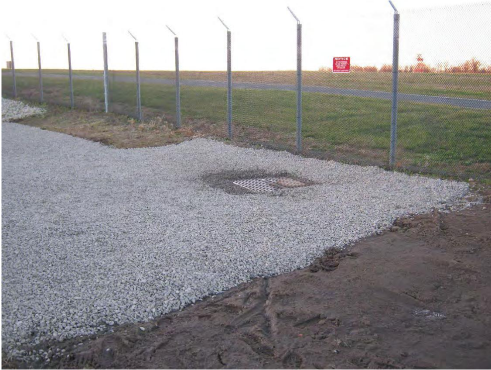
Photo 9 – 7014.2 Post installation with gravel cover and erosion control, part II.
