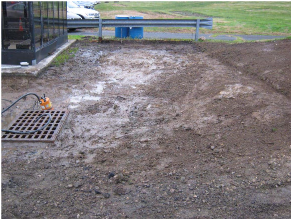
Photo 2 – 7016.1 Post excavation and contouring
