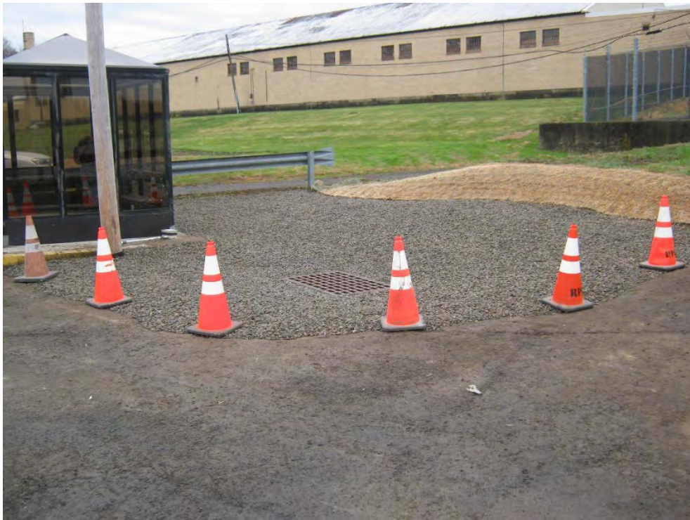
Photo 4 – 7016.1 Post installation with gravel cover, erosion control and traffic control.
