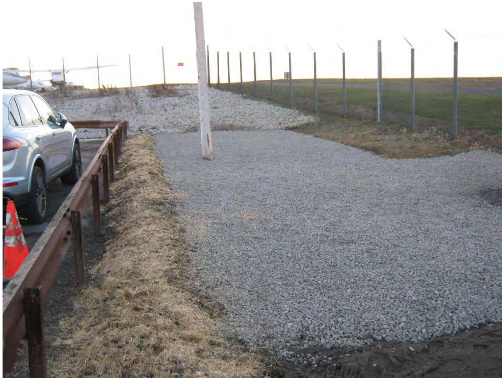
Photo 8 – 7014.2 Post installation with gravel cover and erosion control, part I.
