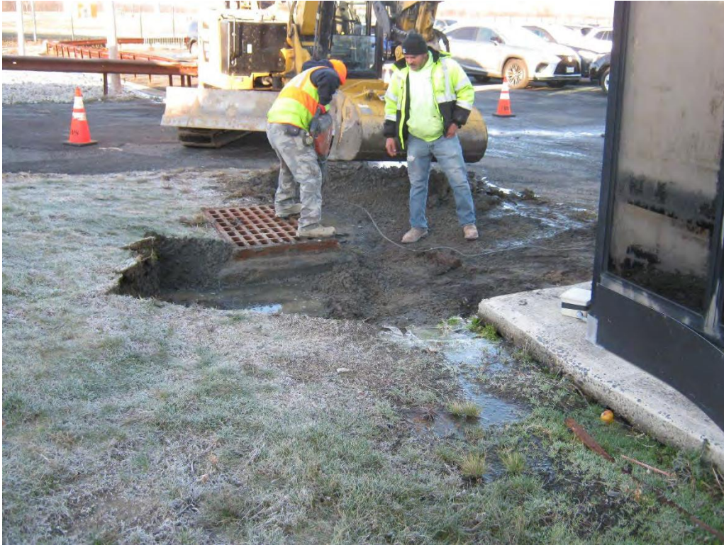
Photo 1 – 7016.1 Area of installation prior to excavation.
