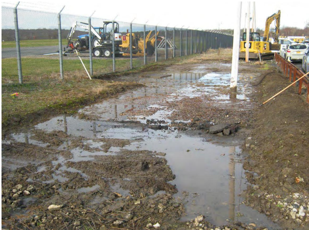
Photo 6 – 7014.2 Post excavation and contouring
