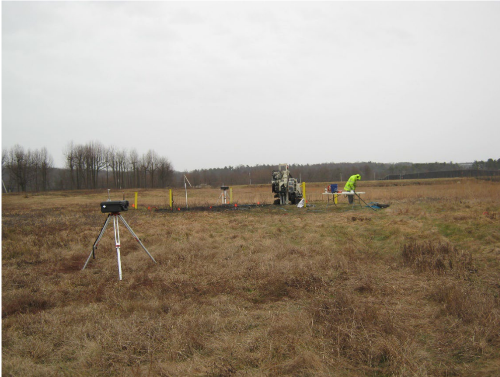
Photo 3 – Injection setup with flags marking injection locations.
