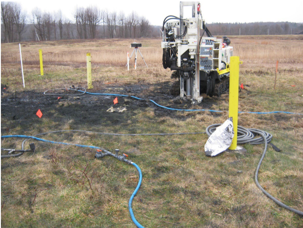
Photo 2 – Drill rig, hose layout and injection area with dust monitoring in background.
