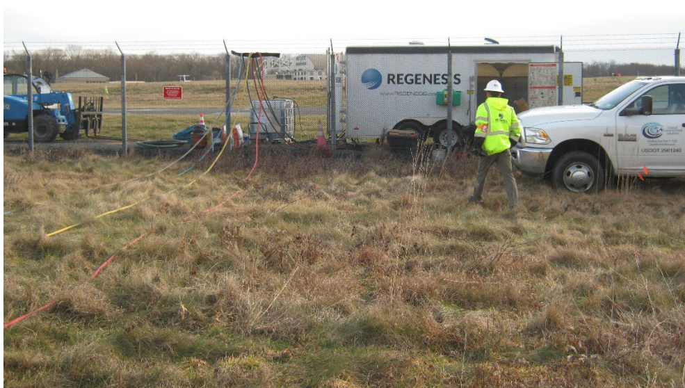
Photo 4 – Injection trailer and hose layout.
