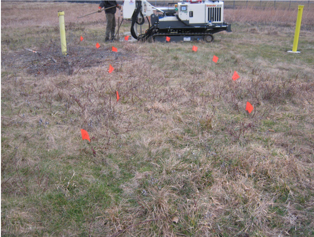
Photo 1 – Injection points as laid out.
