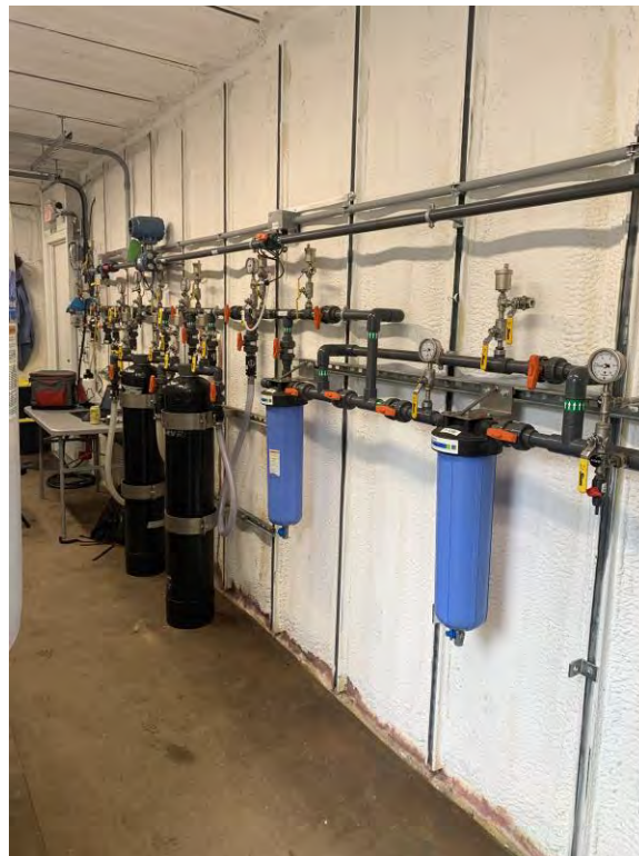
Figure 4 - Example of Similar Containerized FRP Vessel System
