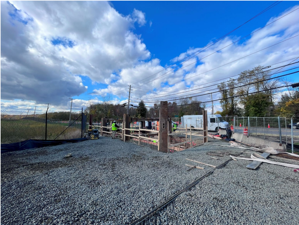
Photo 2 – Taken 11/1/23. Surrounding area around the vault.
