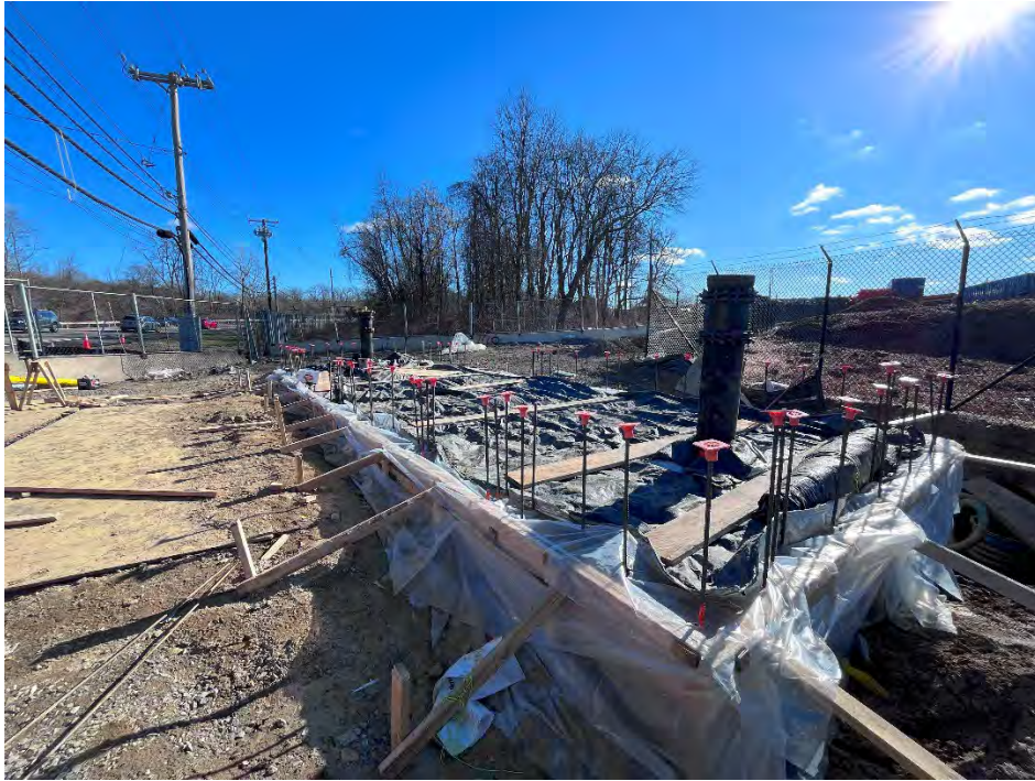
Photo 1 – Progress made as of 1/5/24.
