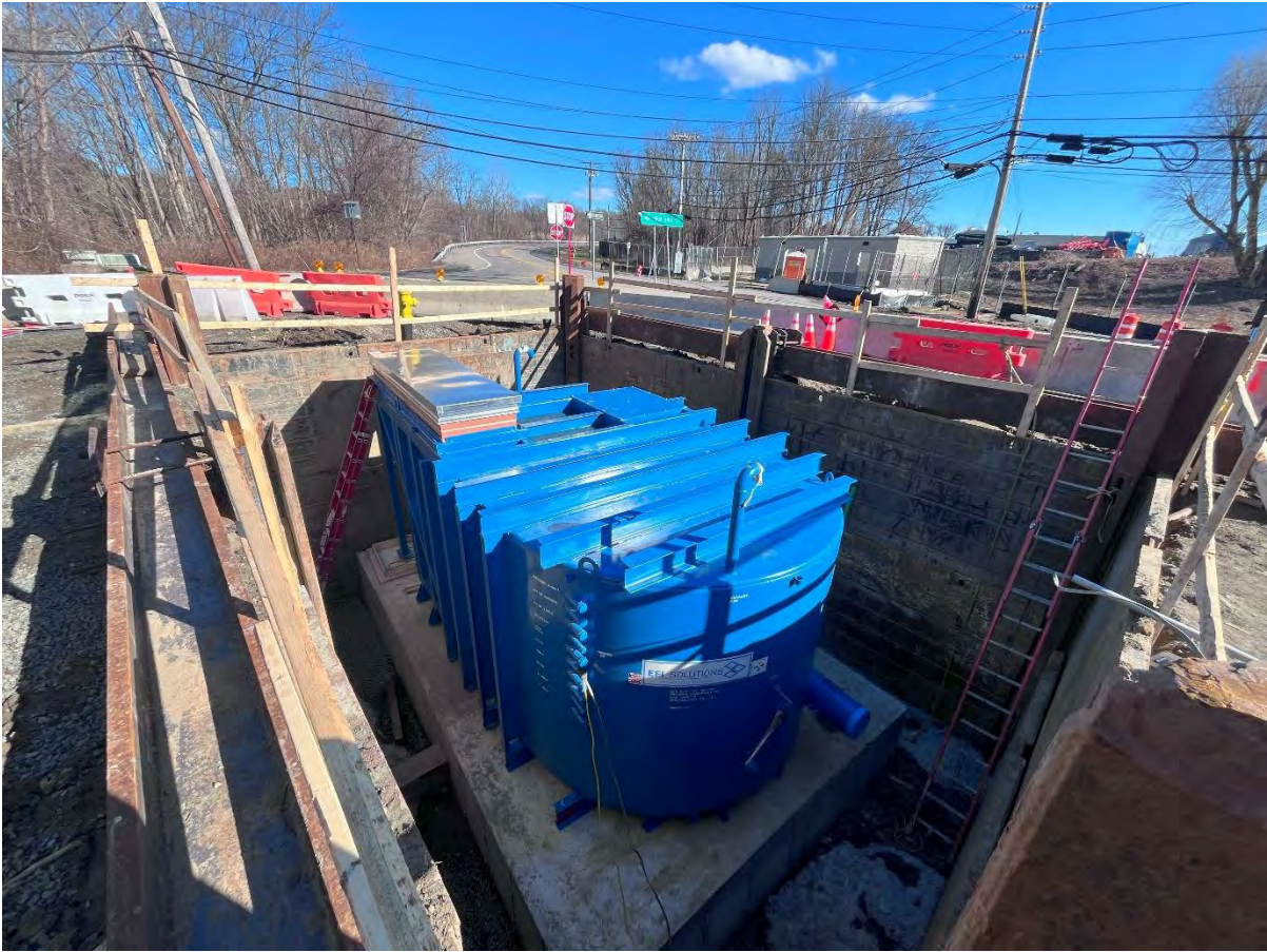
Photo 3 – Taken 2/29/24. The photo shows the newly installed RPZ meter vault on top of the foundation slab. In the background the Airport Road backflow preventer building is also visible.
