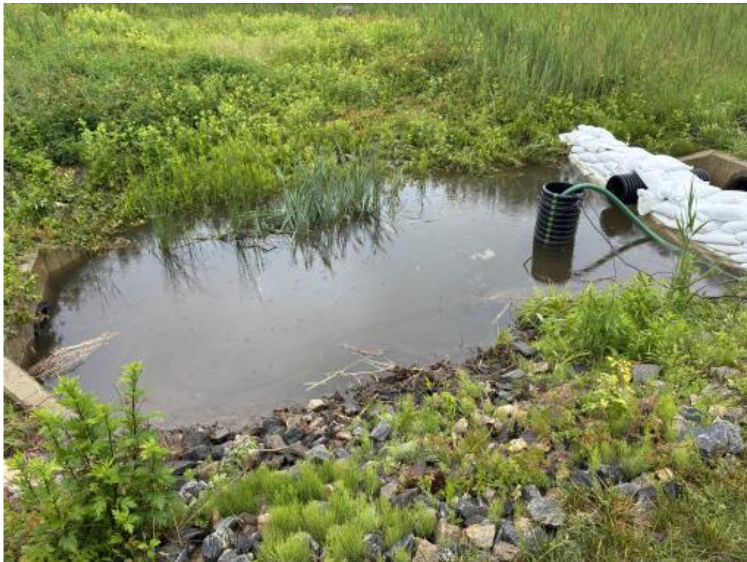
Photo 3: Morning of 5/23/2025, completed weir/OF-7 basin following 0.46" rain event night of 5/22/2025
