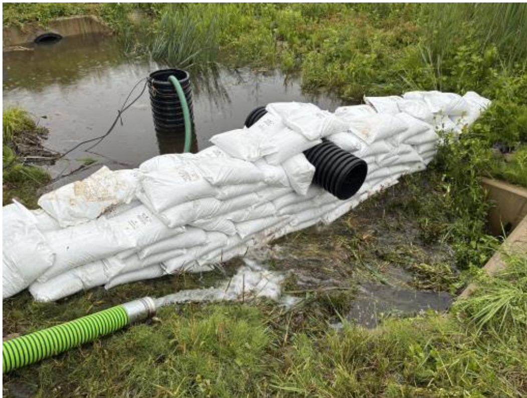
Photo 4: Morning of 5/23/2025, completed weir/OF-7 basin following 0.46" rain event night of 5/22/2025
