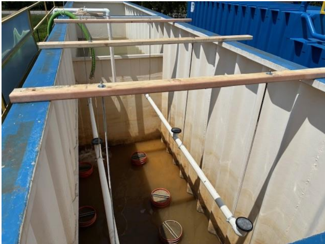
Photo 7: Completion of suspended aeration diffusers in weir tank
