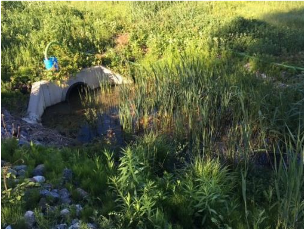
Photo 1: Outfall OF-7 basin prior to site IRM WP site work – 5/19/2024
