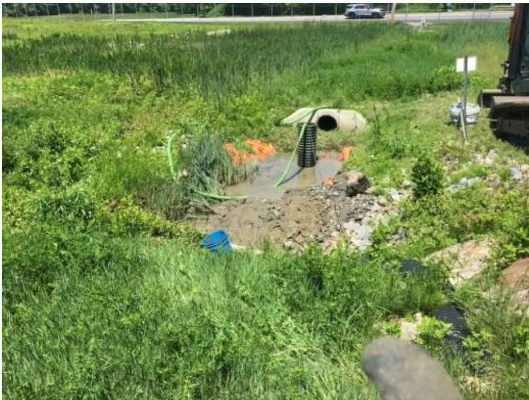
Photo 2: Placement of recovery Sump in OF-7 basin – 5/20/2024
