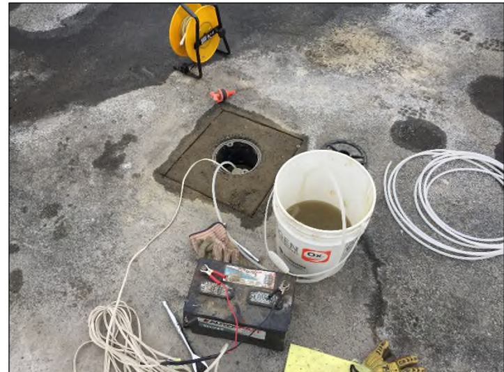
Photograph 4: Development of MW-7.
