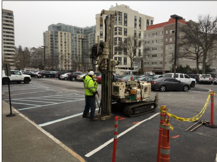
Photograph 1: Installation of soil boring SB-10 with track-mounted Geoprobe 6620DT.
