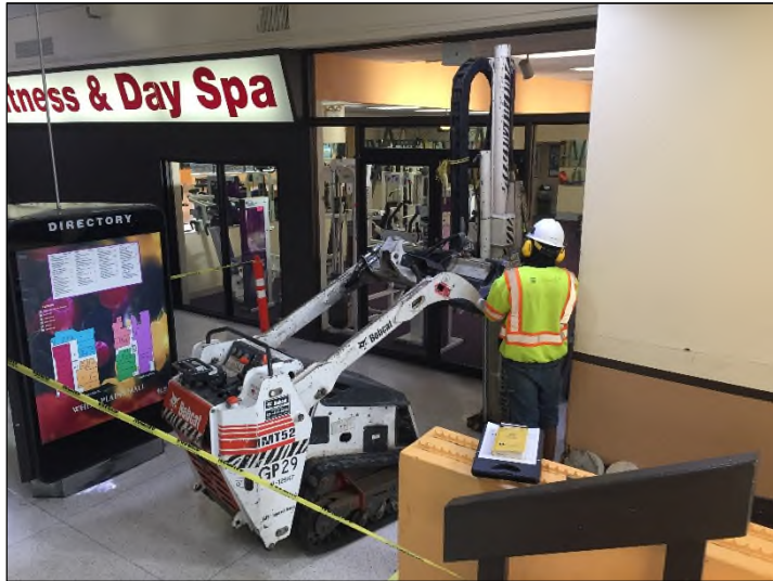
Photograph 5: Installation of soil boring SB-15 with bobcat-mounted Geoprobe 540MT.
