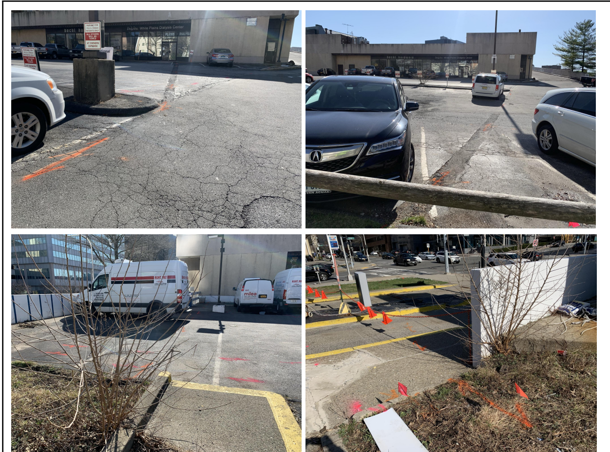
Fig. 3: Images of the two communications trenches detected.
