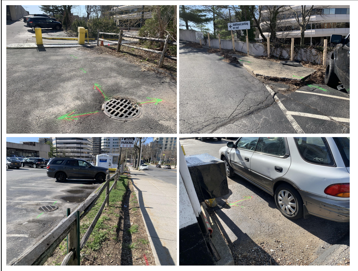
Fig. 4: Images of the storm sewer investigated/detected.
