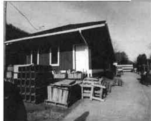
TYPICAL VIEW OF REAR WAREHOUSE
