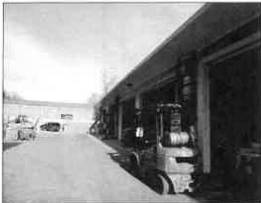
TYPICAL VIEW OF FRONT WAREHOUSE
