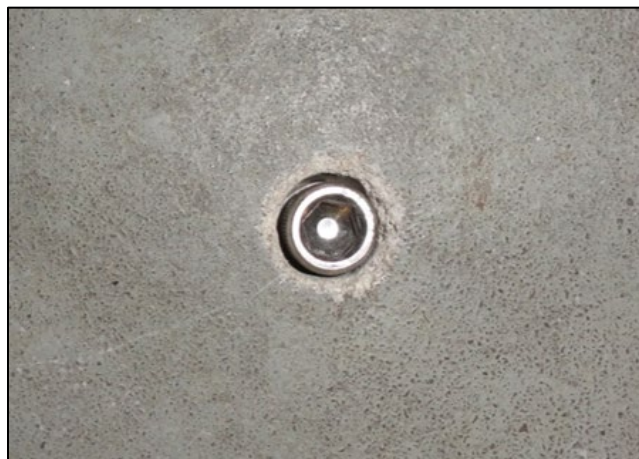
Permanent Floor Test Port
