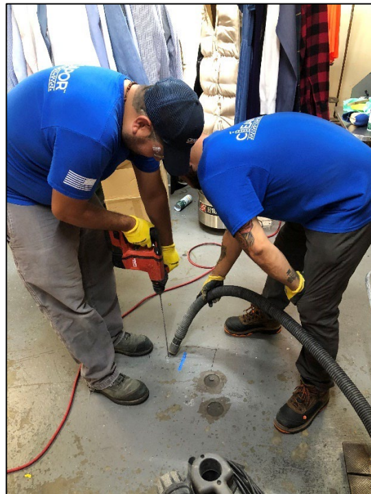
Drilling Quarter-Inch Test Hole with Dust Collection
