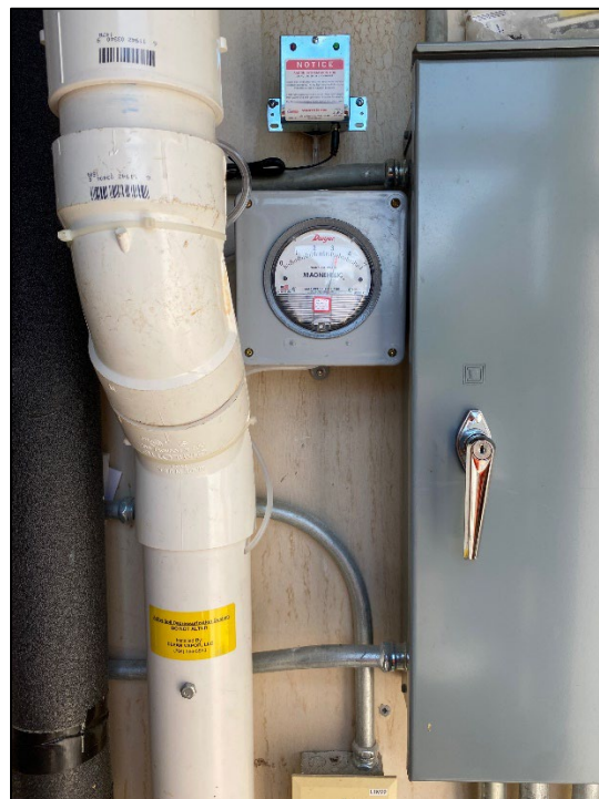
Magnehelic Gauge Enclosure, Riser Test Port with ASD Affixed Label and Checkpoint IIA System Alarm
