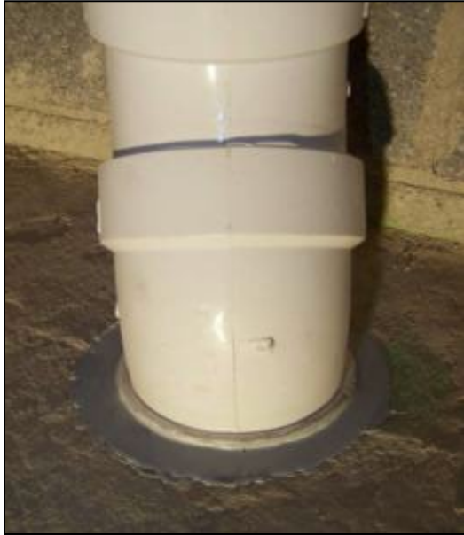
Suction Point Sealing
