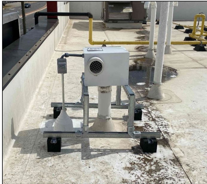
Roof-Mounted AMG Force Blower with Custom Support Frame
