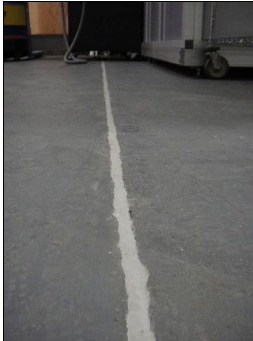
Typical Floor Crack or Expansion Joint Sealing
