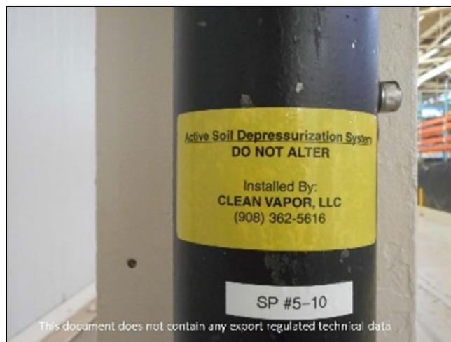
Riser Pipe with System Label, Suction Point # and Sampling Port
