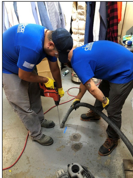
Drilling Quarter-Inch Test Hole with Dust Collection
