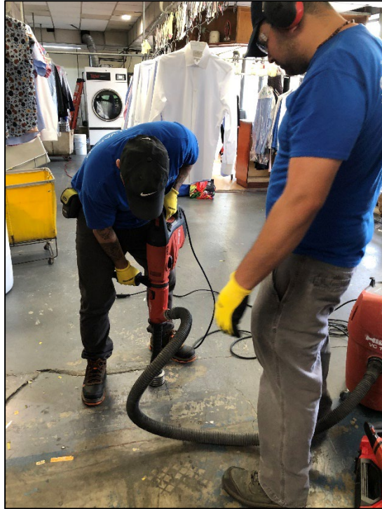
Coring Test Suction Hole with Dust Collection
