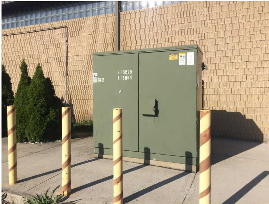
Photo 23: View of one of the pad mounted Con Edison transformers along the eastern exterior of the building (facing west)
