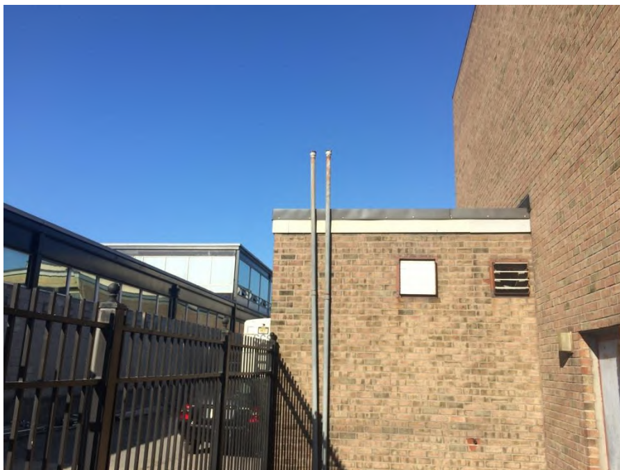
Photo 18: View of tank air vents on the southeastern exterior of the Subject Property (facing west)
