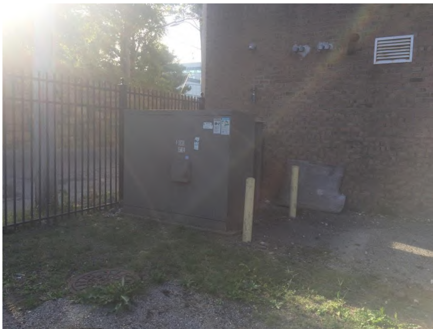
Photo 24: View of a second pad mounted Con Edison transformer located on the southeastern exterior of the Subject Property (facing south)
