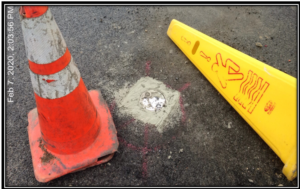
Photograph of a manhole installed for vapor point VP-8
