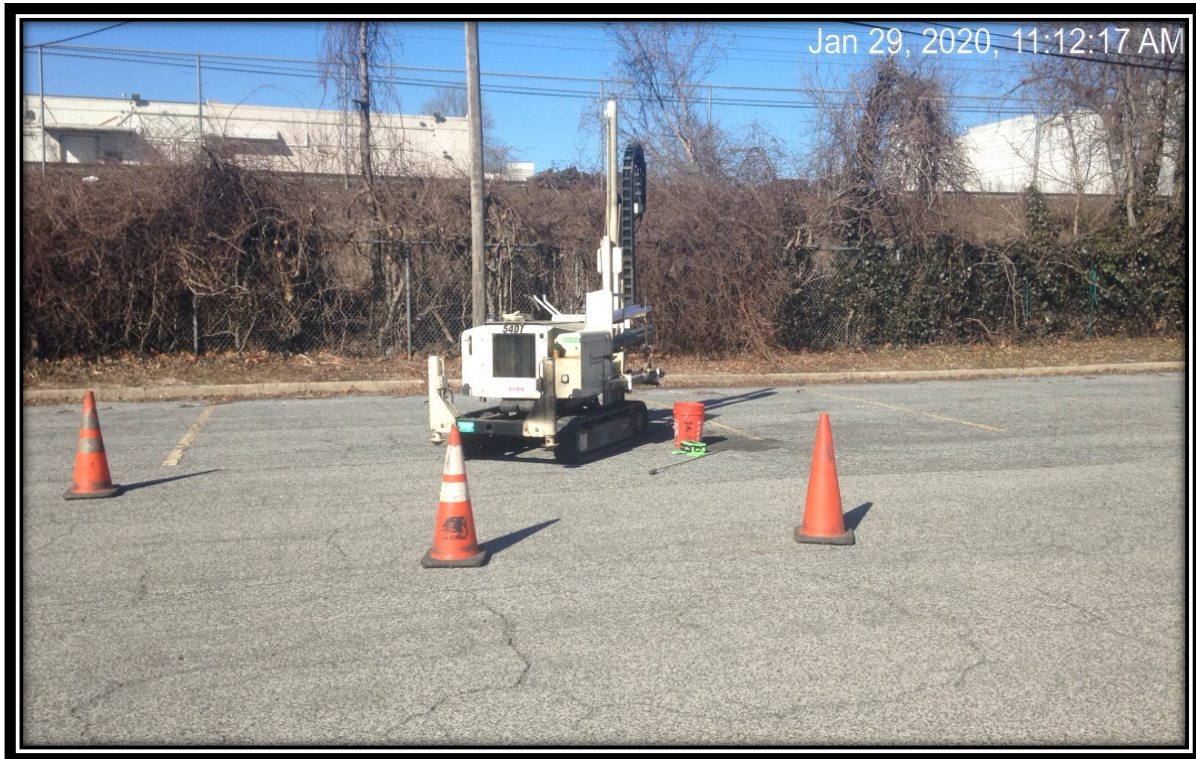
Photograph of GB-8 soil boring being installed on site
