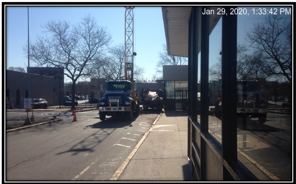
Photograph of Monitor Well MW-1 being installed on-site
