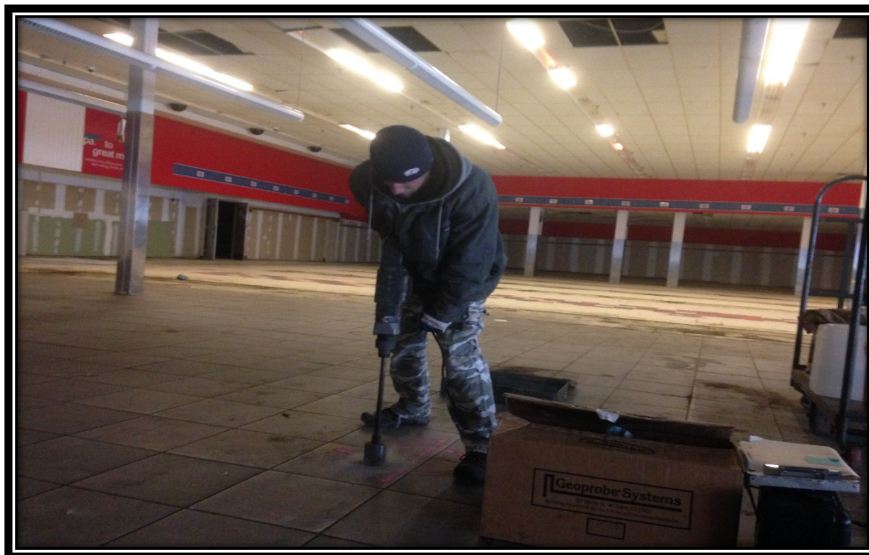
Photograph of soil boring GB-12 being installed by hammering through the interior slab
