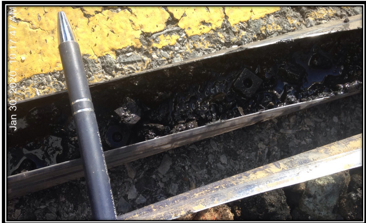
Photograph of visible nuts and bolts found in a macro sampler core during soil boring activities, GB-10
