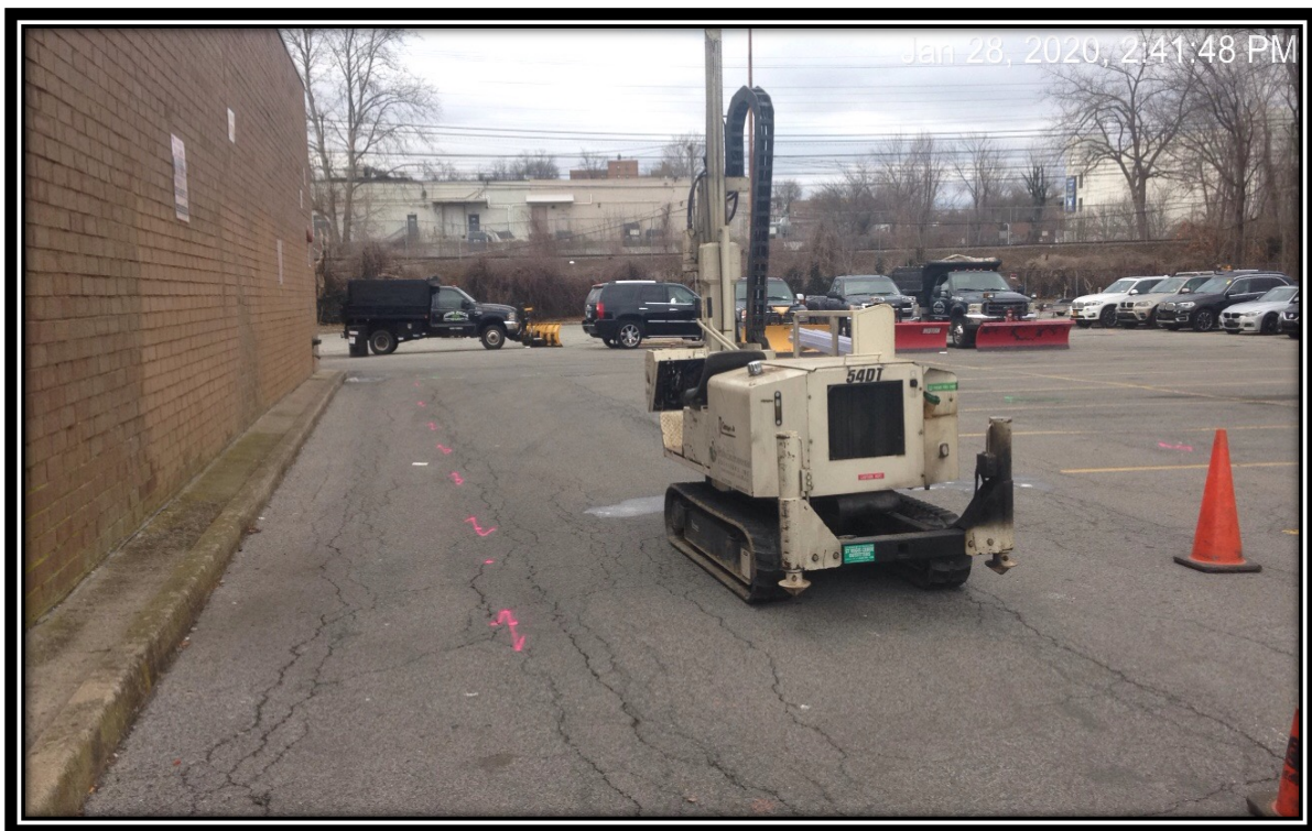
Photograph of soil boring installation activities at GB-6
