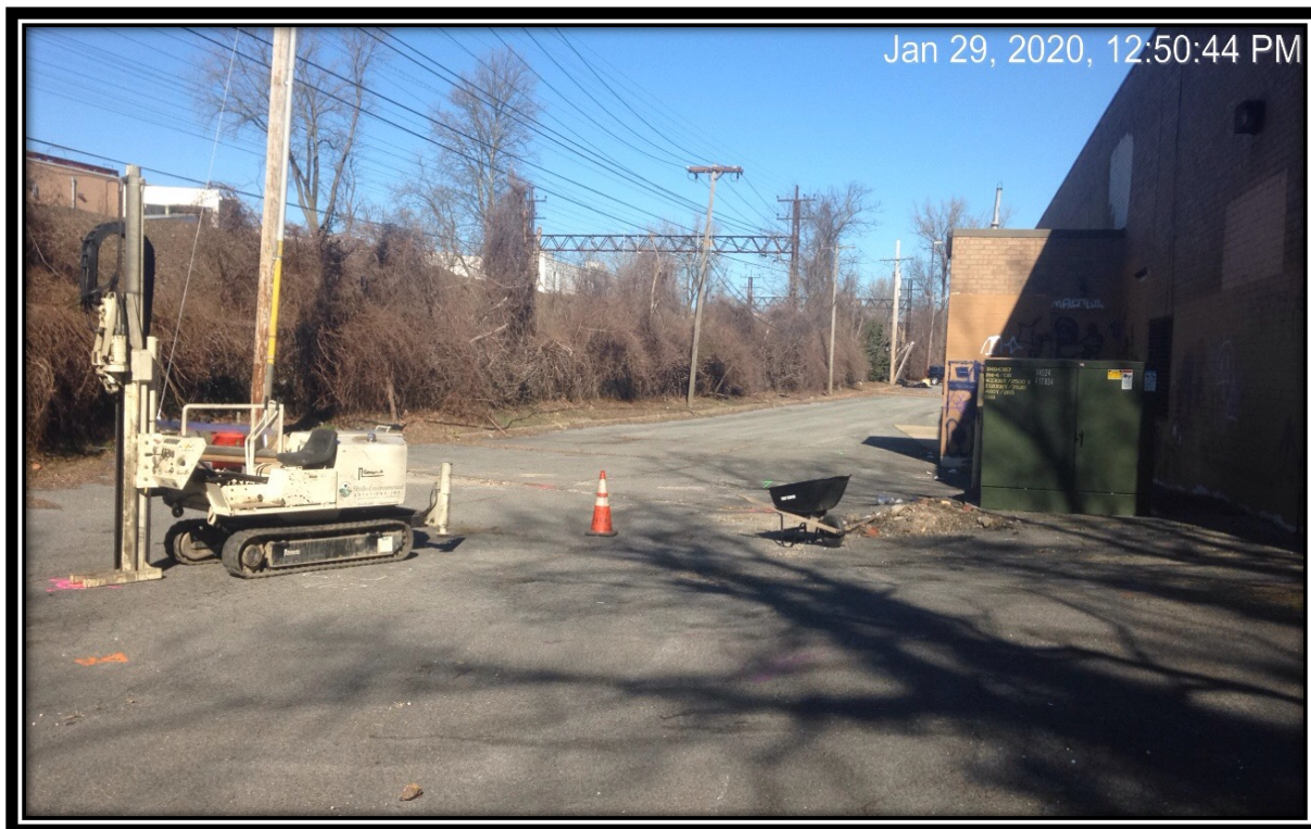
Photograph of soil boring GB-10 being installed
