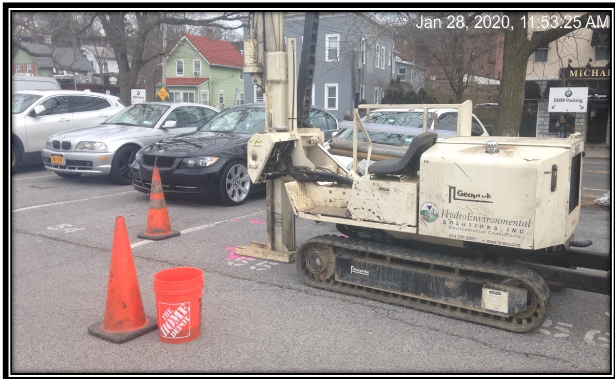
Photograph of Geoprobe® 54DT at GB-5
