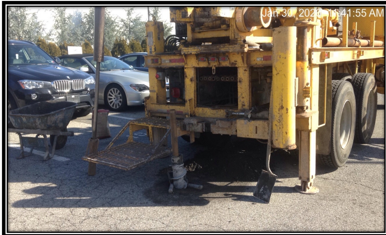
Photograph of Monitor Well MW- 4 being installed using a hallow-stem auger
