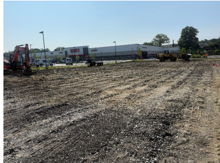
Photo 6. Asphaled Milled Areas (08/15/2025)
