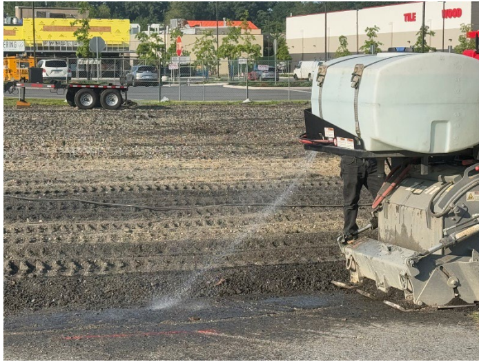
Photo 5. Pre-Wetting of Asphalt (08/15/2025)
