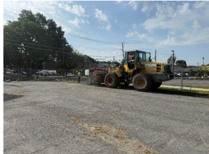
Photo 2. Milling of Asphalt (08/13/2025)
