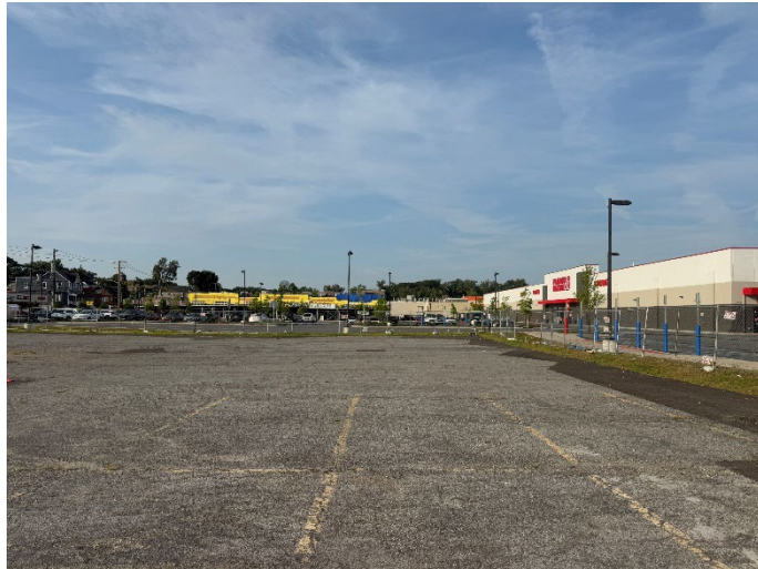
Photo 1. Pre Asphalt Milling Site Condition (08/13/2025)
