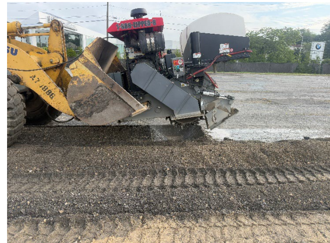
Photo 4. Milling of Asphalt (08/14/2025)
