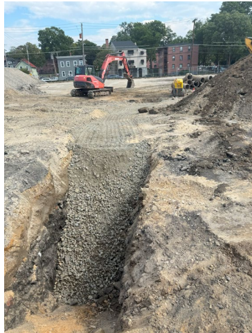
Photo 3. Old Utility Trench (08/29/2025)
