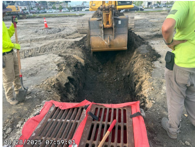
Photo 1. Excavating Old Utility Lines (08/28/2025)
