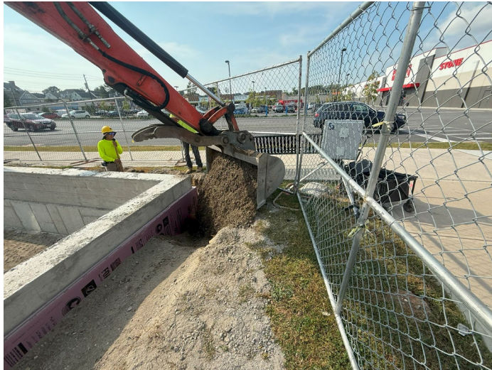
Photo 3. Backfilling (09/23/2025)
