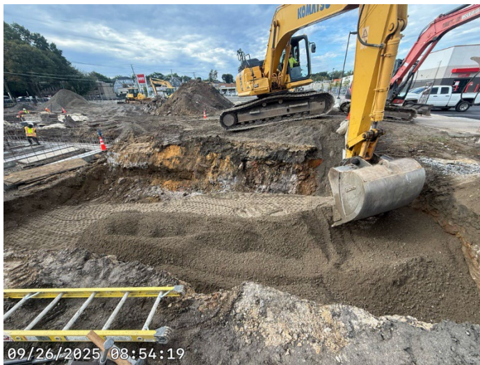
Photo 7. Backfilling (09/26/2025)
