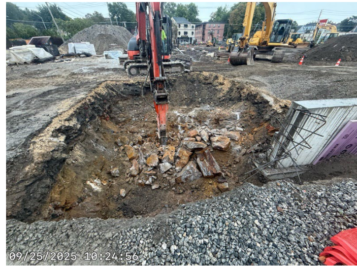
Photo 6. Breaking up Concrete(09/25/2025)
