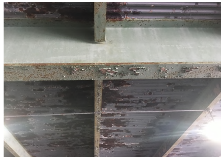
Photograph 4. Suspect peeling and chipping lead-based paint located beneath the upper-level parking deck.
