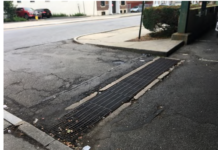
Photograph 2. View of trench drain at the Church Street entrance.
