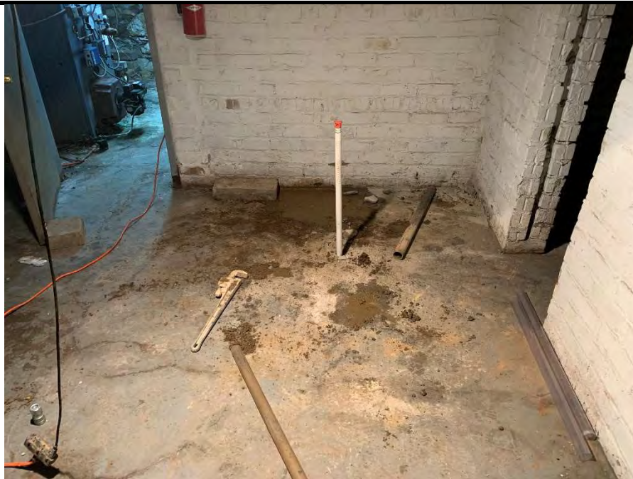
Photo 4: Photograph of monitoring well installation at 12 Church Street.
