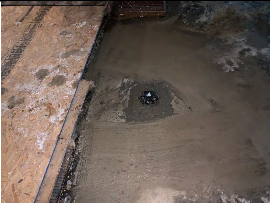
Photo 4: Photograph depicts a completed monitoring well.
