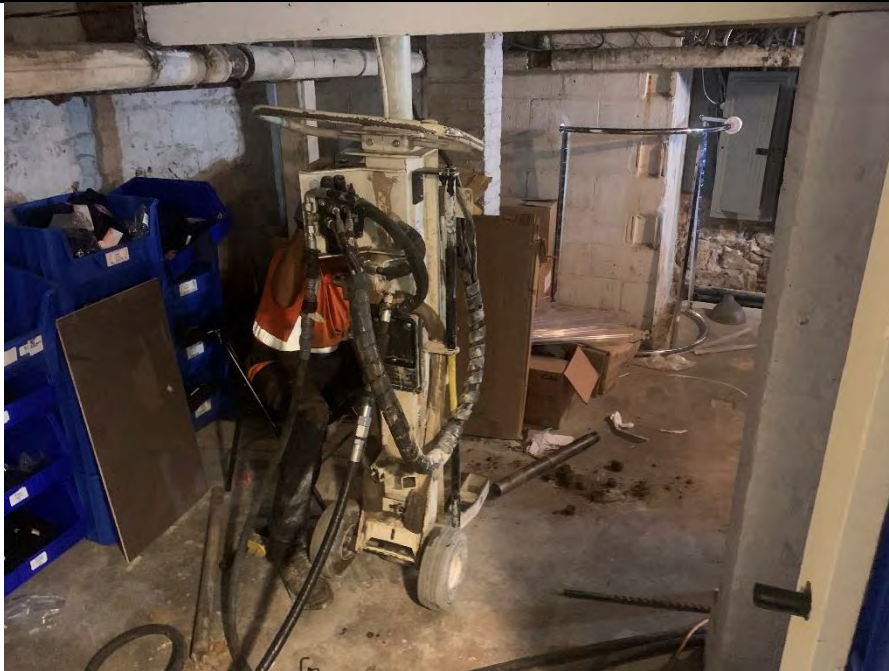
Photo 4: Photograph of direct push activities at boring SB-5.
