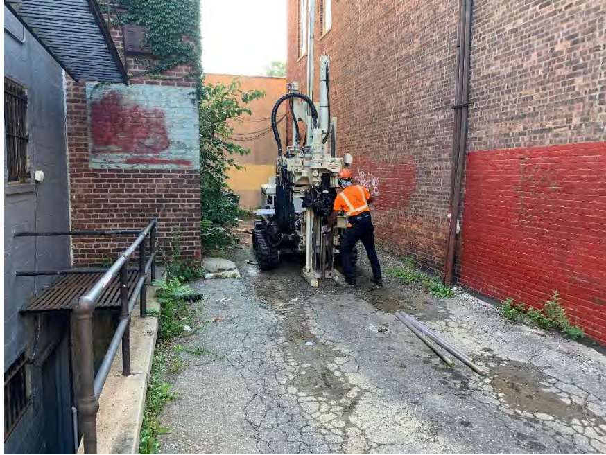
Photo 1: Photograph of drilling activities in the alley north of 12 Church.
