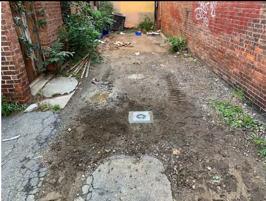
Photo 2: Completed flush mount of MW-4.
