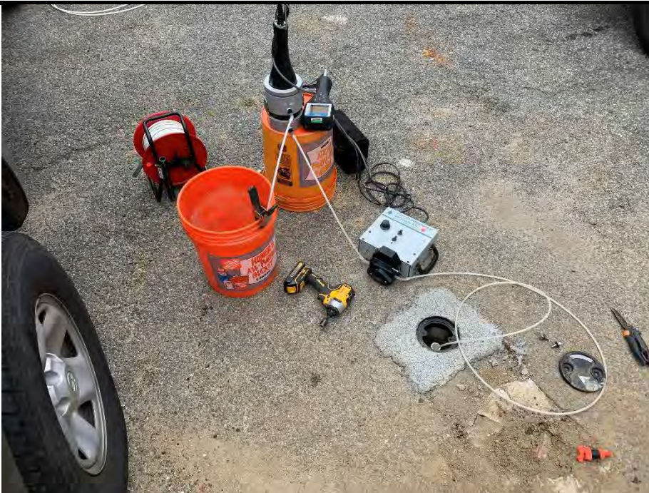
Photo 2: Photograph of low flow sampling at MW-1.
