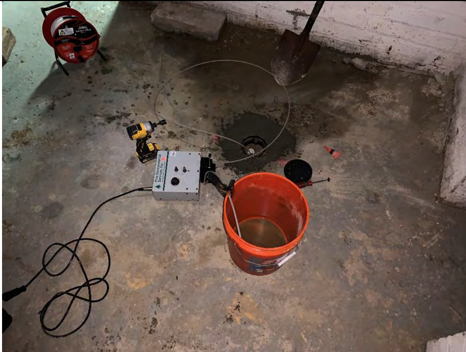
Photo 1: Photograph of development of MW-8.
