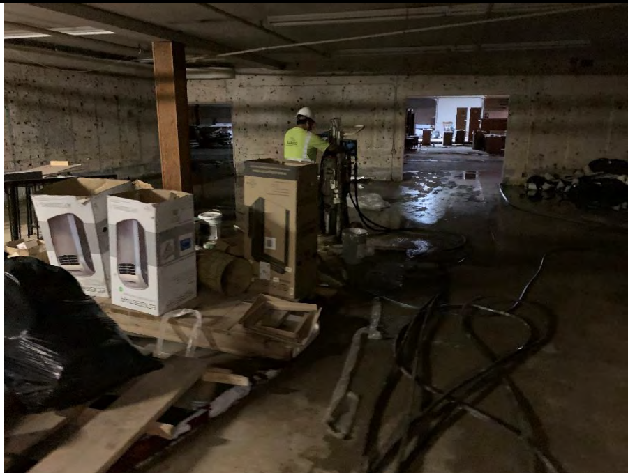
Photo 2: Photograph taken during the drilling of MW-5.
