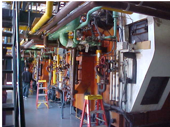
Photo #12: Central heating plant — three No. 6 fuel oil-fired steam boilers
