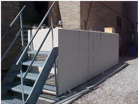
Photo #11: Rear of the central heating plant — 2,000-gallon diesel fuel AST
