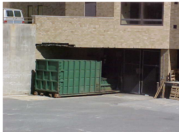
Photo #6: Hydraulic trash compactor servicing the hospital building at the Project
