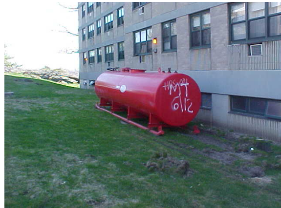
Photo #24: Rear of the apartment building — temporary 2,000-gallon fuel oil AST
