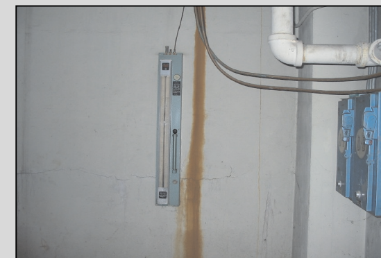
Photograph 18: Former Underground Storage Tank Level Gauge
