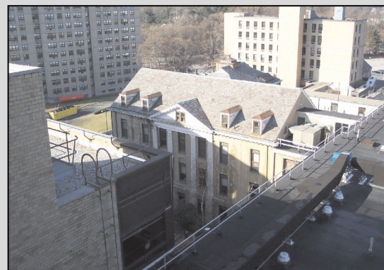
Photograph 5: Original Section of Hospital
