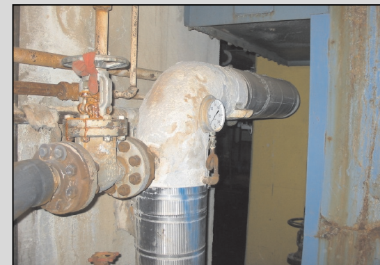
Photograph 21: Location of 10,000-gallon Abandoned-in-Place UST
