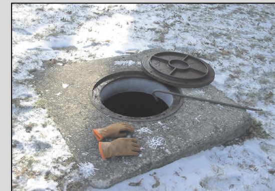
Photograph 16: Man Way Access to Tank
