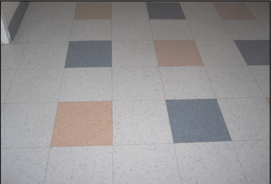
Photograph 9: Typical 12" by 12" Floor Tile Located Throughout Hospital
