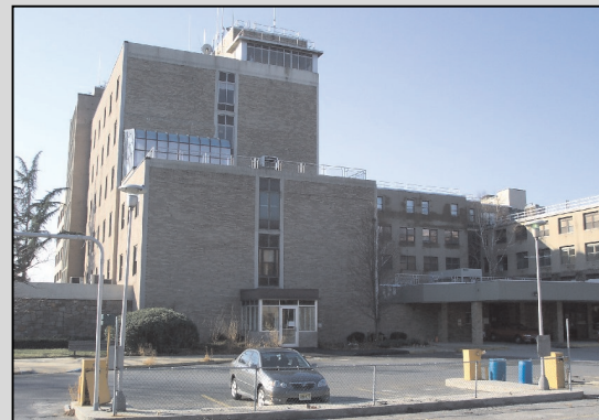
Photograph 1: Northeast Section of Hospital, Emergency Room Entrance
