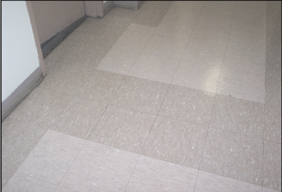
Photograph 10: Typical 12" by 12" Floor Tile Located Throughout Apartment Building
