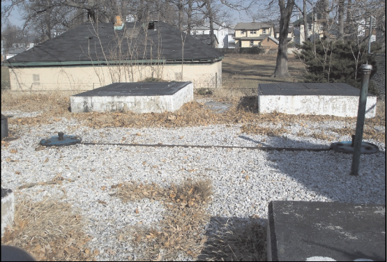
Photograph 13: Area Containing Two 25,000-gallon USTs
