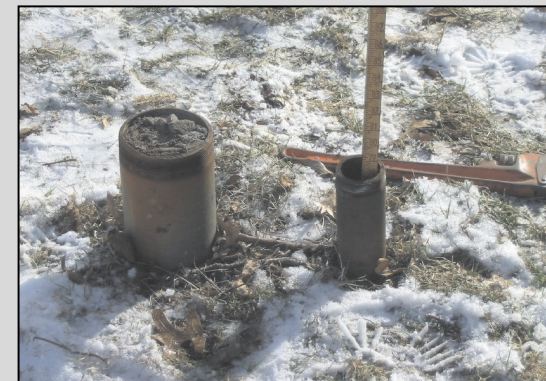
Photograph 15: Concrete-Filled Fill Pipe and Adjacent Tank Entry Pipe
