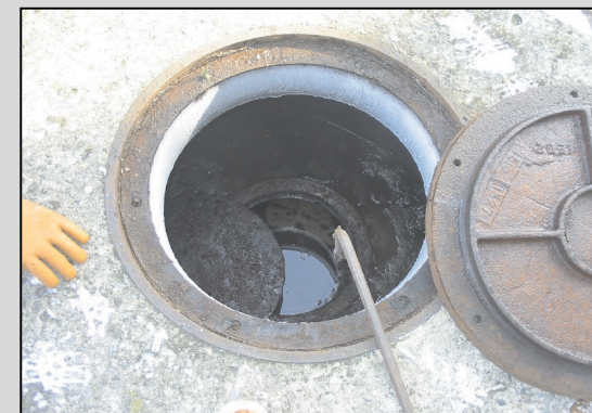
Photograph 17: Inside of Man Way, Concrete Filled
