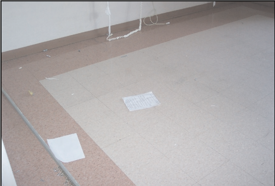
Photograph 8: Typical 12" by 12" Floor Tile Located Throughout Hospital
