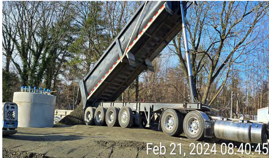
Photograph 1 - Excavation contractor importing Item #4 for use within the antennae COU area, view facing west.
