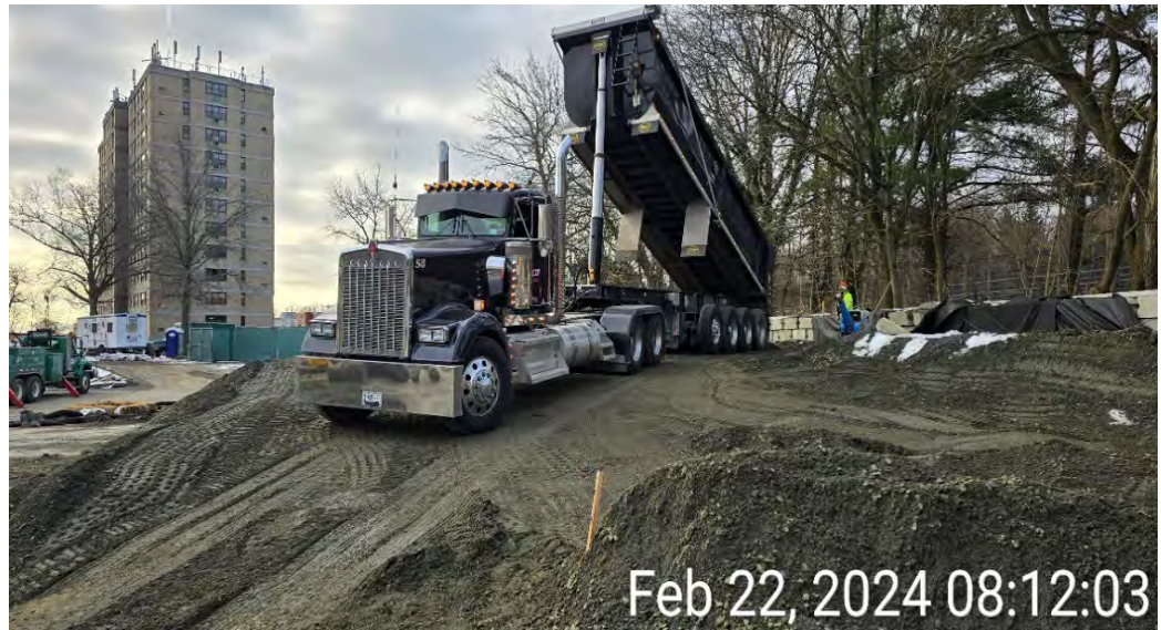
Photograph 1 - Excavation contractor importing Item #4 for use within the antennae COU area, view facing southeast.
