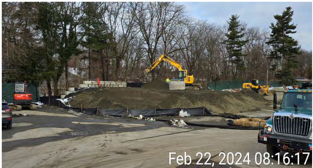
Photograph 2 - Excavation contractor conducting general grading and compaction of Item #4 within the antennae COU area, view facing northwest.
