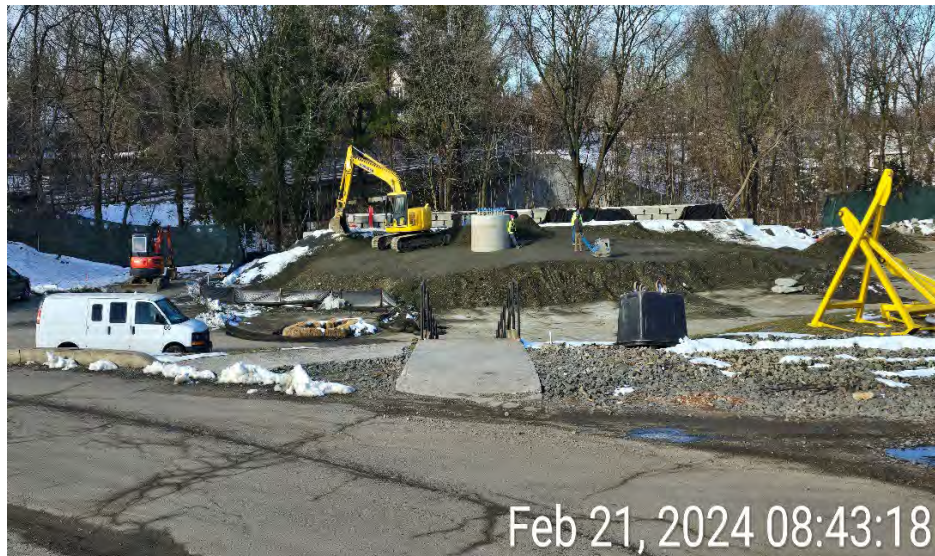
Photograph 2 - Excavation contractor conducting general grading and compacting Item #4 within the antennae COU area, view facing southwest.
