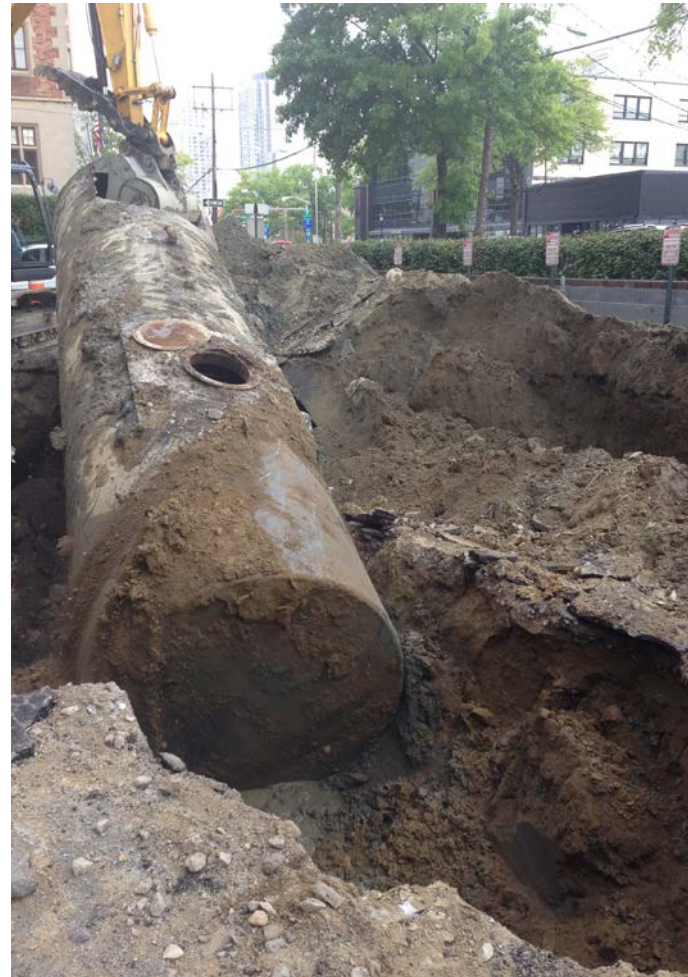
UST BEING REMOVED FROM ITS EXCAVATION
