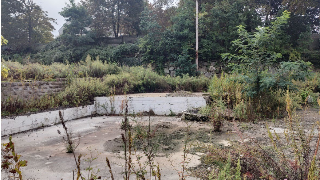
Photo 4 – Expanded view of the elevated concrete pad containing the two detections.
