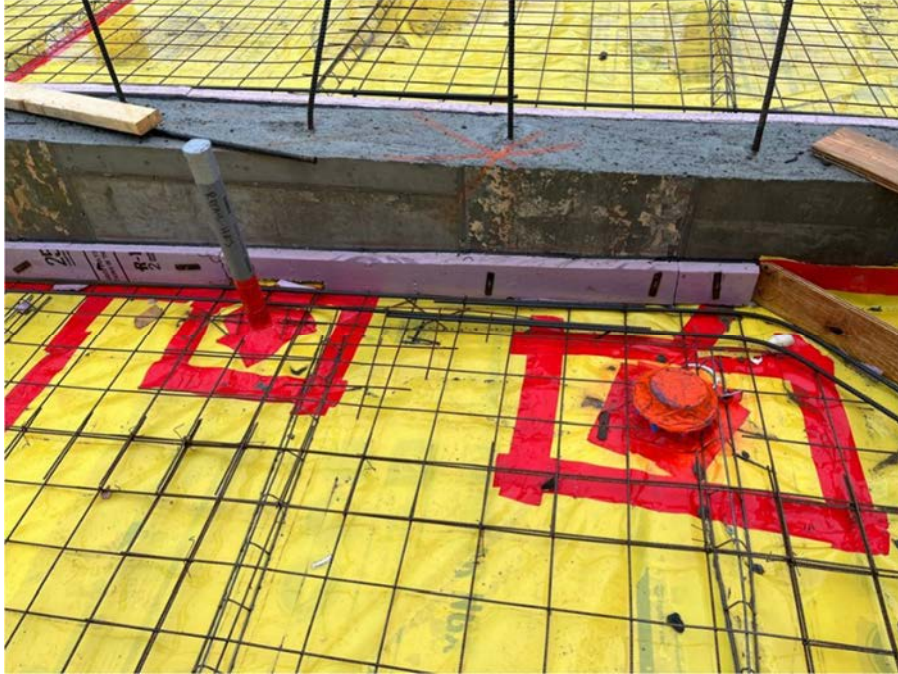
Photo 18: Vapor Barrier Sealed with Tape at Penetrations and Seams.
