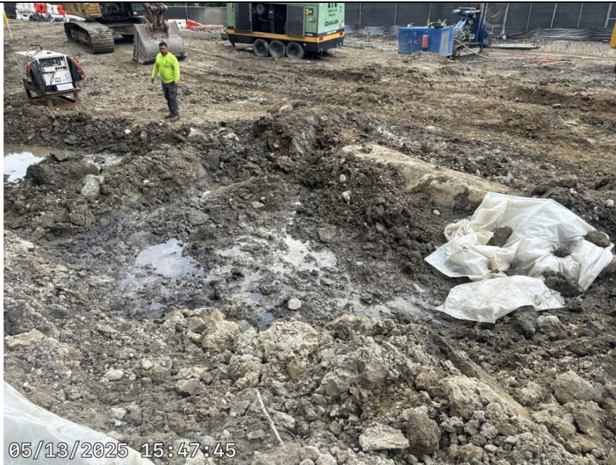
Photo 5: Uncovered Underground Storage Tank (UST).
