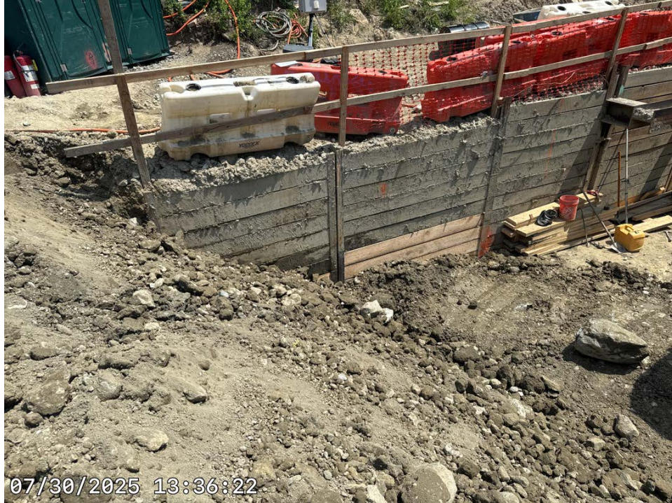
Photo 3: SOE lagging installation.
