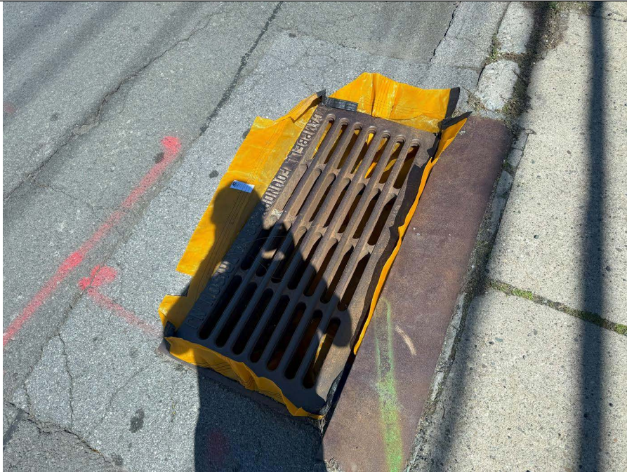
Photo 2: Erosion control installed on stormwater inlet.
