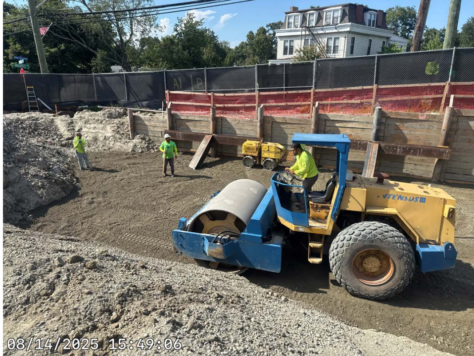
Photo 3: Backfill and compaction
