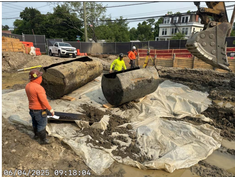
Photo 10: View of UST-2 and UST-3 Encountered and Removed
