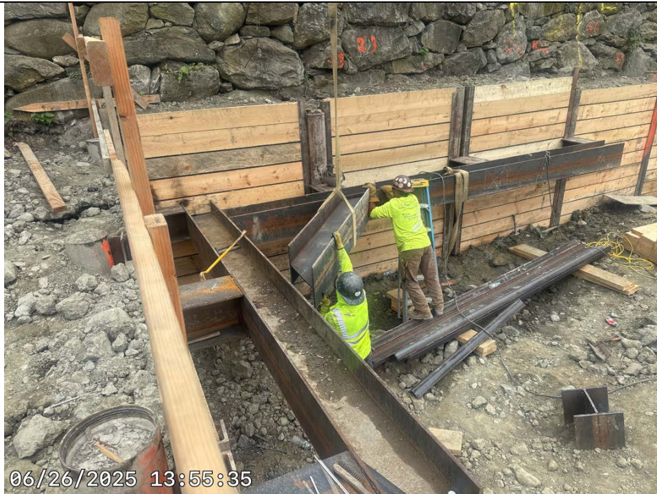
Photo 4: Support of excavation installation.
