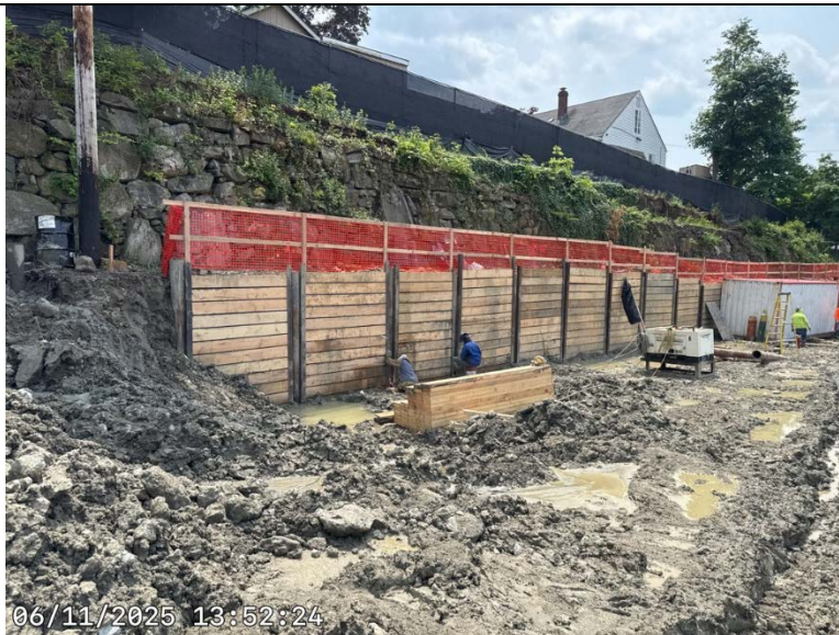
Photo 2: Support of excavation installation.
