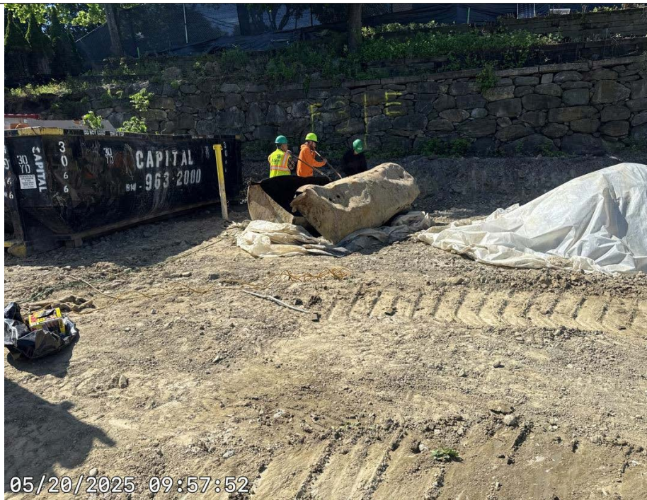
Photo 4: Cleaning and Offsite Disposal of Underground Storage Tank (UST).
