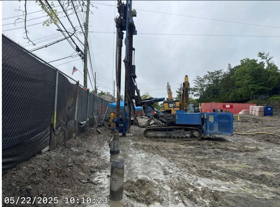
Photo 1: SOE Installation.
