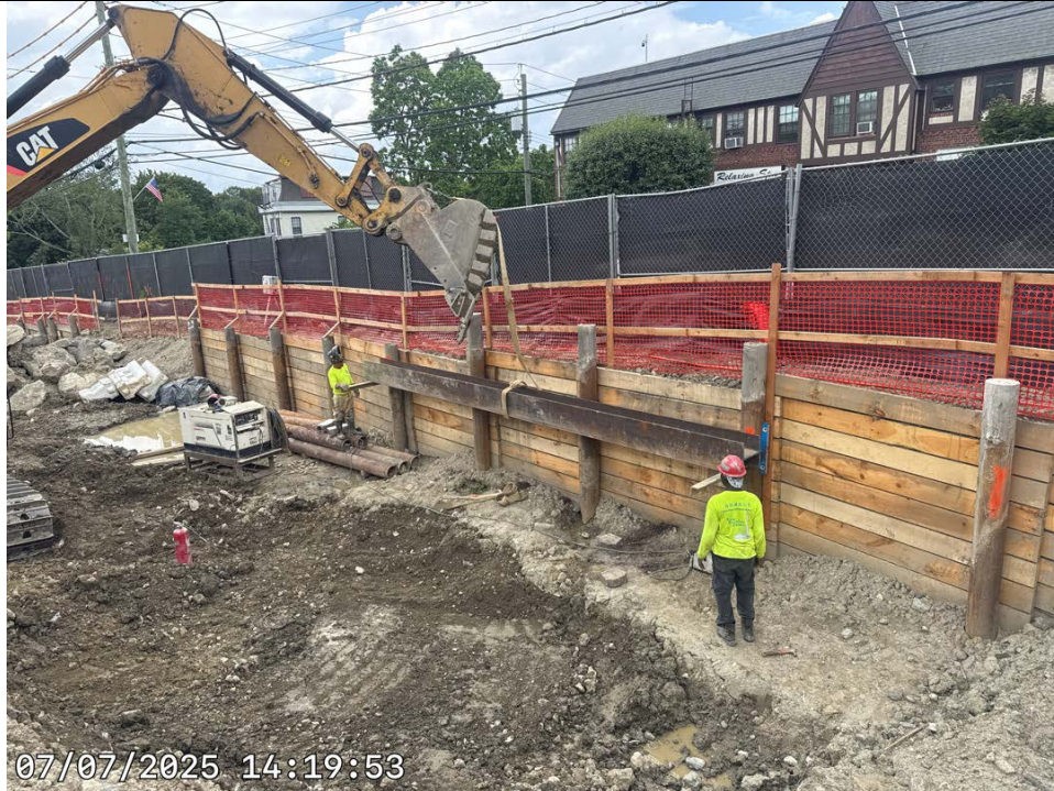
Photo 2: Support of excavation installation.
