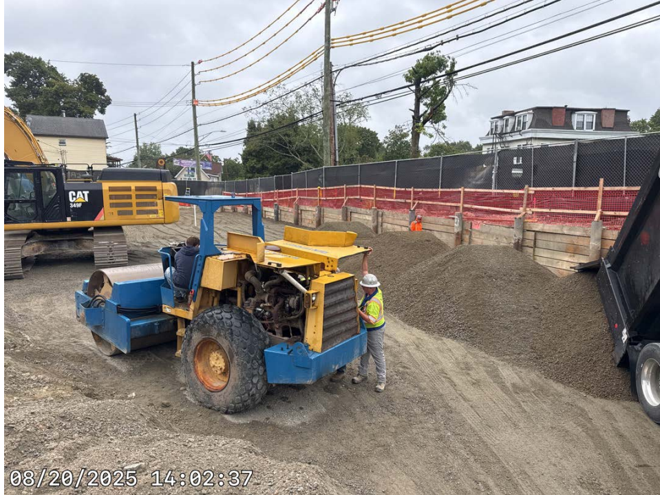
Photo 15: View of Structural Fill Import.
