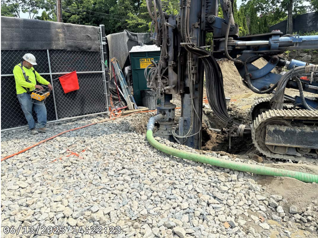
Photo 1: Drilling pile in northeastern portion of the site.
