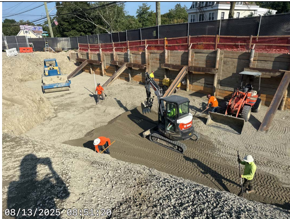
Photo 2: Backfill and compaction
