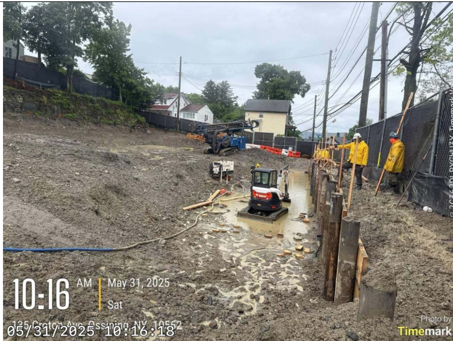
Photo 6: Stormwater Removal from the Northwestern Corner of the Site.
