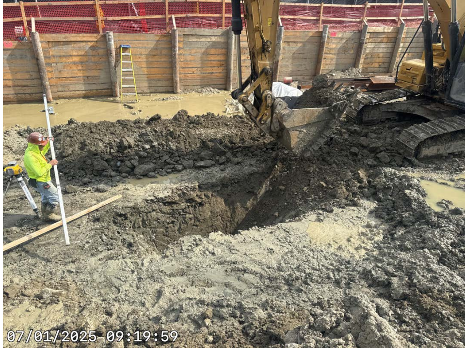
Photo 1: Excavation for soil remediation in northern portion of the Site.
