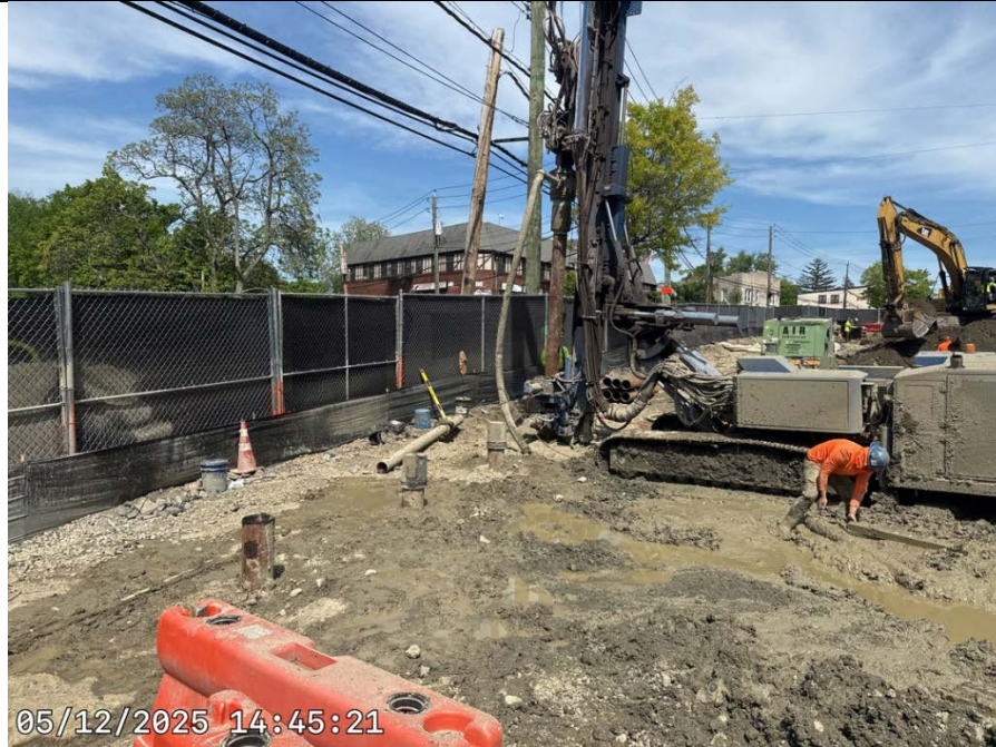
Photo 1: SOE Installation.
