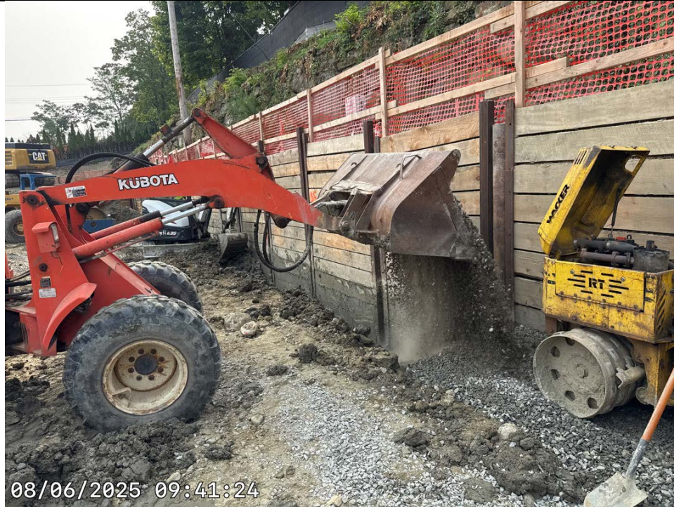
Photo 3: Stone placement for footings.
