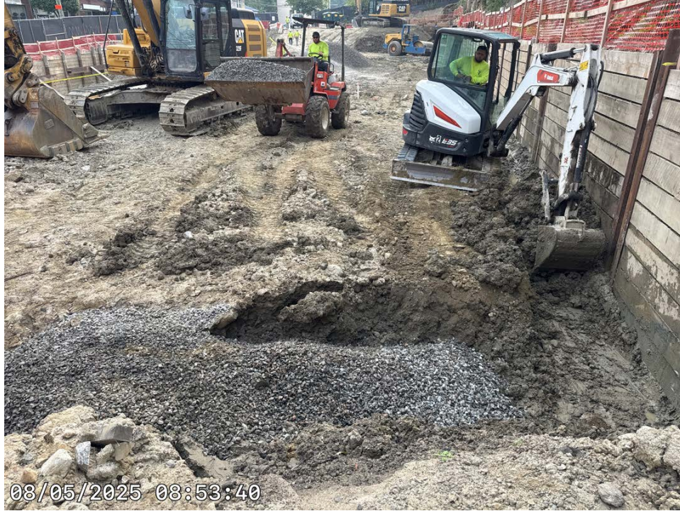
Photo 13: View of Soil Excavation and Footing Excavation.
