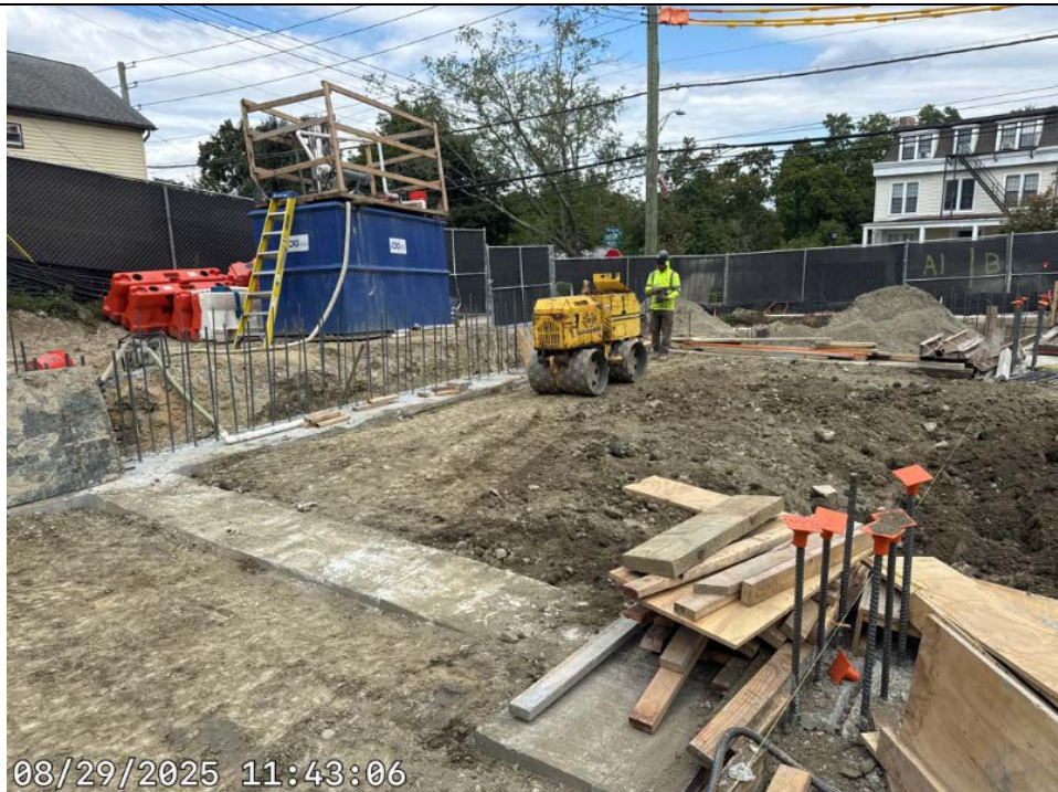
Photo 4: Fill and Compaction
