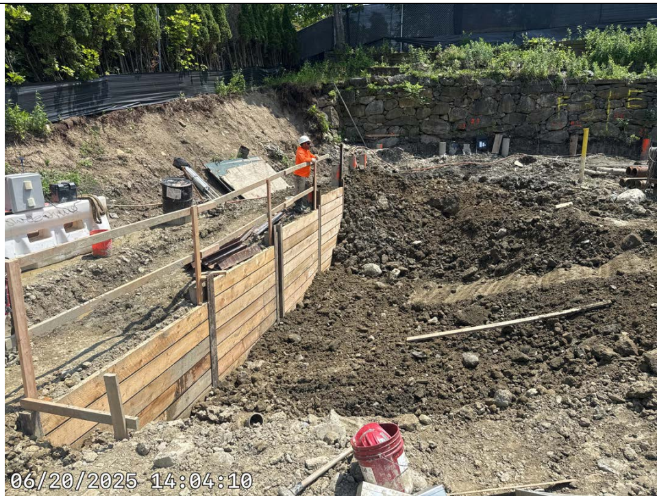
Photo 2: Support of excavation installation.
