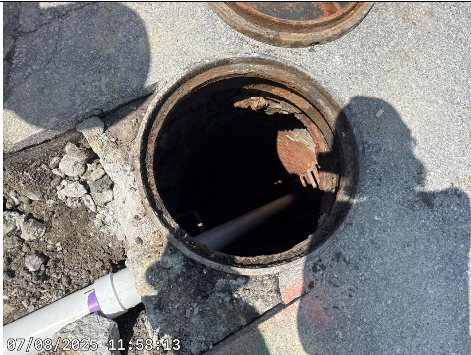
Photo 12: View of Dewatering System Discharge Point to Sanitary Sewer on Croton Avenue.
