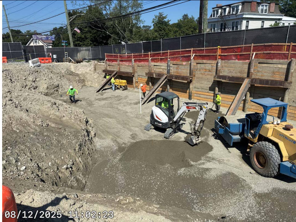
Photo 1: Backfill and compaction
