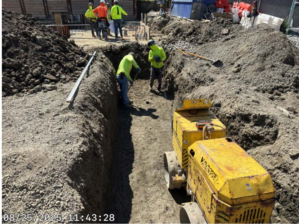
Photo 1: Footing Subgrade
