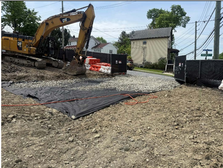
Photo 4: View of Soil Erosion and Sediment Controls – Installation of Construction Entrance
