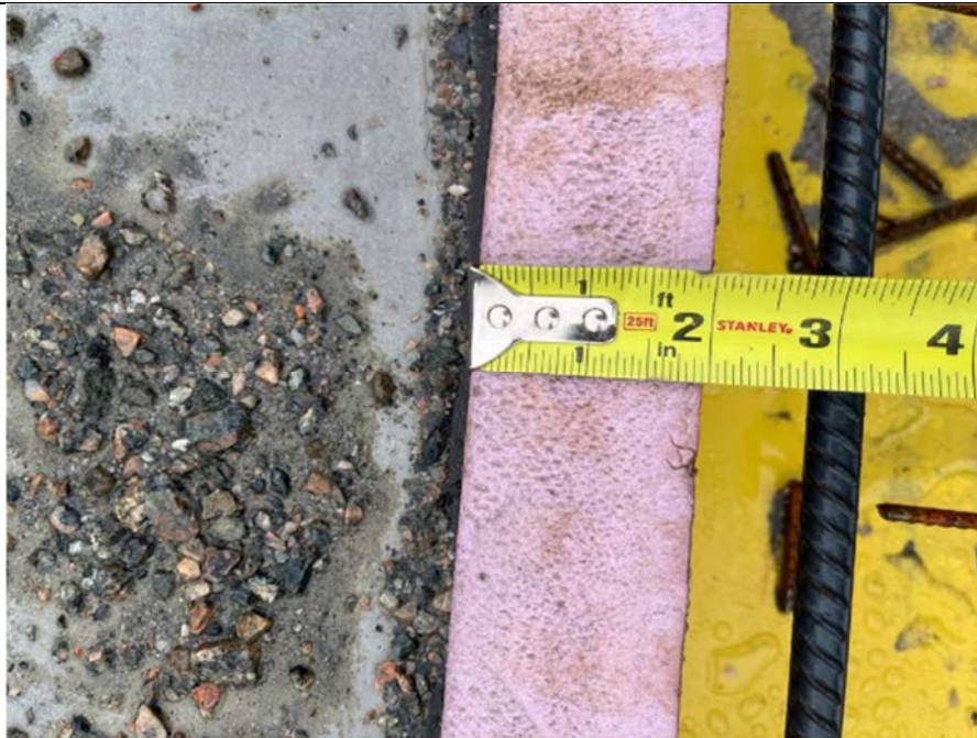
Photo 19: 2" XPS (R-10) Slab on Grade Insulation.
