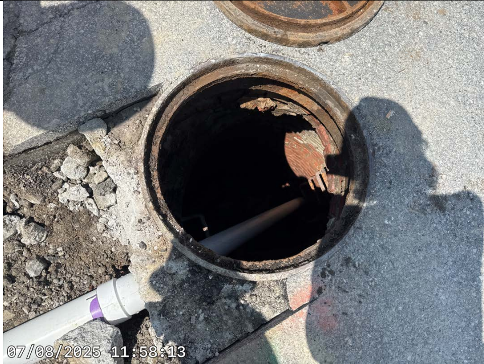
Photo 1: Dewatering system discharge point to sanitary sewer on Croton Avenue prior to pavement restoration.
