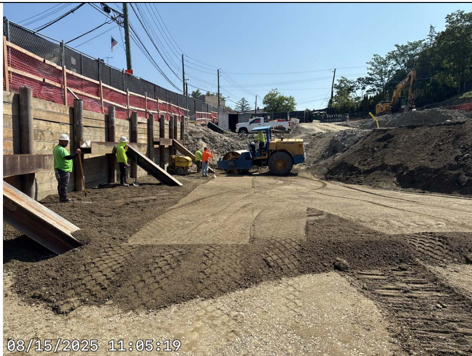
Photo 4: Backfill and compaction
