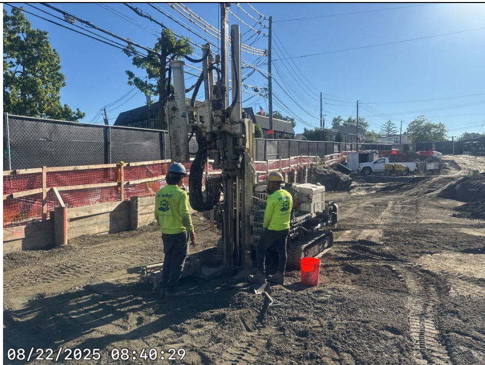
Photo 4: Monitoring Well Installation
