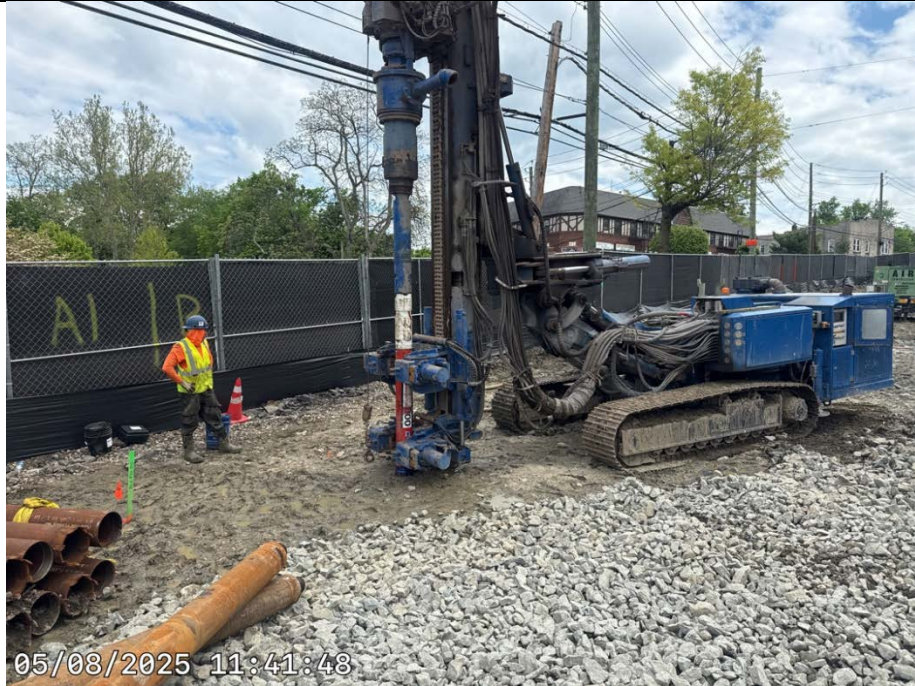
Photo 5: SOE installation.
