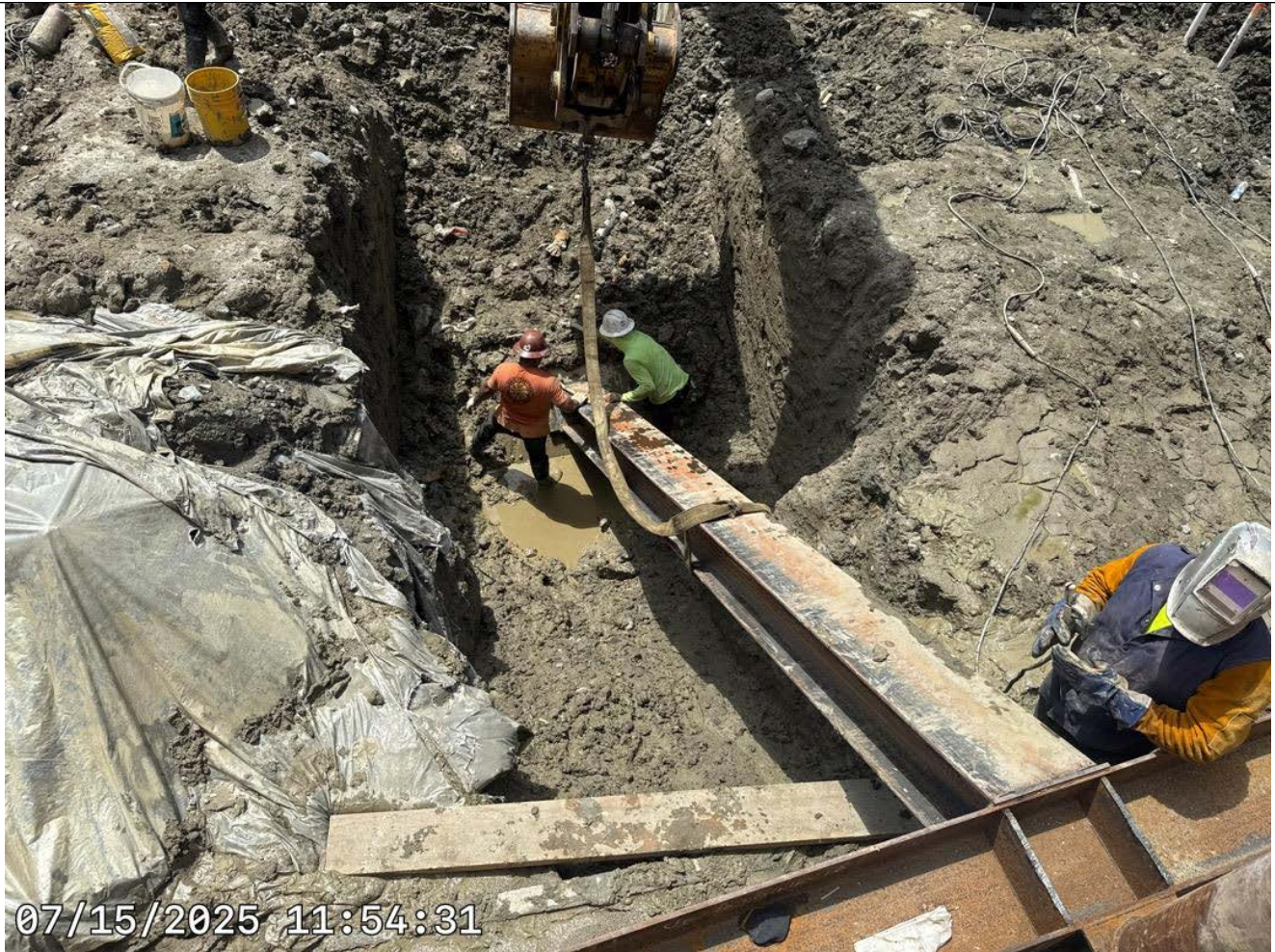
Photo 1: Support of Excavation Installation.
