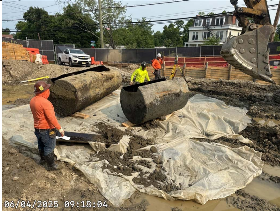
Photo 1: Removal of USTs.
