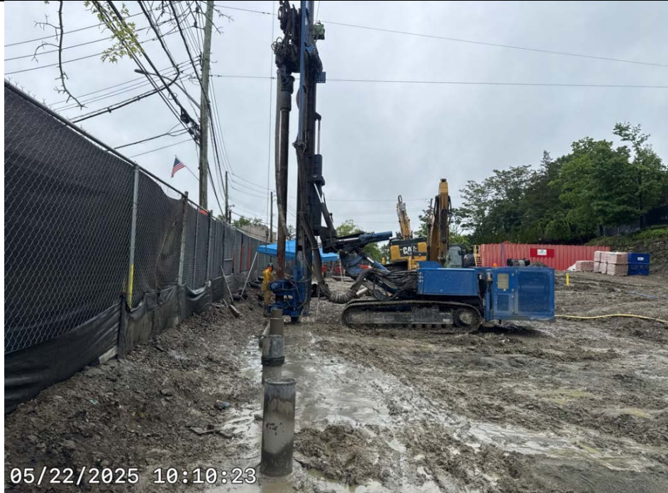
Photo 7: View of Support of Excavation Installation
