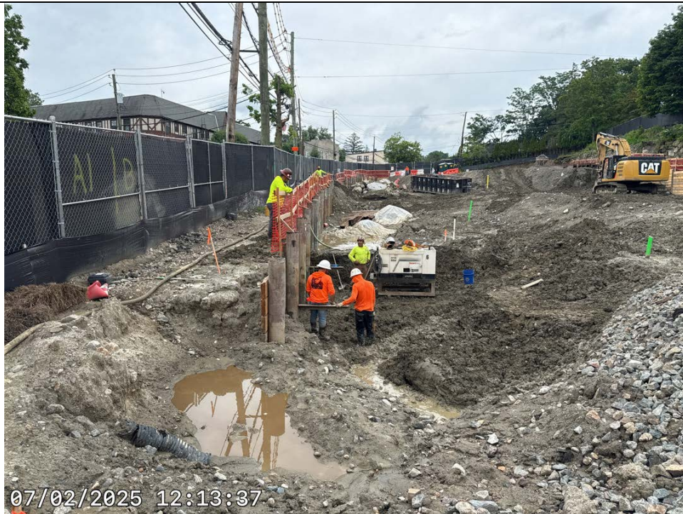
Photo 2: Support of excavation installation.
