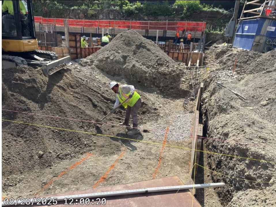
Photo 3: Footing Subgrade
