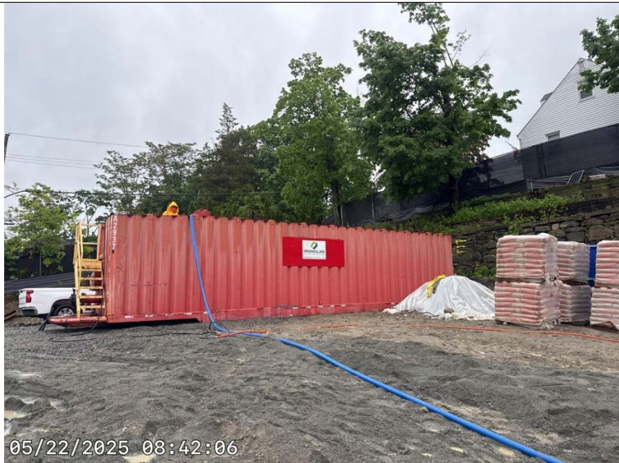
Photo 5: Stormwater Management Frac Tanks in the Southwestern Corner of the Site.
