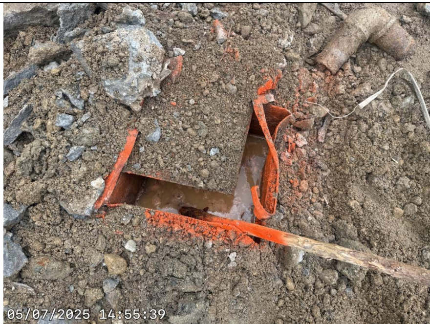
Photo 2: Subsurface grease trap.
