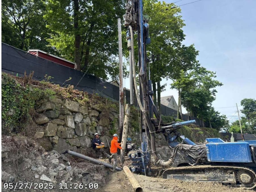
Photo 1: SOE Installation.
