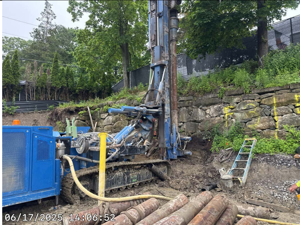
Photo 1: Drilling pile in southern portion of the site.
