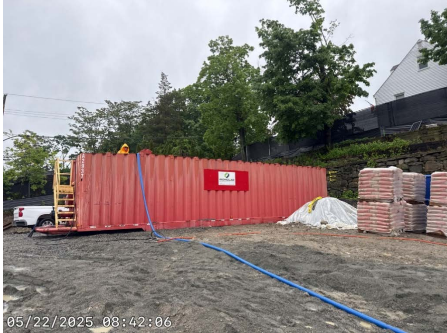
Photo 11: View of Stormwater Management Frac Tanks in the Southwestern Corner of the Site.
