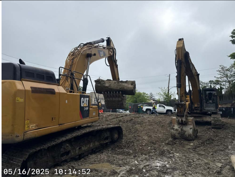
Photo 9: View of UST-1 Encountered and Removed
