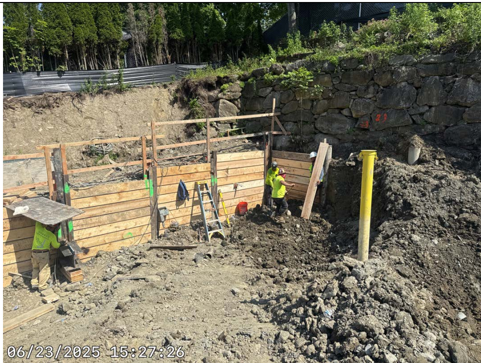
Photo 2: Support of excavation installation.
