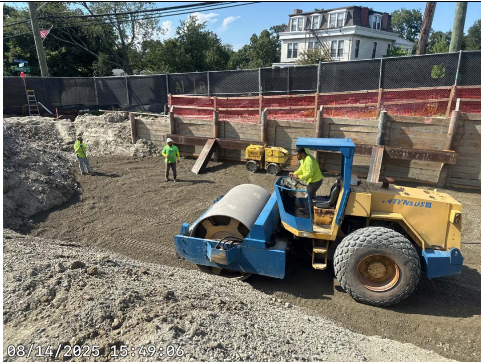
Photo 14: View of Backfill and Compaction.
