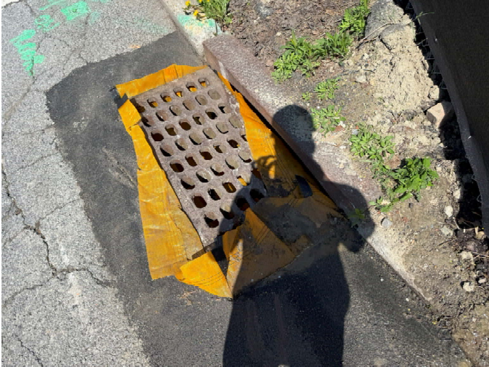
Photo 3: View of Soil Erosion and Sediment Controls – Installation of Storm Drain Inlet Protection
