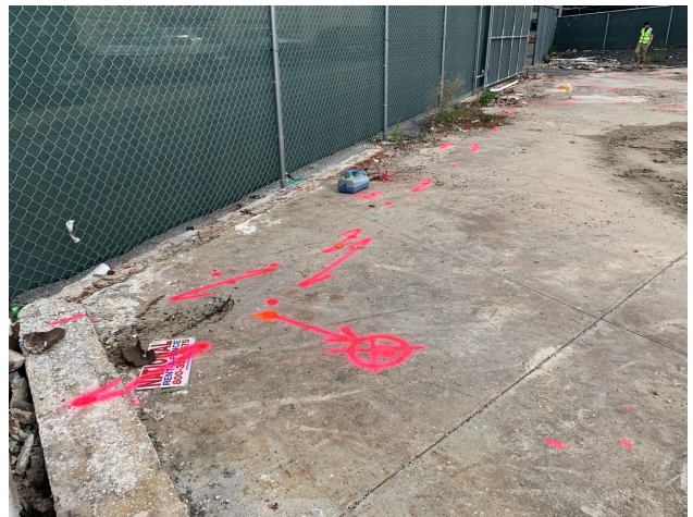
Fig. 1: Images of the areas investigated at 8 Westchester Place, with detected anomalies and utilities in pink paint, and the proposed boring locations marked as circles with an X inside.
