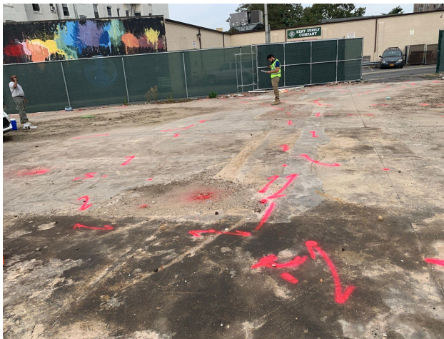
Fig. 1: Images of the areas investigated at 8 Westchester Place, with detected anomalies and utilities in pink paint, and the proposed boring locations marked as circles with an X inside.
