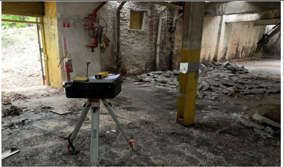
Photo 2 – CAMP station adjacent to demolished slab
