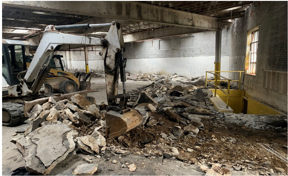
Photo 4 – Demolished slab being moved around by excavator
