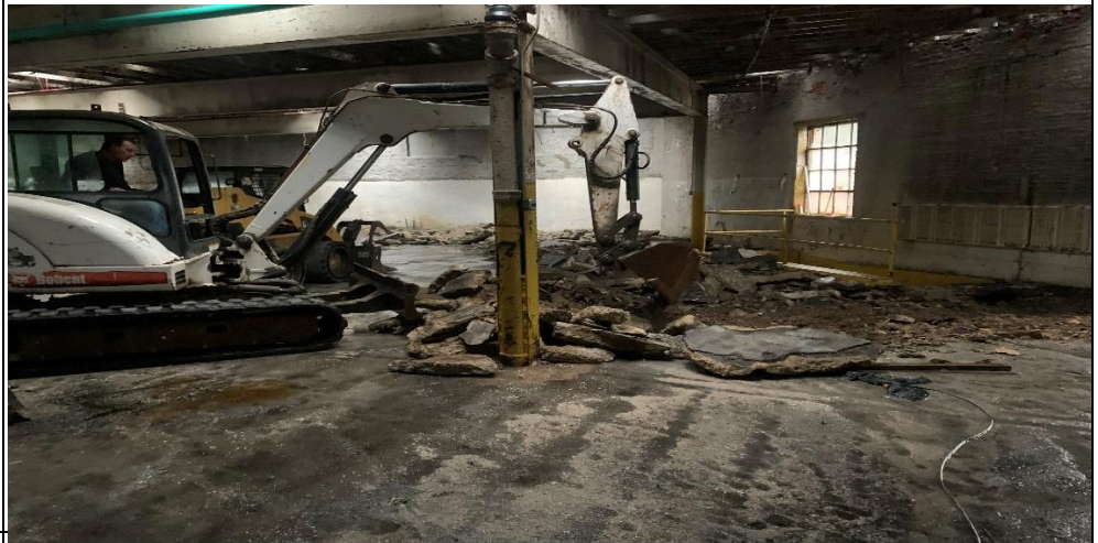
Photo 1 – Start of broken up slab being cleared
