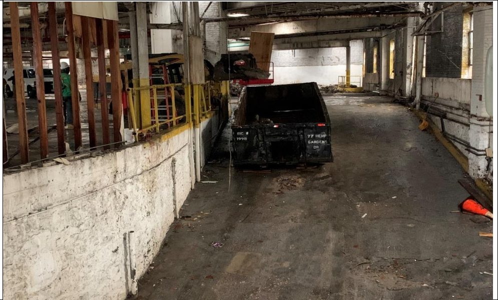
Photo 3 – View of broken up slab being placed into container
