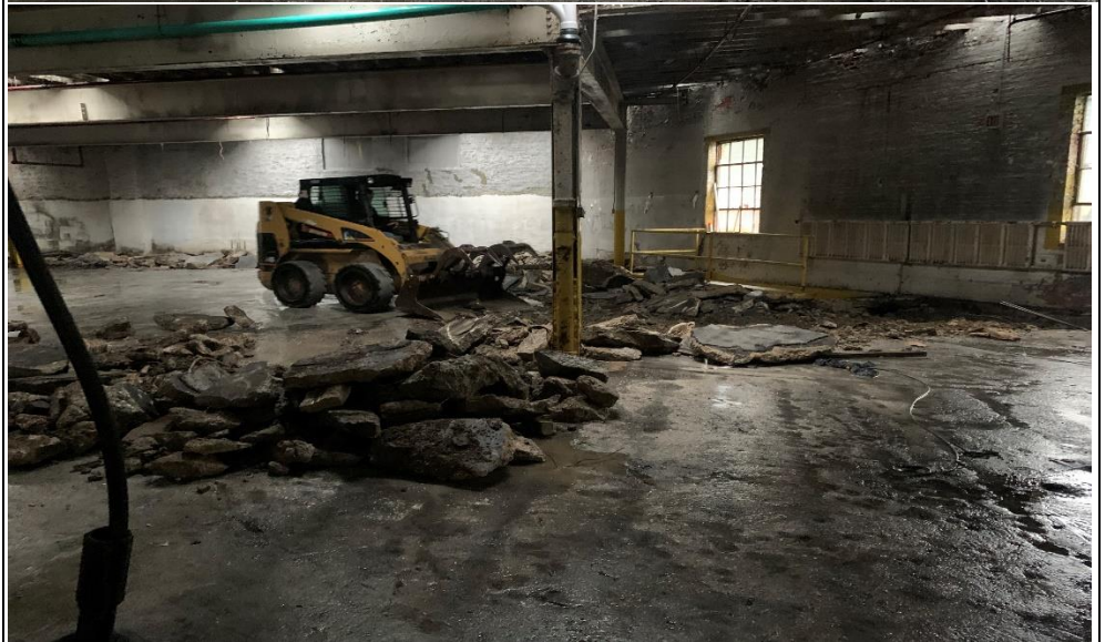
Photo 2 – View of broken up slab piled up
