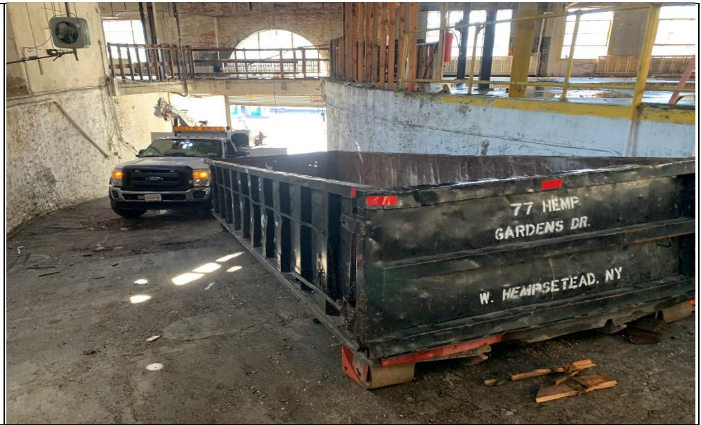
Photo 3 – View of slab/rubble container and repair truck on the ramp
