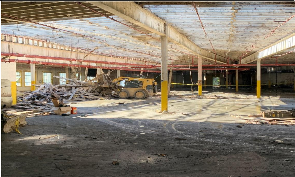
Photo 4 – View of roof, and wood pile after partial removal
