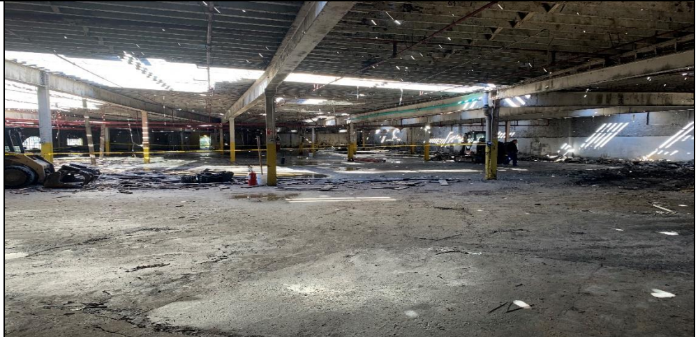
Photo 1 – General view of site facing west
