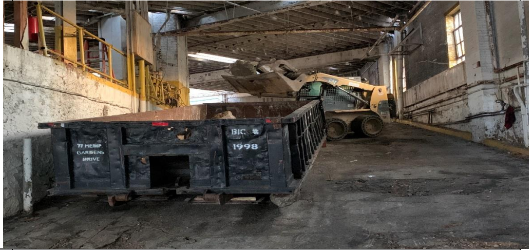
Photo 1 – View of broken slab being placed into container
