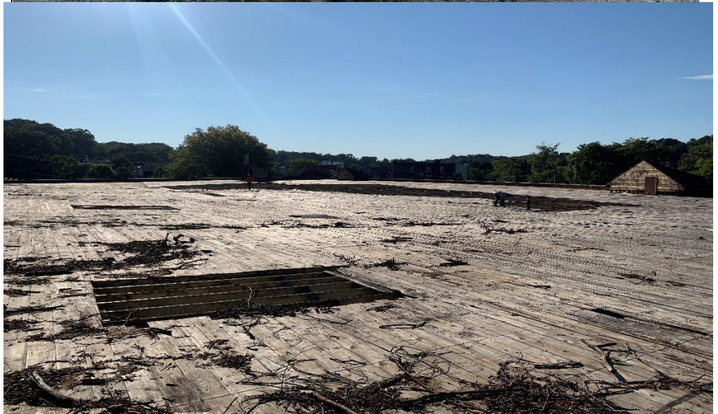
Photo 4 – View of roof with wooden boards being removed
