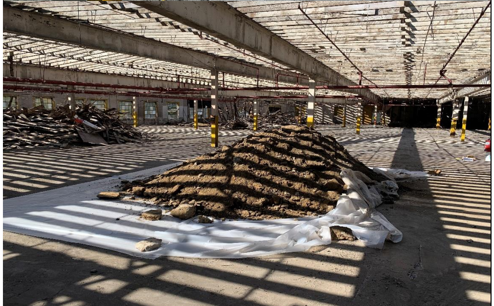
Photo 4 – Soil from piston excavation stockpiled on top of poly sheeting
