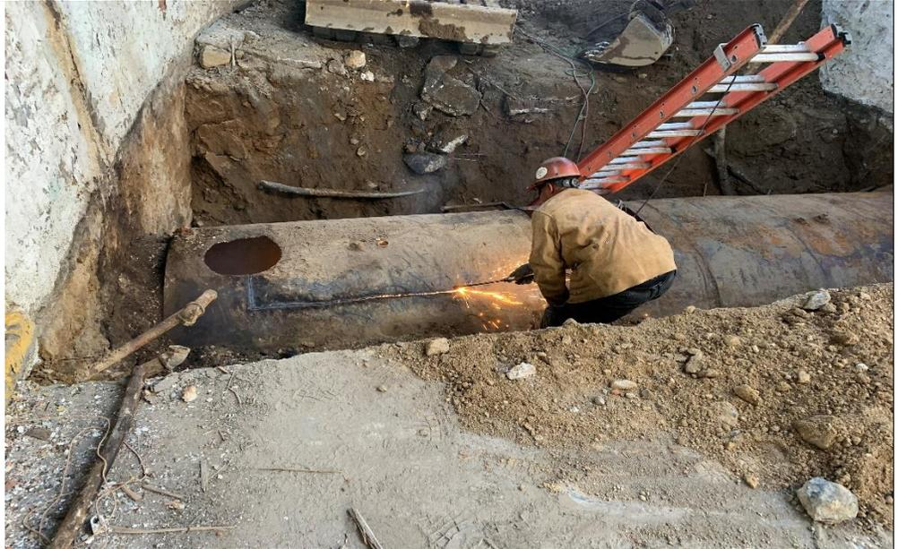
**Photo 2** – View of removal of the UST. Minor staining along eastern wall was evident.
